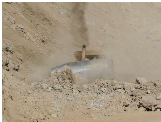
Figure-7: Darreh-Shahr to Abdanan Road (20km from Darreh-Shahr) caused the road block (about 52km to the epicenter.)
