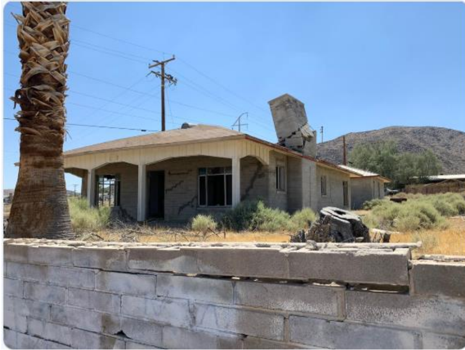
Figure 24. Broken masonry chimney and damaged masonry walls (Source: Ken O'Doll via Twitter)
