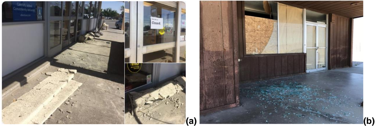
Figure 15. (a) Fallen concrete panels at a building in North Ridgecrest (Source: Karen Hua via Twitter ); (b) Glass facade damage in retail building due to M 6.4 event (Source: AP)
