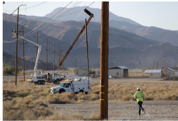
Figure 38. (a) A utility pole in Trona was damaged during the earthquake 32 ; (b) Workers repair damaged utility lines in Trona, CA (AP Photo/Mario Tama | Getty Images 33
