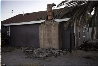
(a) Collapse of a chimney and upper section of a masonry wall
