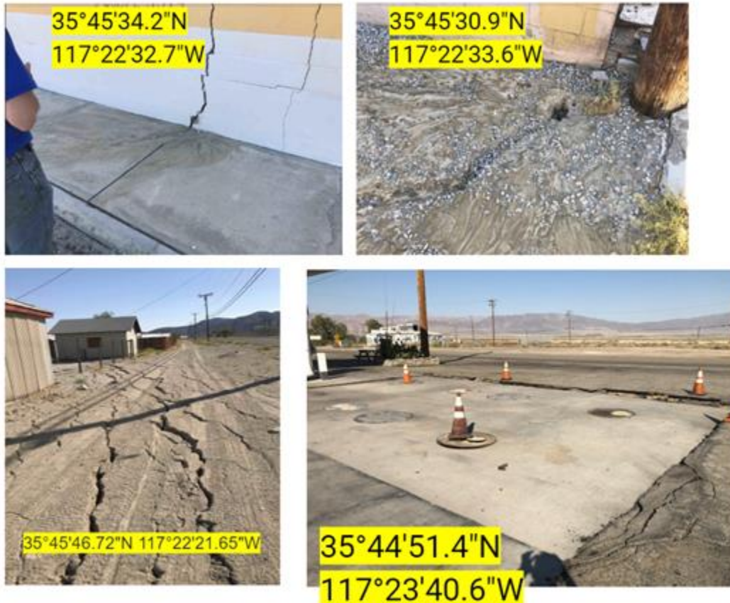
Figure 51. Liquefaction induced lateral spreading and sand boils causing damage to the roadway, and infrastructure in the Trona area (source for all: courtesy of Kenneth Hudson, one of EERI field investigation team members) [clockwise from top left: Esparza restaurant commercial building distance from – closest distance to Searles Lake 0.6 mile; US Post Office Building – closest distance to Searles Lake 1.0 mile; corner of California Street and Argus Avenue; Shell gas station – closest distance to Searles Lake 1.0 mile].
