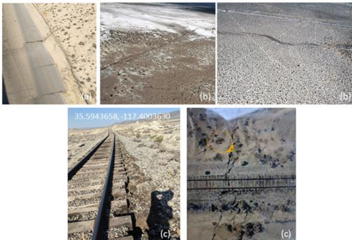
Figure 46. (a) Aerial view of the faulted road on the China Lake NWAS base, about 6.5 feet (1.83 m) right lateral (RL) and 3 feet (0.91 m) vertical offset 51 , (b) North-West trending fault rupture measuring 6 feet (1.83 m) of right-lateral offset on the China Lake NWAS base 52 , and (c) Bent railroad track due to the fault rupture , close to 3 feet (0.91 m) of RL offset 53
