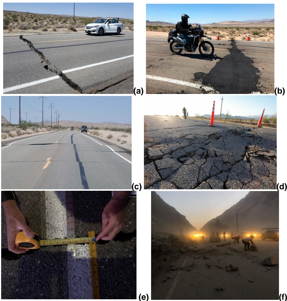
Figure 31. Damage reported in Highway 178 (a) Large crack formed near Trona 20 (b) a motorcyclist rides over a temporarily repaired part of the damaged highway in Ridgecrest one day after the earthquake, demonstrating the rapid response of repair crews; (c) damage reported in Ridgecrest during the M 6.4 event 21 ; (d) surface cracks near Ridgecrest following the M 6.4 event 22 (AP Photo/David McNew) (e) Crack length near Ridgecrest after the July 4th event 23 ; (f) rockslides cause closure of the highway from the M 7.1 event on Friday night; announced clear Saturday at 1 AM by Kern Country 24
