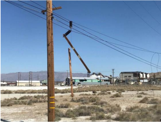
Figure 38. (a) A utility pole in Trona was damaged during the earthquake 32 ; (b) Workers repair damaged utility lines in Trona, CA (AP Photo/Mario Tama | Getty Images 33
