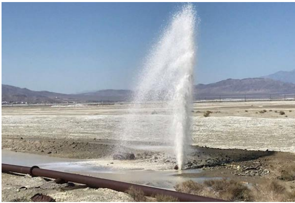
Figure 39. (a) Water spews from pipes in Trona damaged by the M 6.4 event (AP Photo/Matt Hartman 34 ; (b) A crack on Highway 178 seen during fixing a broken water line south of Trona (Source: AP Photo/F.J. BROWN | AFP/GETTY IMAGES 35
