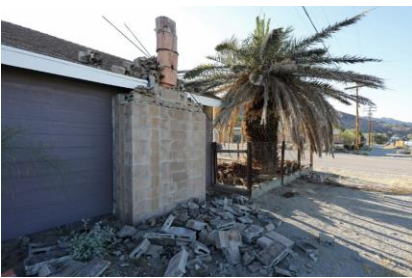
(a) Collapse of a chimney and upper section of a masonry wall
