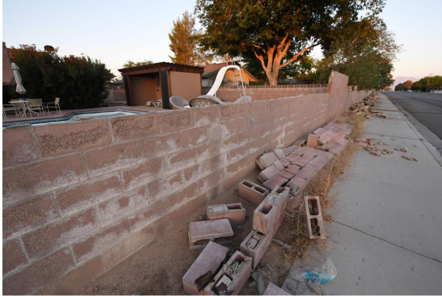
Figure 19. A cinderblock wall partially destroyed in Ridgecrest following the magnitude 7.1 Earthquake (CNN, 2019)
