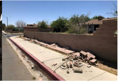
(a) Collapse of a chimney and upper section of a masonry wall
