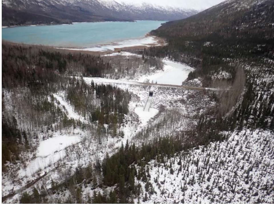
Photo 7. Eklutna Dam where we observed no evidence for ground deformation from aerial reconnaissance. Municipal utilities appeared to perform well during the earthquake. GPS position: 61.420135314°, -149.220729256° (Credit: Rob Witter, USGS)
