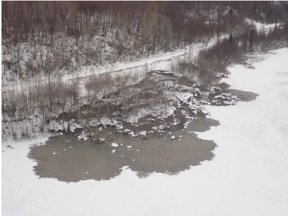
Photo 6. Complex earthflow slumping along Alaska Railroad overlooking tidal flats along Knik Arm near Mirror Lake. Failure of these low bluffs may have involved liquefaction. GPS position 61.437615866°, -149.449646677° (Credit: Rob Witter, USGS)
