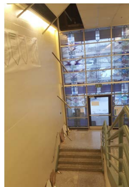
( Twitter ) Chugiak High School - damage to suspended ceilings
