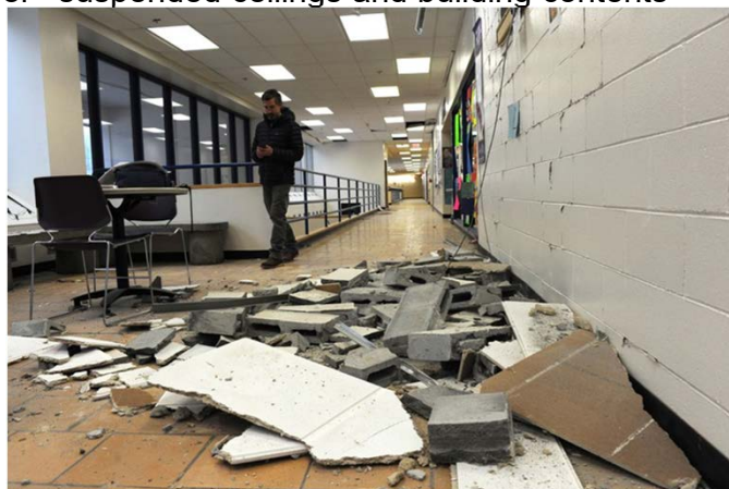
( Anchorage Daily News ) Damage to cinder block wall (non-weight bearing) and ceiling at King Tech High School
