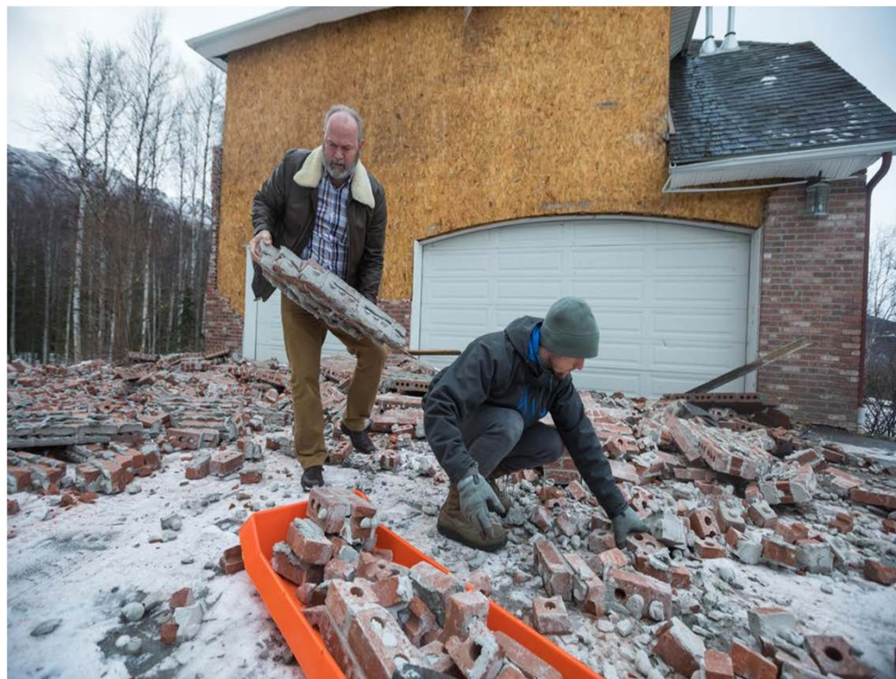
Collapsed Masonry Walls in Eagle River, Alaska
