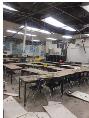
( Twitter ) Chugiak High School - damage to suspended ceilings
