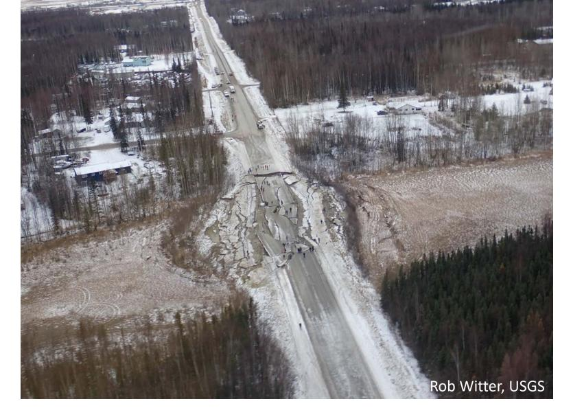
Lateral spreading disrupted Vine Road near Wasilla. Many failures of engineered materials occurred on or adjacent to saturated lowlands filled with organic sediment, silt, or sand.
