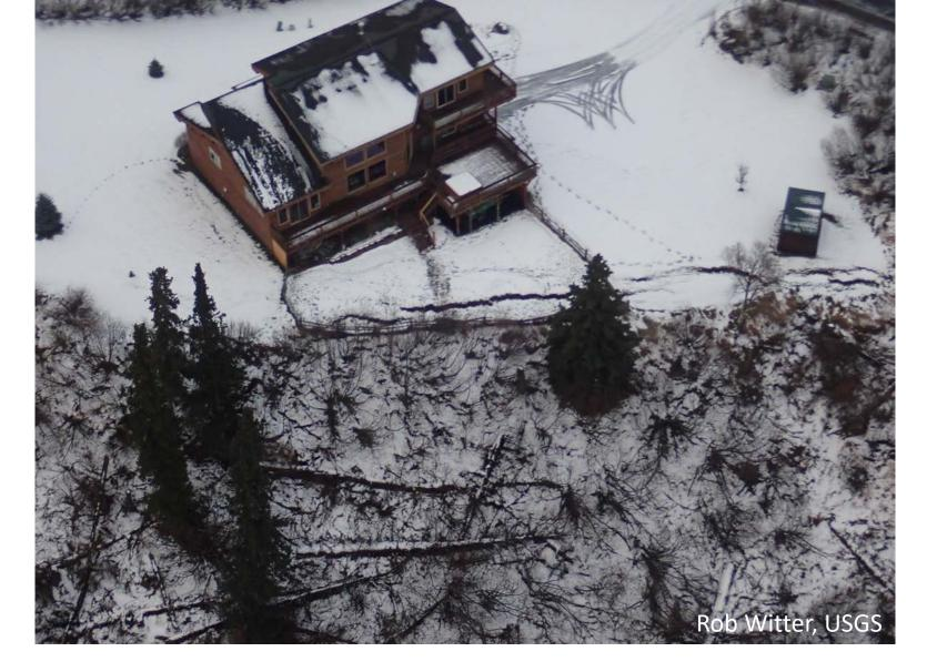
Ground cracks present the potential for future slope failure during aftershocks or heavy rainfall. These cracks occur at the top of a steep valley wall on the south side of Potter Creek in south Anchorage.
