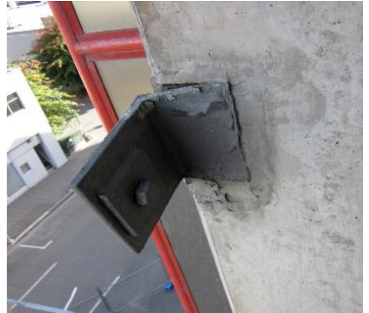
Deformed connections
