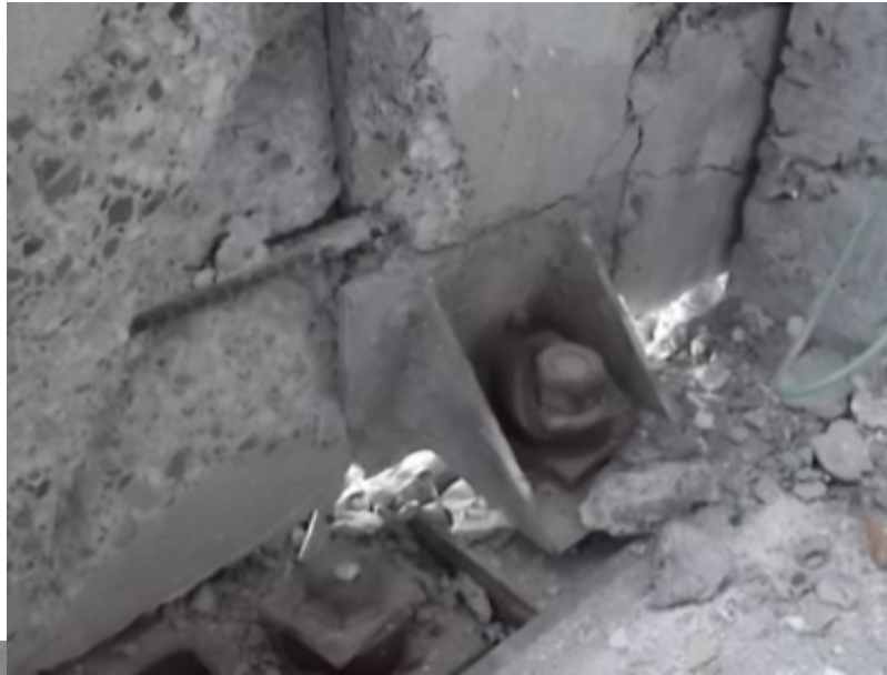
Cracked and spalled concrete
