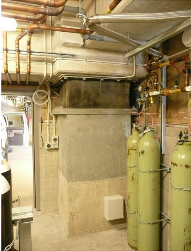
Lead rubber bearing
