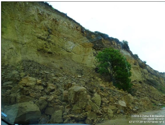
Major rock fall on SH70
