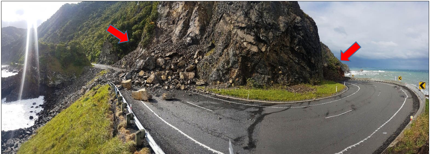
End of the road – Attempts are being made to start removing the rock fall (-42.449696, 173.575200)
