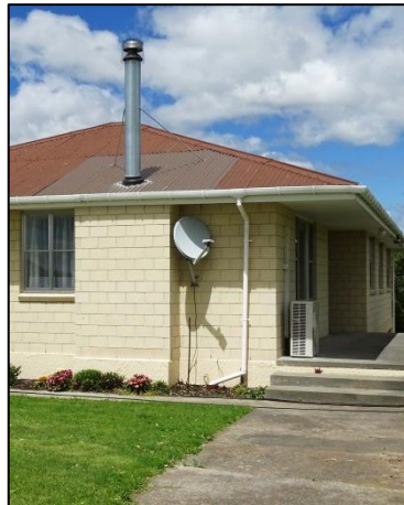
Example of removed chimney, Seddon
