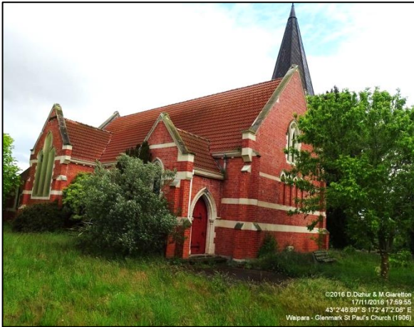
Glenmark St Paul's Church – damaged also following the 2010/2011 Canterbury earthquakes
