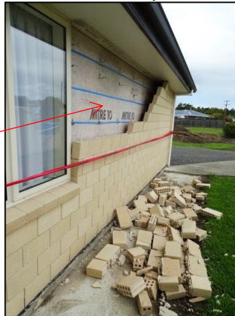
Out-of-plane collapse
