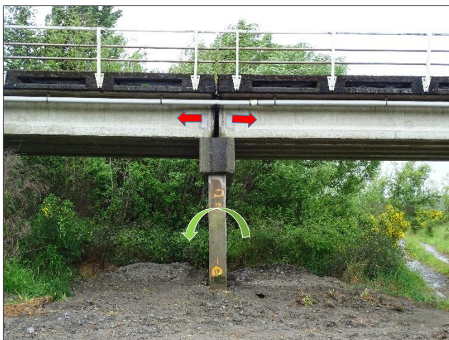
Movement of the Waiau River bridge #1842 deck and potential rotation of the pier (-42.655400, 173.033227)
