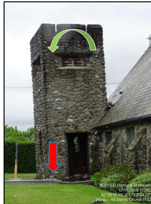
Tilting of the bell tower (note significant settlement of tower foundation)
