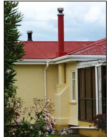
Example of removed chimney, Seddon
