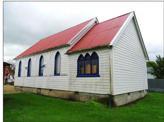
Presbyterian Church – timber framed building with no damage
