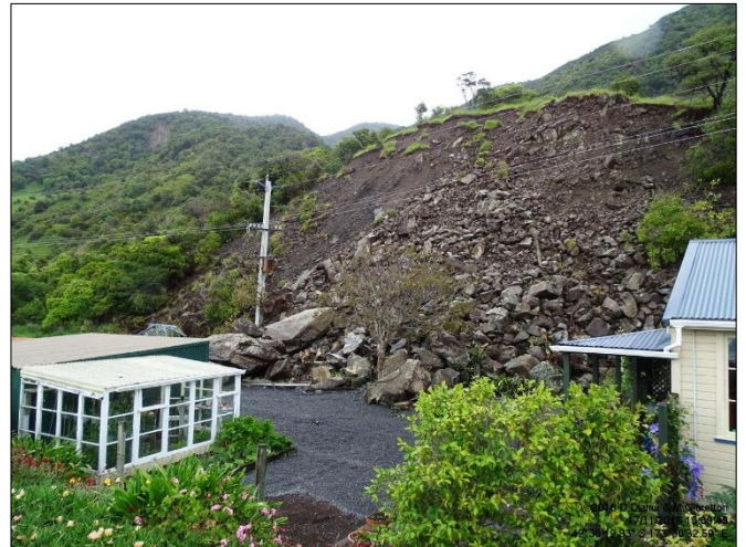
Major rockfall near coast along SH1, near miss of residential dwelling
