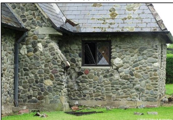
In-plane damage
