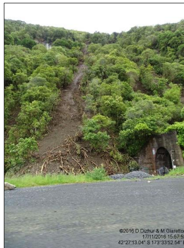
Typical example of soil sliding – blocking railway lines and tunnel entry
