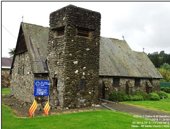
All Saints Church, stone and lightly reinforced concrete
