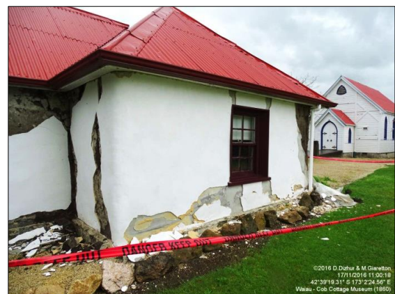
Cob Cottage museum – evidence of textile reinforced mortars used as retrofit
