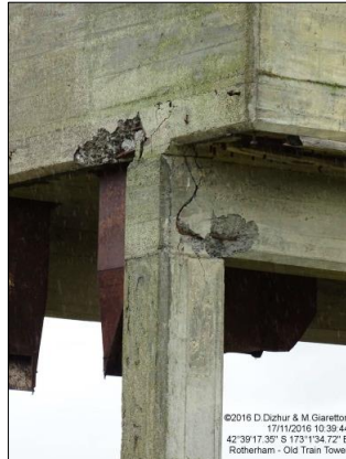
Hinging of the column-to-beam joints
