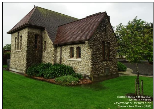
Knox Presbyterian Church – rear view with no observed damage
