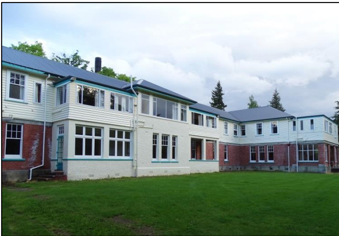
Queen Mary Hospital (1916) – Nurses' Hostel (no damage to loadbearing masonry)
