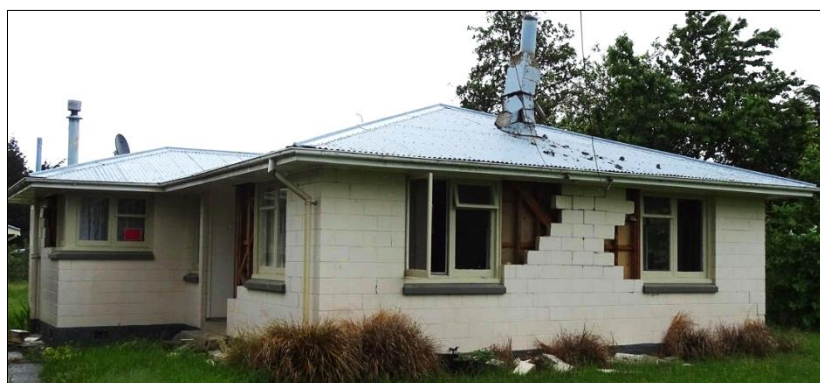
In-plane and out-of-plane damage to veneer, Waiau
