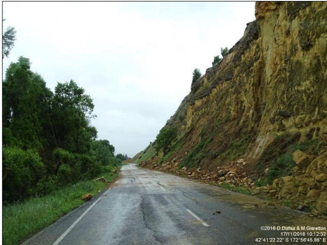
Cleared rock fall on SH70 towards Waiau
