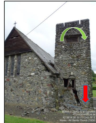
Tilting of the bell tower (note significant settlement of tower foundation)
