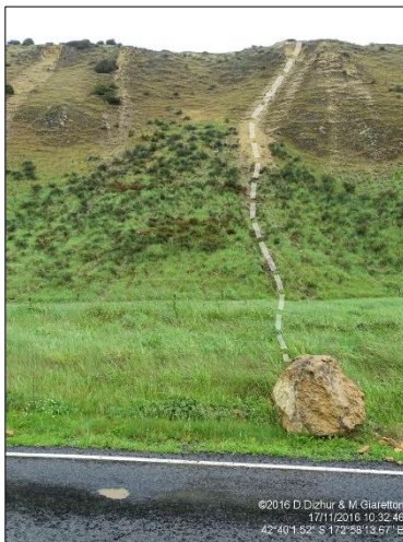
Commonly observed rock rolling path. Multiple examples along SH 70 towards Waiau
