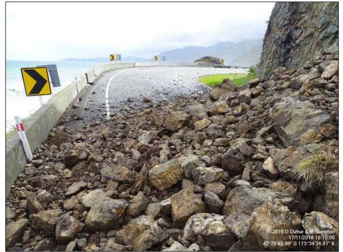
Rockfall over SH1, looking north
