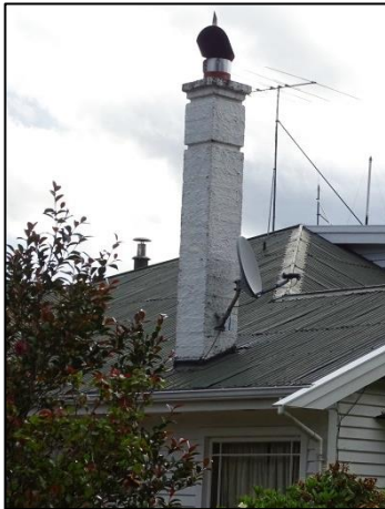
Non-damaged tall chimney, Hanmer Springs
