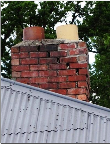
Dislodgment of the bricks, Hanmer Springs
