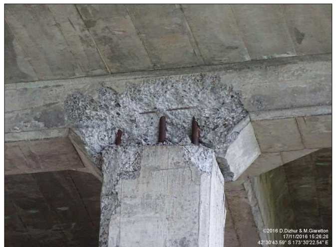
Hinging at the top of column
