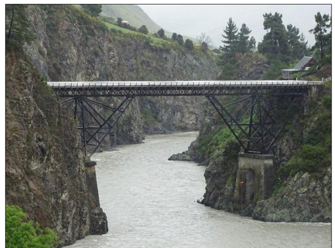
Historic steel bridge originally constructed in 1887. No observed damage, open to all traffic (SH7A leading to Hanmer Springs) (-42.584195, 172.782635)
