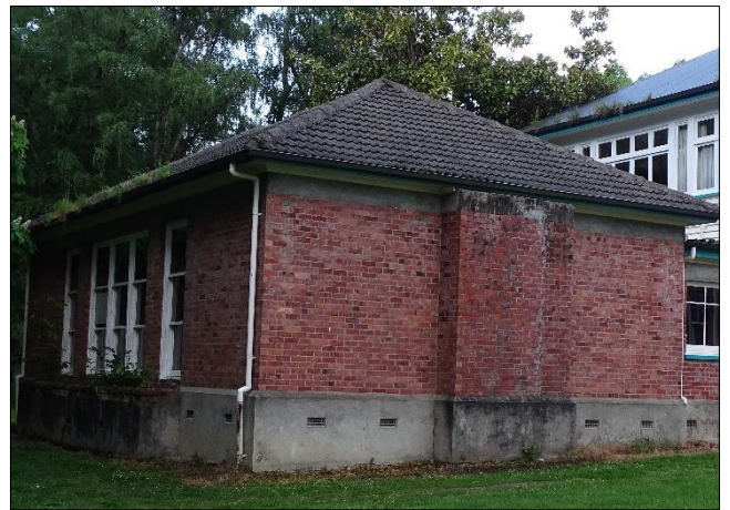
Clay brick cavity masonry building - Queen Mary Hospital (1916) – Chisholm Ward (no damage)
