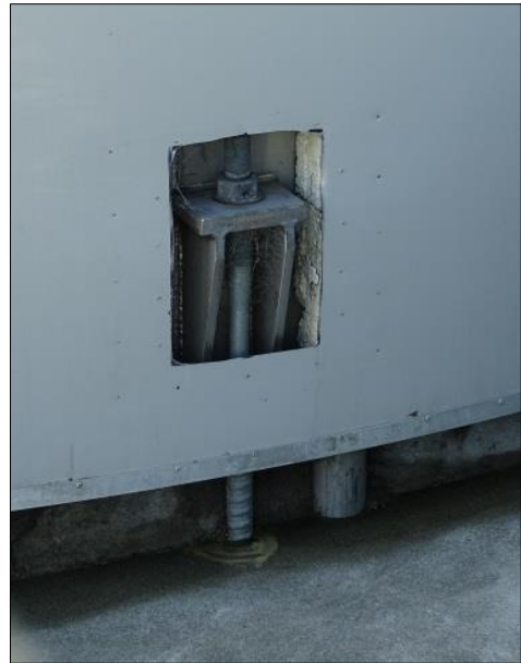
No damage observed for large connections
