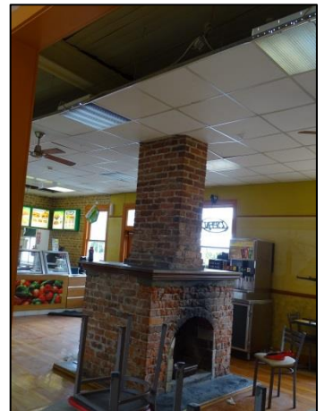
Chimney damage and consequent ceiling damage
