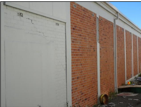
RC with masonry in-fill buildings
