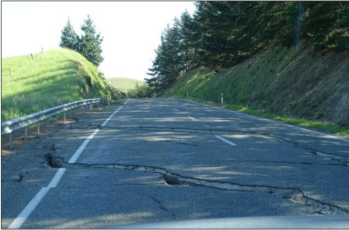
Typical road conditions on approach to Clarence
