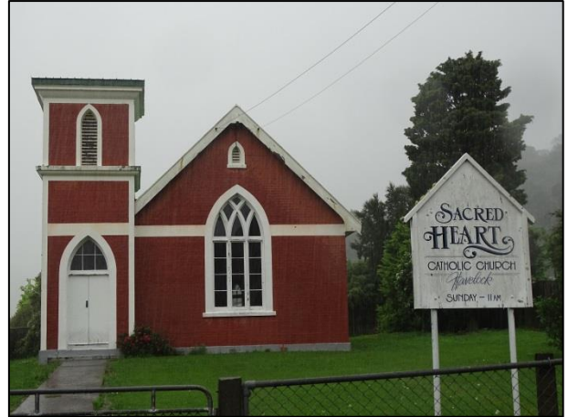
The Sacred Heart Church, clay brick masonry
