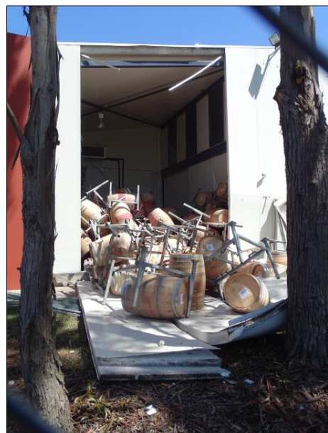
Collapse of stacking systems - wooded barrels' storage
