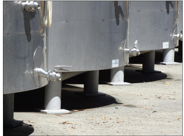
Free standing tanks – no evidence of significant movement
