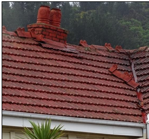
Chimney damage and consequent ceiling damage
