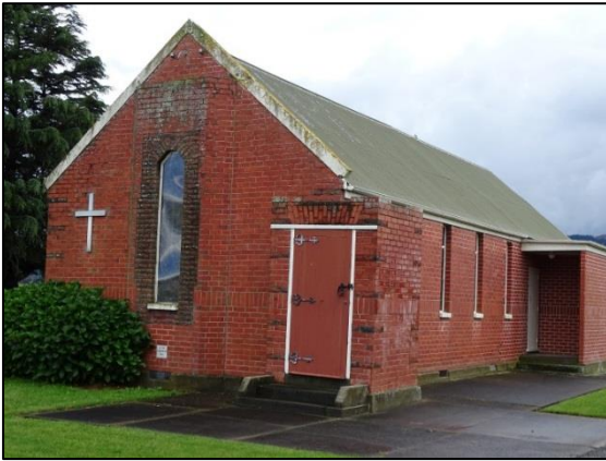
Rapaura Community Church – no visible damage
