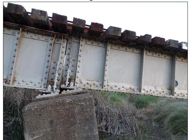
Close up of pier rotation
