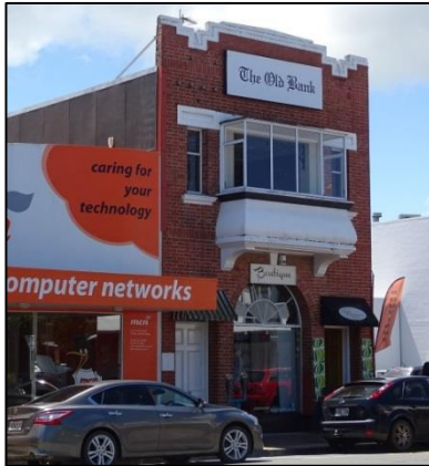
Bank of Australasia, retrofitted clay brick masonry building
