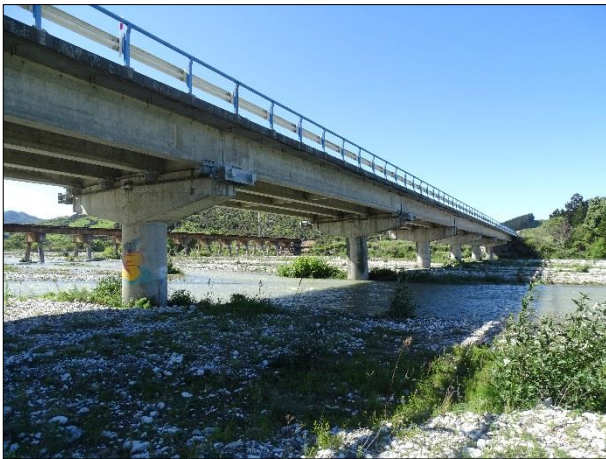
Overall bridge view – accessible to trucks
