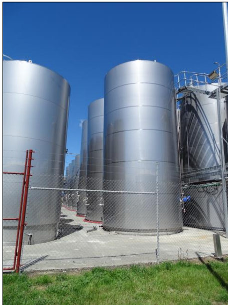
Typical tanks inspected
