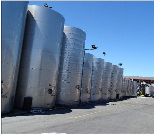
Typical tanks inspected
