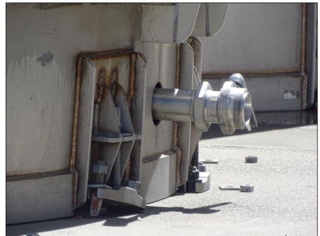
Pull-out of some adhesive anchoring connection
