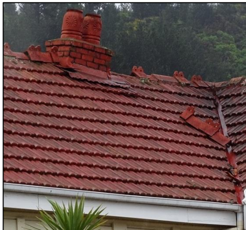
Chimney damage and consequent ceiling damage
