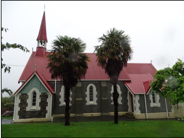
St Peter's Church, stone masonry probably retrofitted
