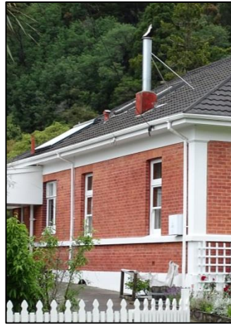
Example of removed chimney, Picton
