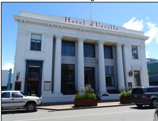
Hotel d'Urville, retrofitted concrete building
