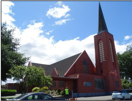
The Church of Nativity, retrofitted clay brick masonry building
