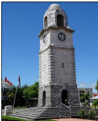
War Memorial and Clock Tower, stone and concrete
