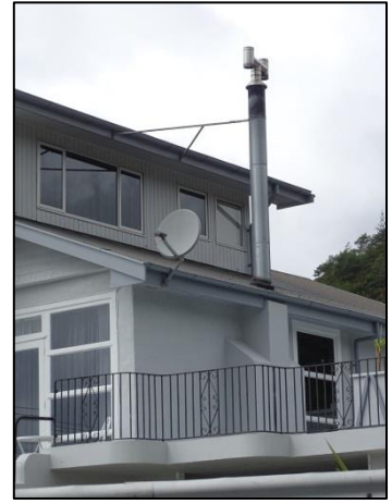
Example of removed chimney, Picton
