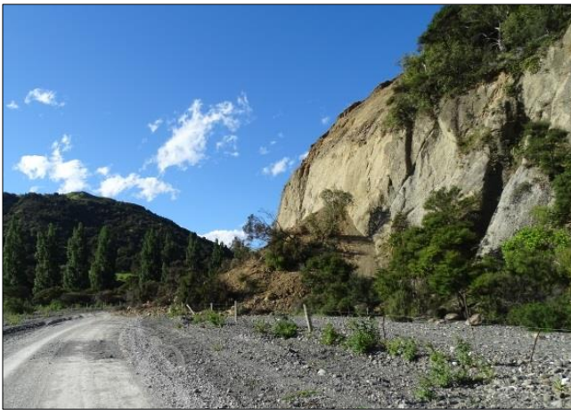
Typical condition of nearby rural roads - 100s land slips
