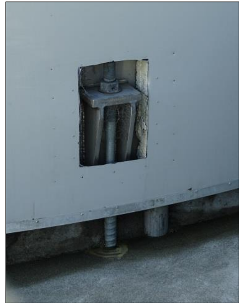
No damage observed for large connections
