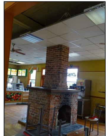
Chimney damage and consequent ceiling damage
