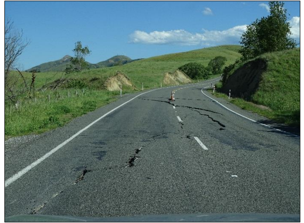
Typical road conditions on approach to Clarence
