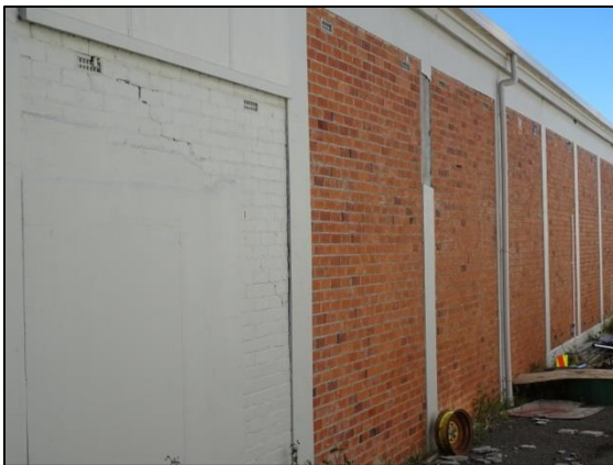
RC with masonry in-fill buildings
