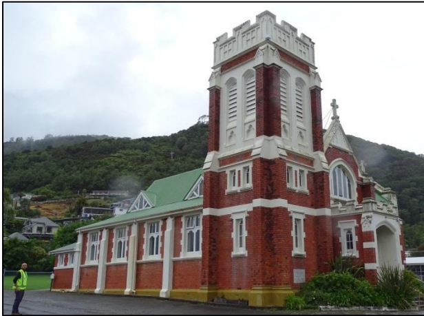
St Joseph's Church, clay brick masonry cavity-wall building (probably retrofitted)
