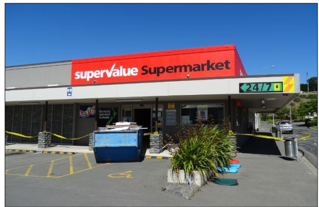
Major non-structural damage to local supermarket, shops and cafes
