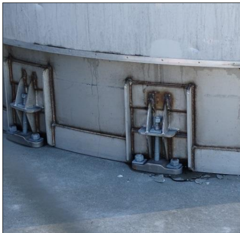
Pull-out of some adhesive anchoring connection
