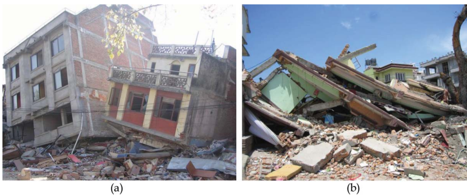
Figure 6. (a) Open ground storey failure of two adjacent buildings in Sitapaila, Kathmandu, and (b) complete collapse of residential building in Khadka Gaon, Kathmandu. To view this figure in colour, please see the online version of the journal.
