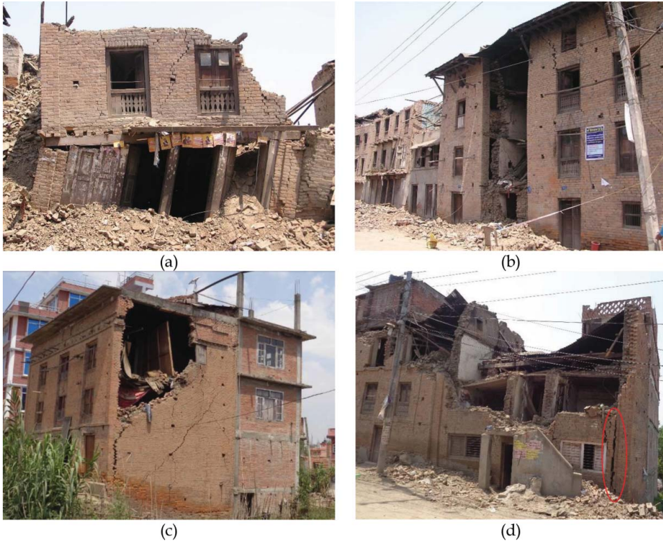
Figure 4. Performance of 50–60-year-old URM buildings at Nikosera in Bhaktapur: (a) collapse of three-storey unreinforced masonry building, (b) out-of-plane failure of the masonry wall, (c) combined in-plane and out-of-plane failure of the wall, and (d) collapse of a building due to poor connection of wall with the floor and cross walls. To view this figure in colour, please see the online version of the journal.
