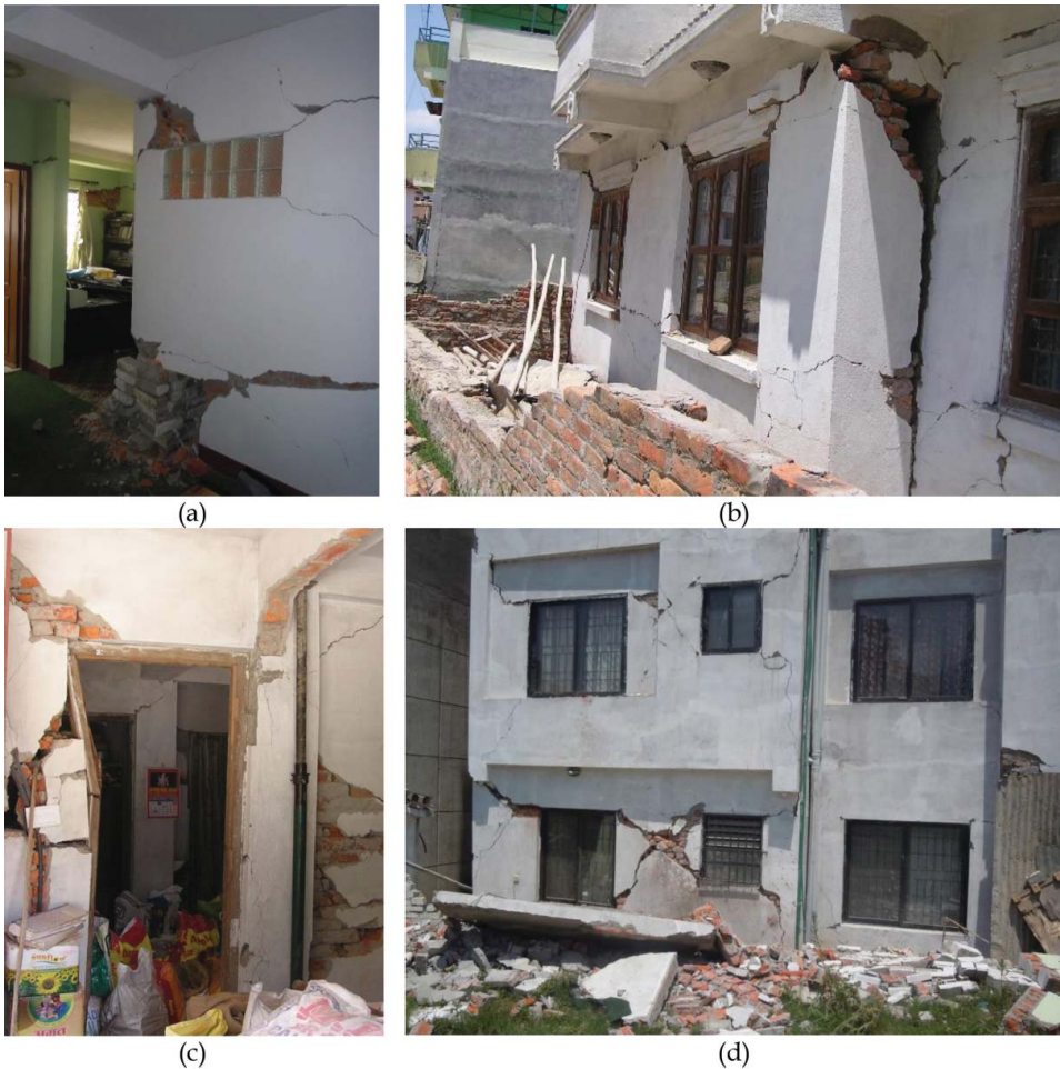
Figure 7. Various structural defects in newly constructed residential buildings: (a) absence of column at the intersection of two walls, (b) projection of masonry wall beyond the column grid line, (c) and (d) damage to the wall panel due to absence of confinement all around the openings. To view this figure in colour, please see the online version of the journal.
