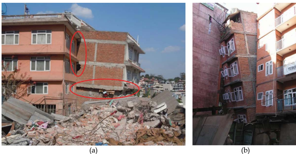
Figure 9. (a) Collapse of intermediate storey due to pounding of adjacent building, and (b) collapse due to extension of the upper storey plan beyond the column grid lines which created vertical irregularity. To view this figure in colour, please see the online version of the journal.
