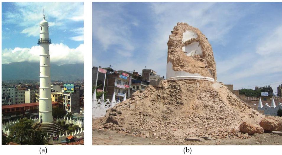
Figure 12. Dharhara tower in Sundhara, Kathmandu: (a) before earthquake (“Creative Commons Dharhara November 10, 2011” by Sugat Shrestha is licensed under CC BY-SA 3.0, link: creativecommons.org/licenses/by-sa/3.0/ ), and (b) after earthquake. To view this figure in colour, please see the online version of the journal.
