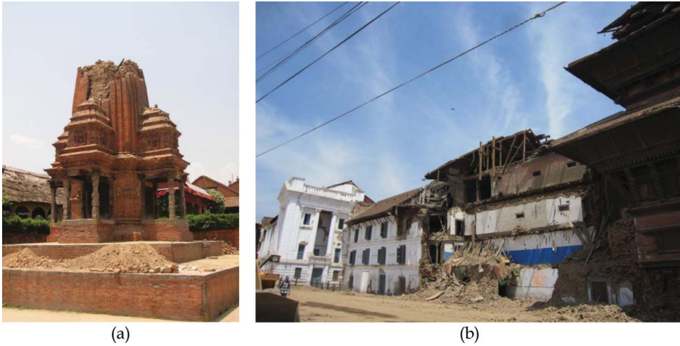
Figure 11. (a) Partial to complete collapse of temples in Bhaktapur Durbar square, and (b) severe damage to unreinforced masonry buildings in the Palace complex of Kathmandu Durbar square. To view this figure in colour, please see the online version of the journal.
