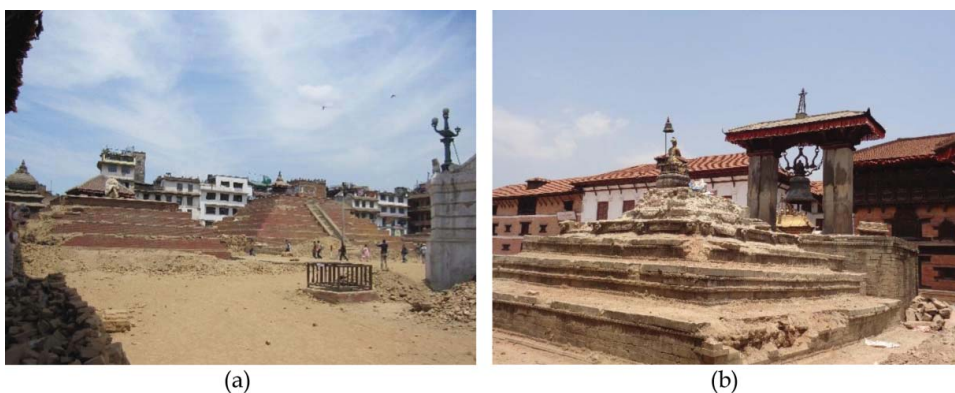
Figure 10. (a) Complete collapse of dega temples in Hanuman Dhoka, Kathmandu, and (b) collapse of Vatsala Durga temple made of sandstone in Bhaktapur Durbar square. To view this figure in colour, please see the online version of the journal.
