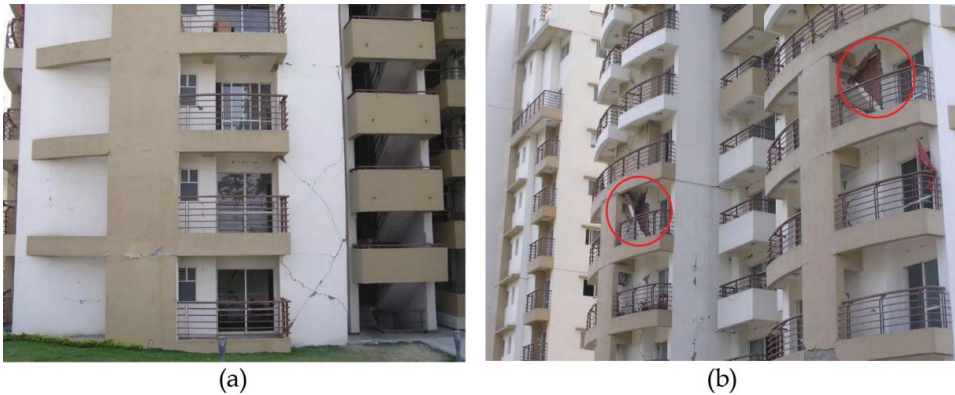
Figure 8. Seventeen-storey apartment building in Patan: (a) shear cracks in the lower storeys of infill wall; (b) combined in-plane and out-of-plane failure of the extended infill wall in upper storeys. To view this figure in colour, please see the online version of the journal.
