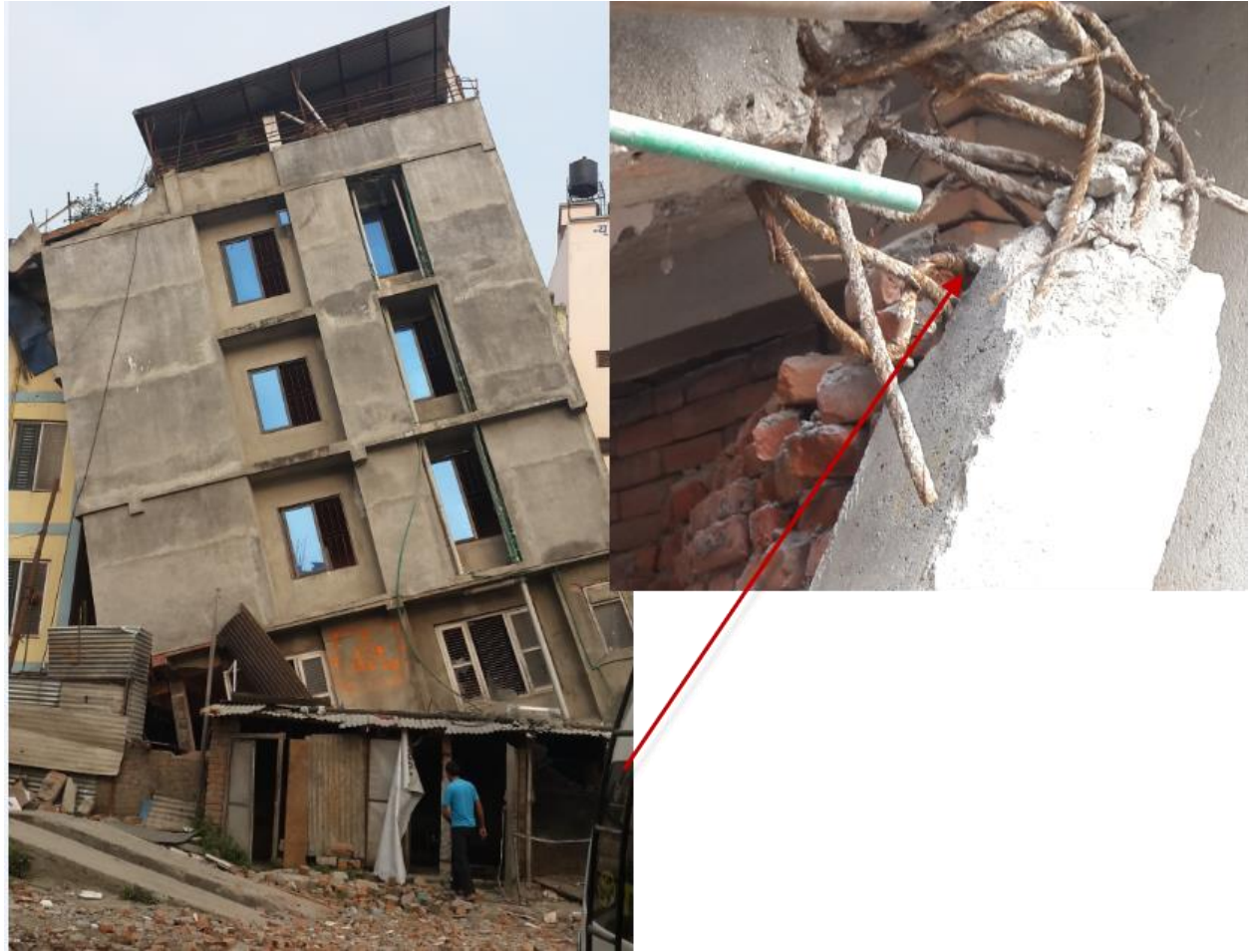
Column shear failure on the ground floor of the house Balaju, Kathmandu ( Photo by Kiran )
