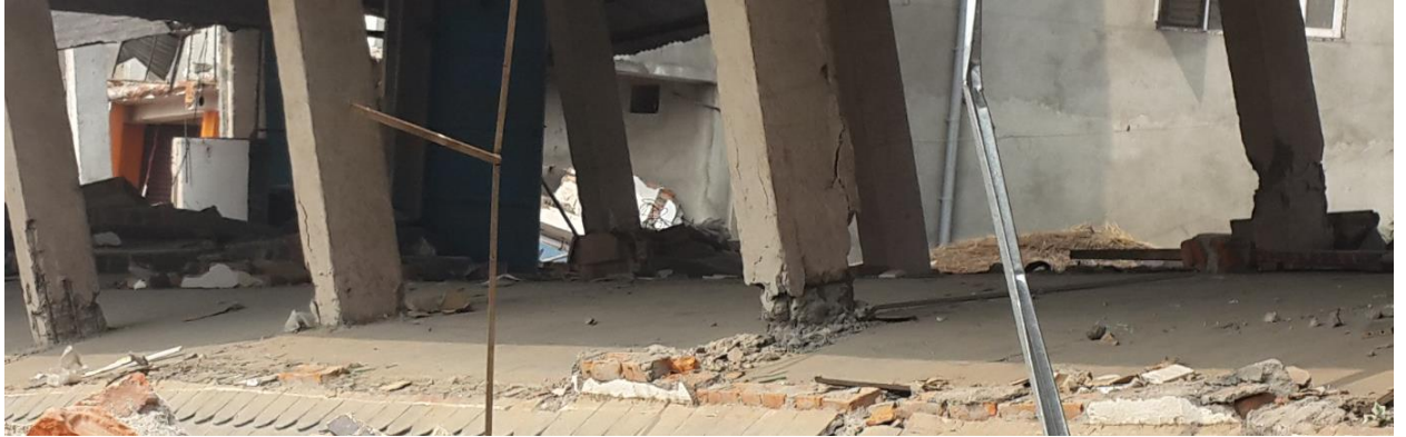
Damaged column bases on upper story of the previous building ( Photo by Kiran )
