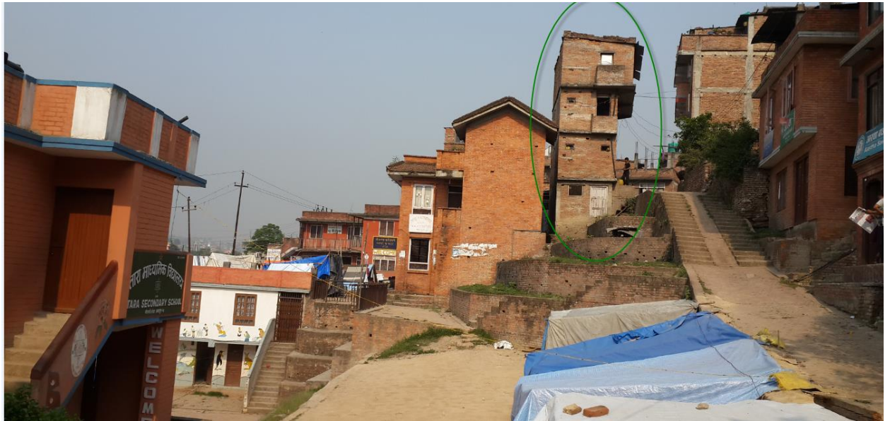
Surprisingly no damage in the marked house, near to the above cracked house. The building on the left corner of the photograph is the retrofitted school building which has no damage at all. (Photo by Kiran)
