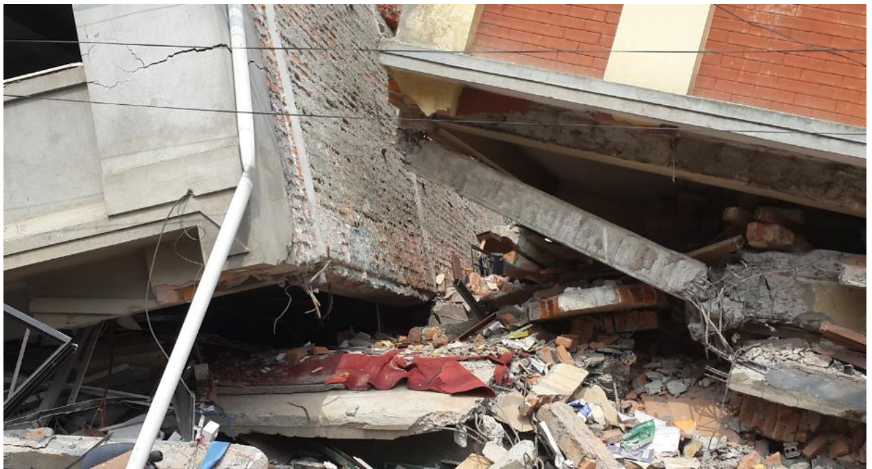
Damaged columns at the marked location of the previous photos ( Photo by Kiran )
