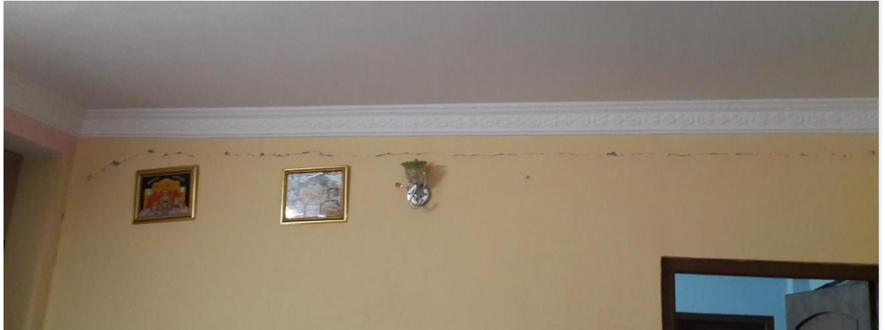
Horizontal crack at the beam interface in a wall that was constructed after constructing the frame in Lalitpur. No other cracks are seen in this 4 story RC frame building except similar vertical cracks at column interface. (Photo by Kiran)
