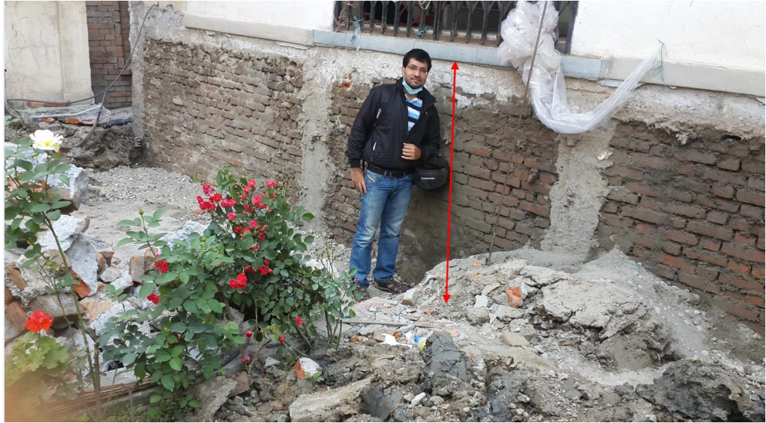
Settlement of the front garden of the white house seen in the previous figure by around 1.5 m (Photo by Kiran)
