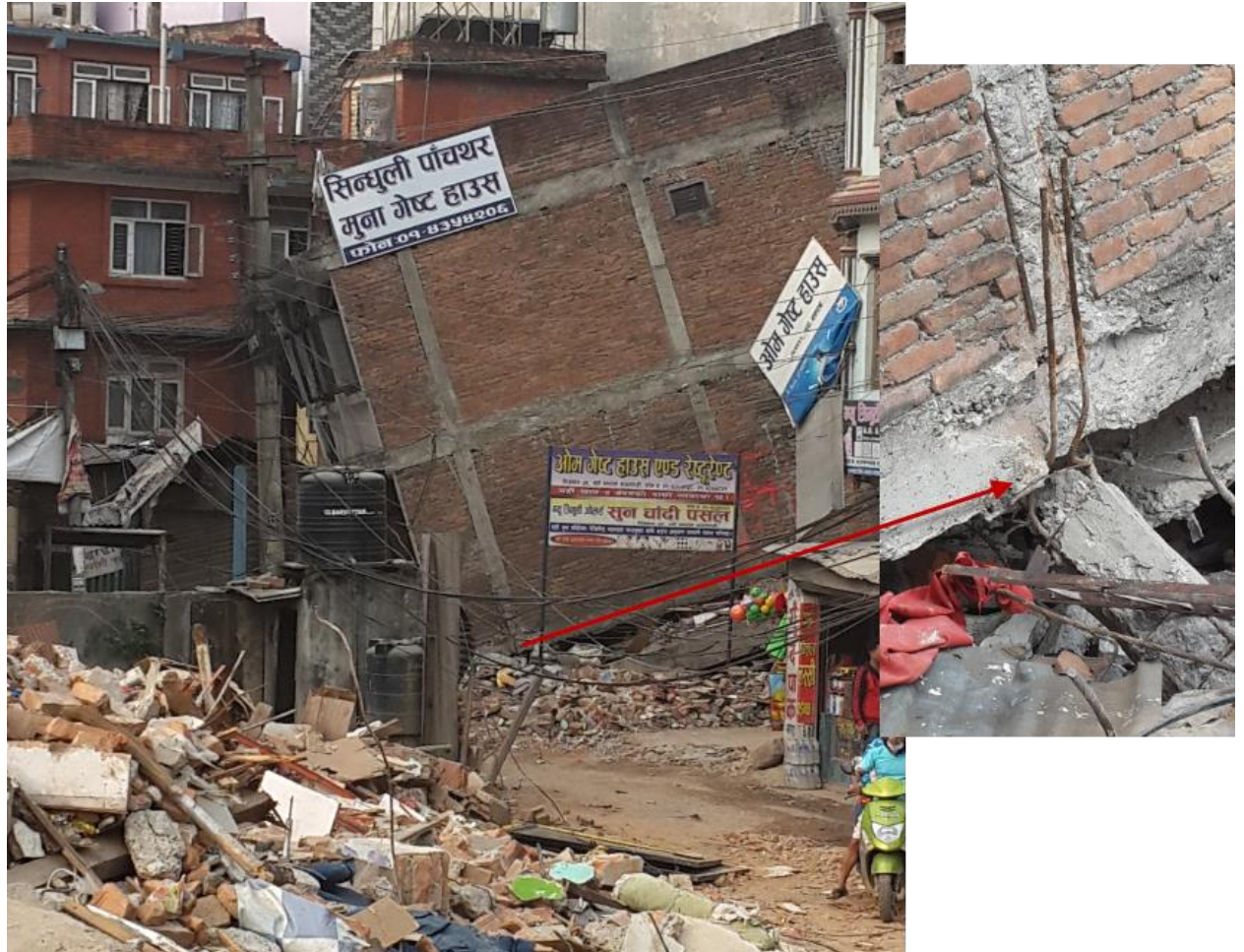
Damaged column of the house in Balaju, Kathmandu area (Photo by Kiran)
