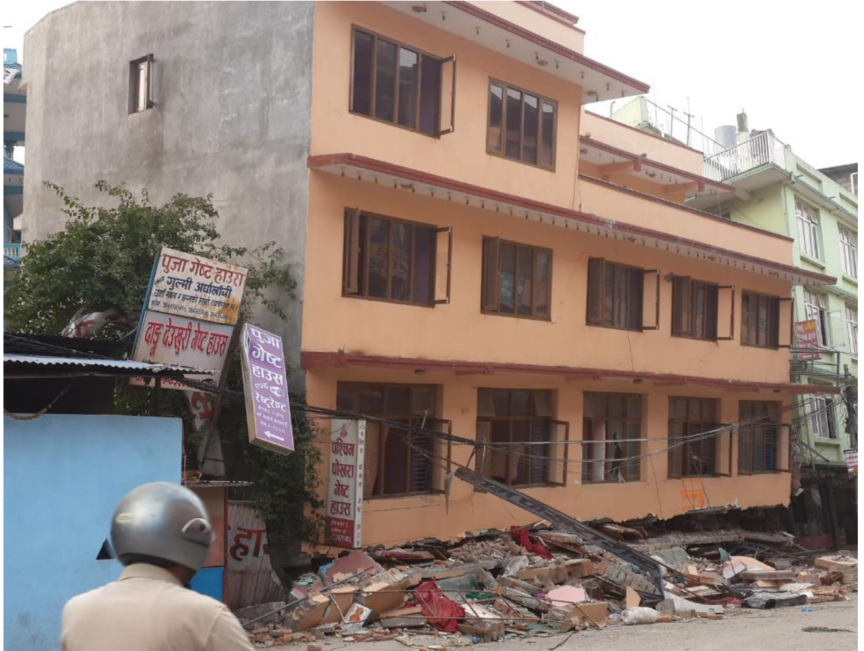
Complete collapse of first two story of a five story house Balaju, Kathmandu, due to soft story effect. There were no infill walls at the periphery of the ground floor. (Photo by Kiran)
