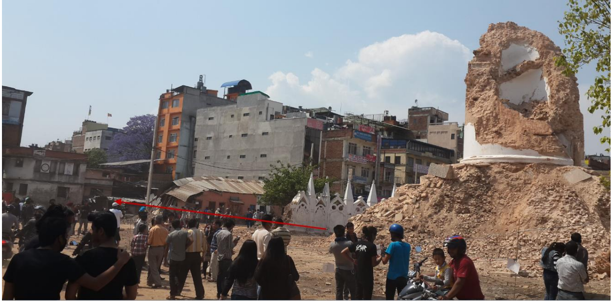
Stump of the 9 storey tall Dharahara tower. It felled down towards the marked direction (Photo by Kiran)
