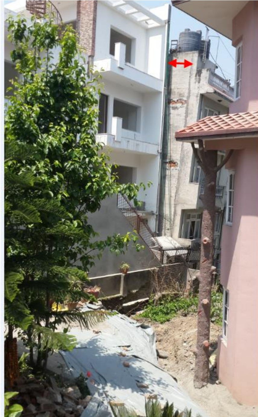
Tilting of the house by around 1 m near the surface cracks (Photo by Kiran Acharya)
