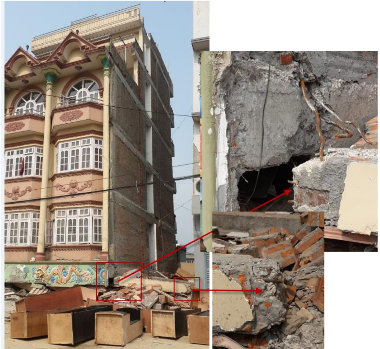
Soft story collapse of another building in Sitapaila, Kathmandu. No stirrups were provided at the beam column joint location. (Photo by Kiran)
