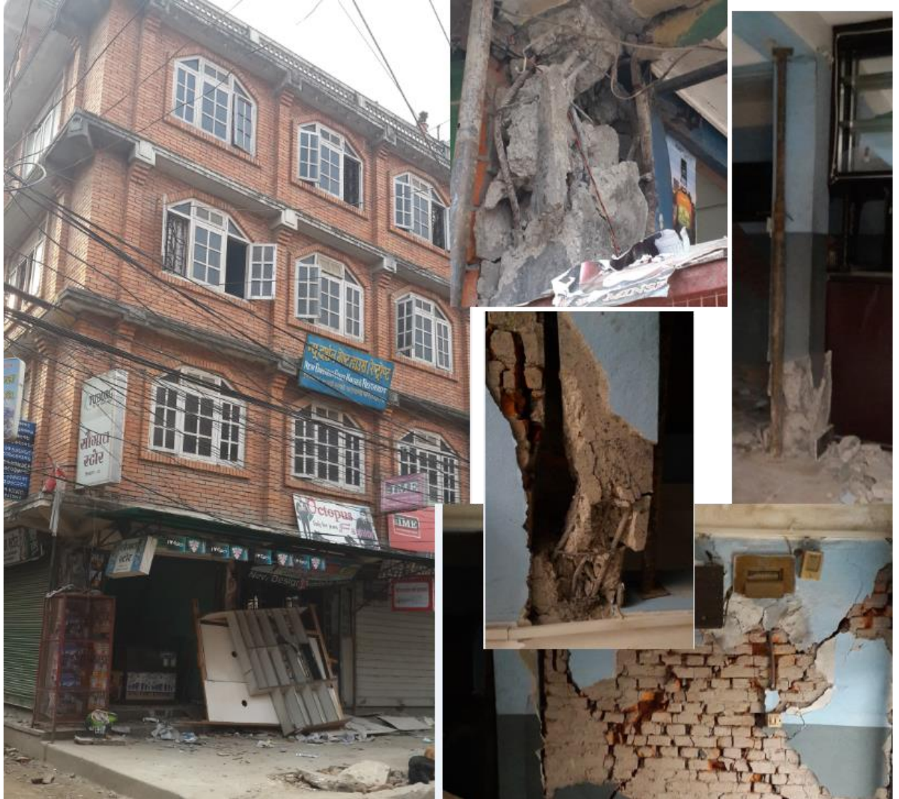
Damages in the interior walls and columns of the house in Balaju, Kathmandu. Longitudinal rebar are buckled after concrete crushing at the soffit of the beam and at column base (Photo by Kiran)
