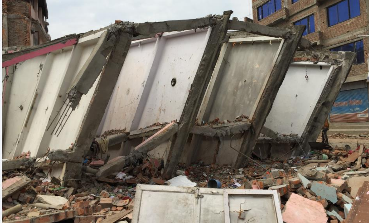
Overturning of a 7 storey tall building in Kapan area, Kathmandu (Photo by Surya Raj Acharya)
