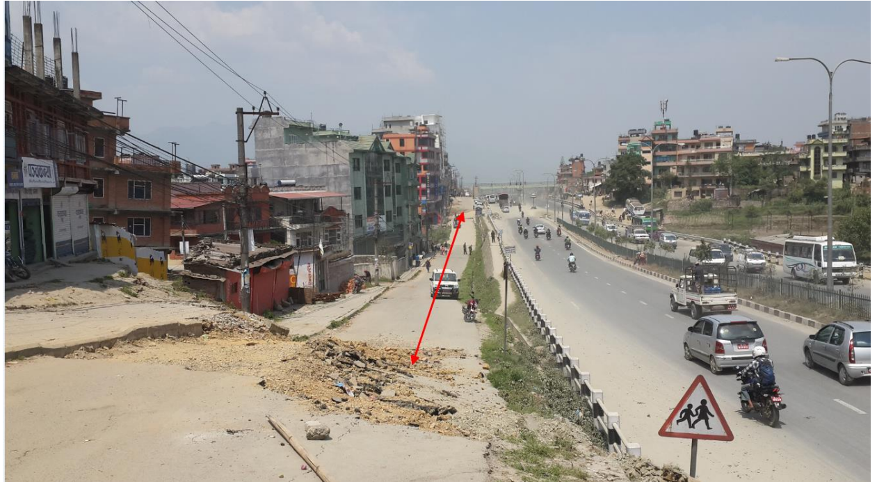
The land along the marked width has been settled by around 1.5 m. No major cracks in the surrounding houses except tilting and shifting of the affected house. (Photo by Kiran Acharya)
