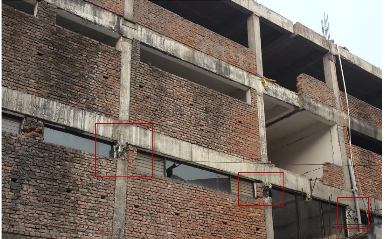
Shear failure of the columns on ground story at the soffit of the beam due to short column effect induced by the infill wall in Balaju, Kathmandu ( Photo by Kiran )
