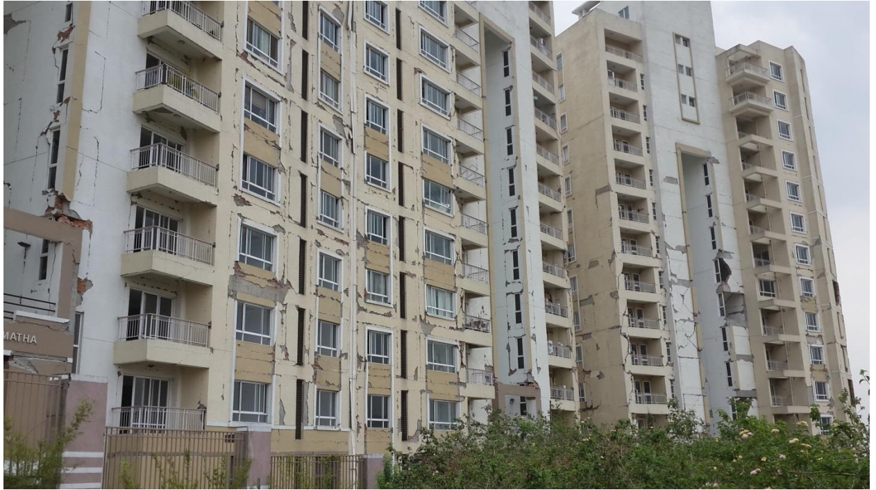
Infill wall damage of a 17 storey tall apartment building in Kathmandu (Right face of the building) (Photo by Kiran)
