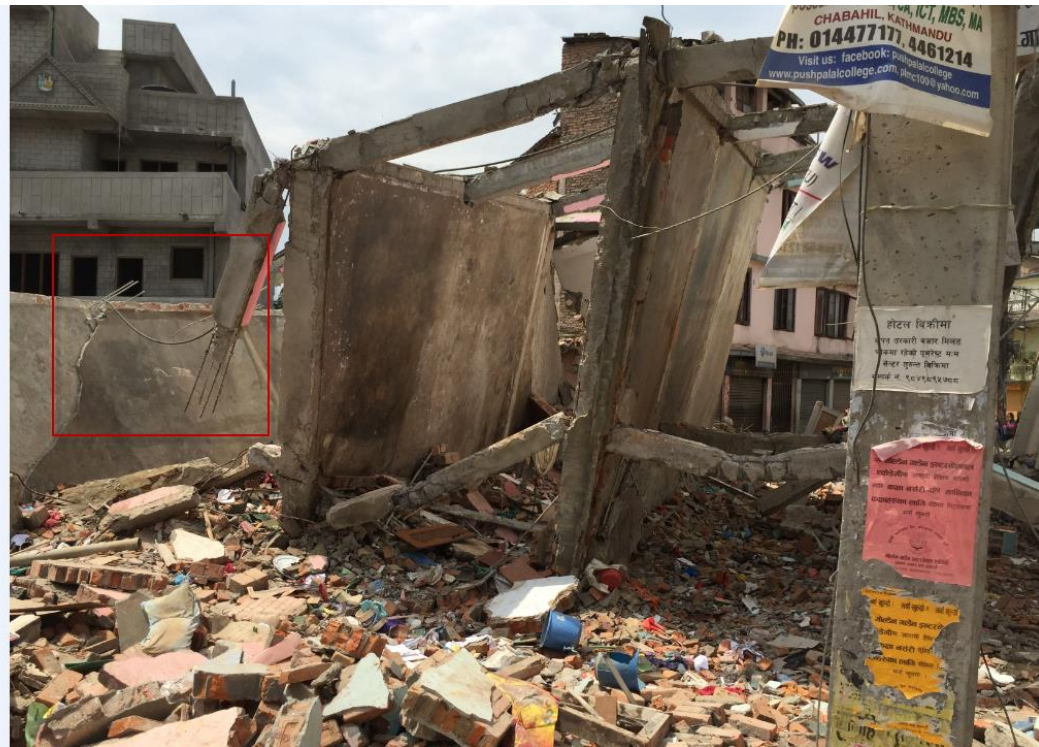
Longitudinal reinforcements were spliced at same location in the column and building overturned by lap splice failure at tension location (Photo by Surya Raj Acharya)
