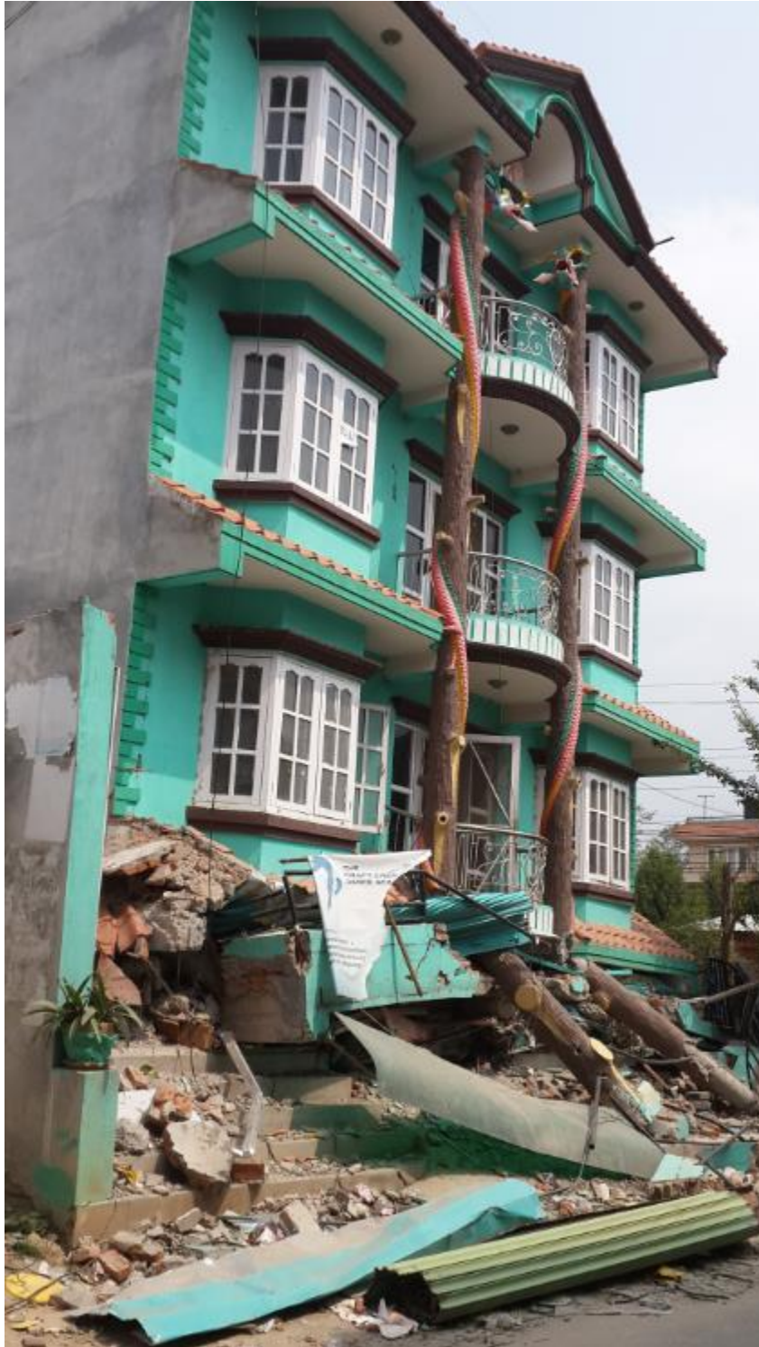
Soft story collapse of a 5 story house in Dhapasi, Kathmandu
