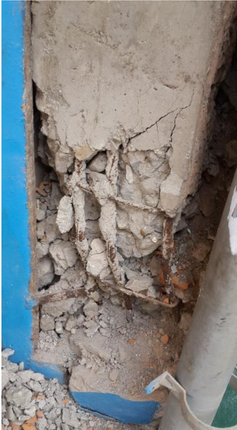
Shear failure of the column at base of other building in Balaju, Kathmandu. (Photo by Kiran)
