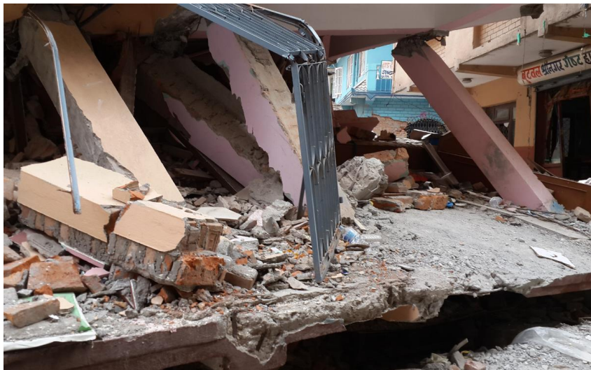
Close up view of the damaged columns of the previous building. (Photo by Kiran)
