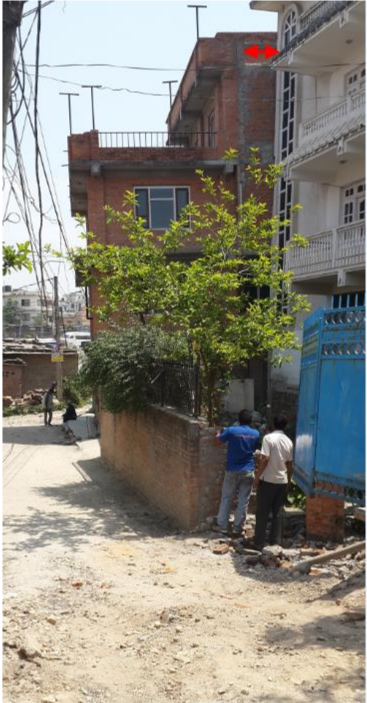
Tilting of the red house. No structural damage in the white house (Photo by Kiran)
