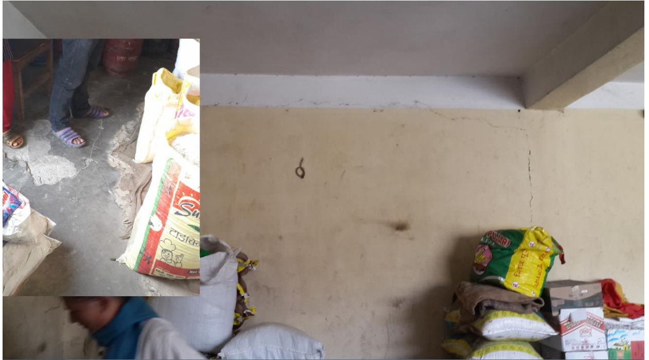
Maximum damages on the walls and floors of the green house seen in the previous figure. (Photo by Kiran Acharya)
