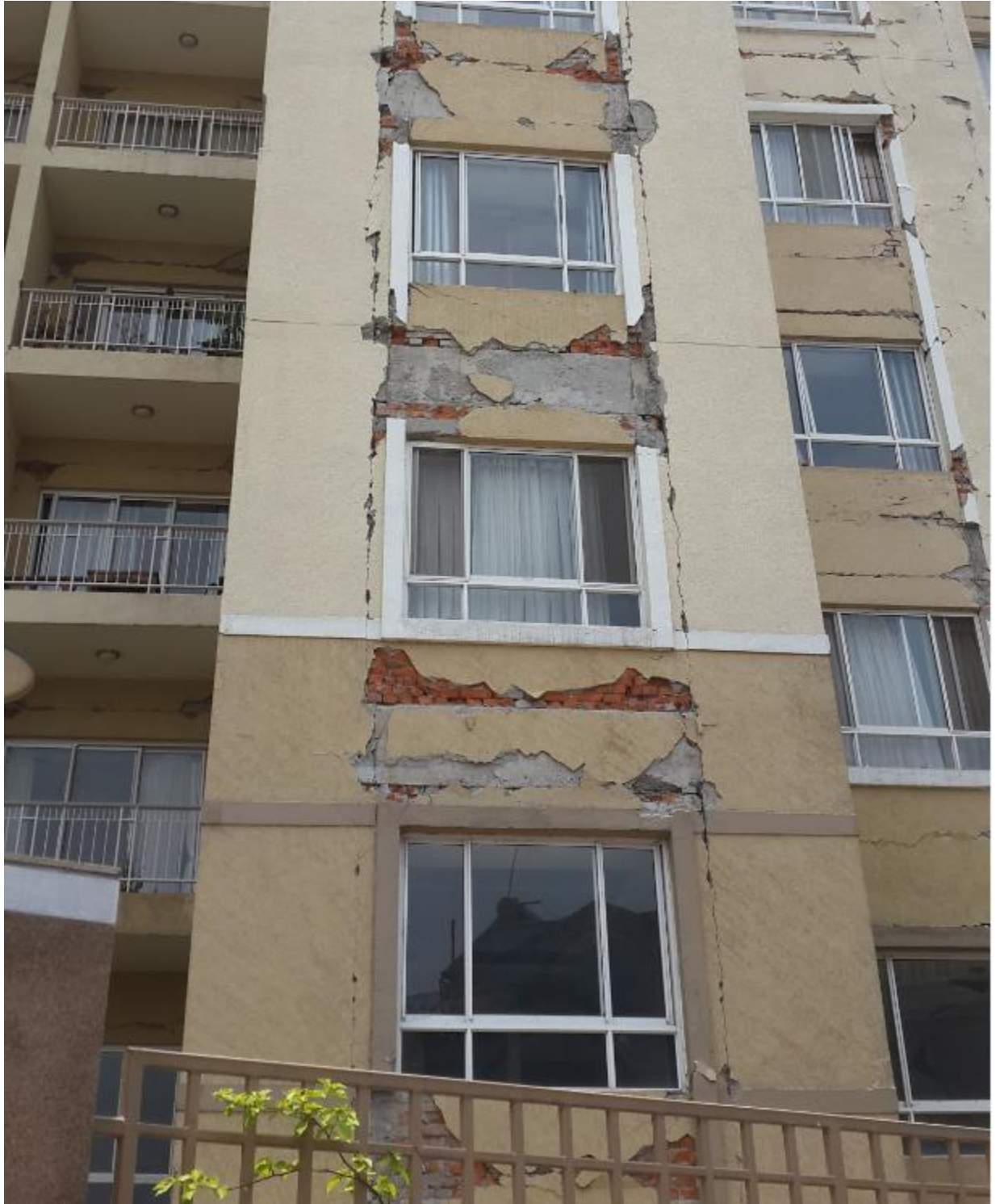
Damage in Spandrel on left face of the (Photo by Kiran)
