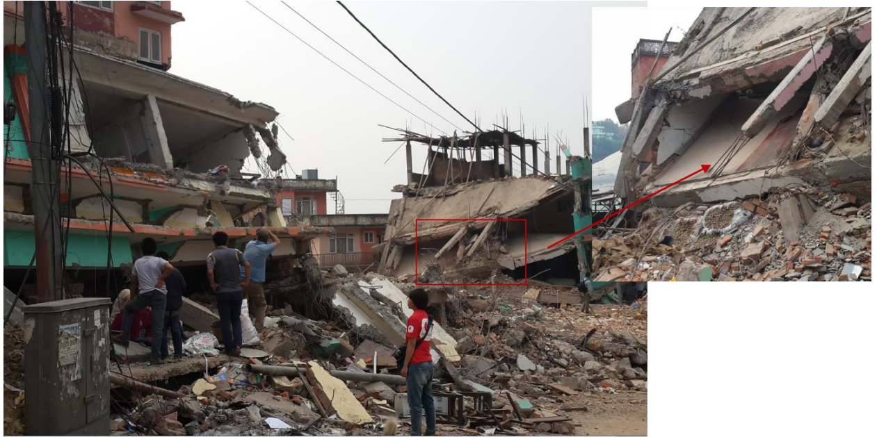
Collapsed building in Sitapaila, Kathmandu. All the rebar were spliced at the same location in the column as marked in the diagram. (Photo by Kiran)
