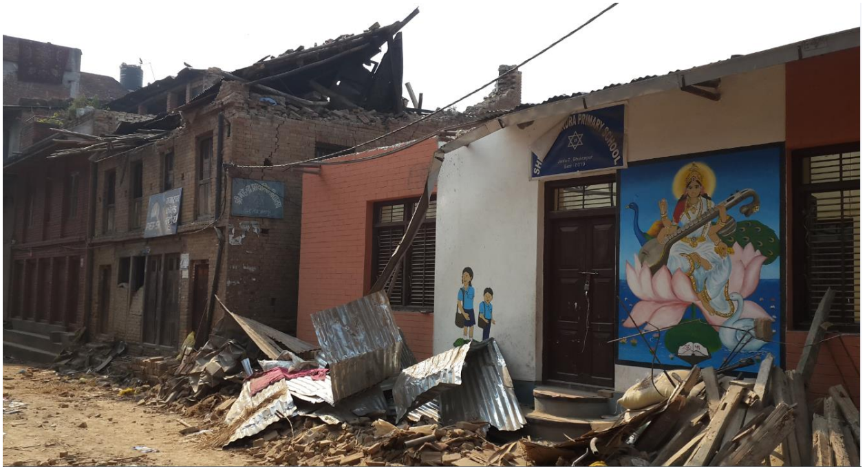
Roof of the retrofitted school building is damaged by the adjacent house (Photo by Kiran)
