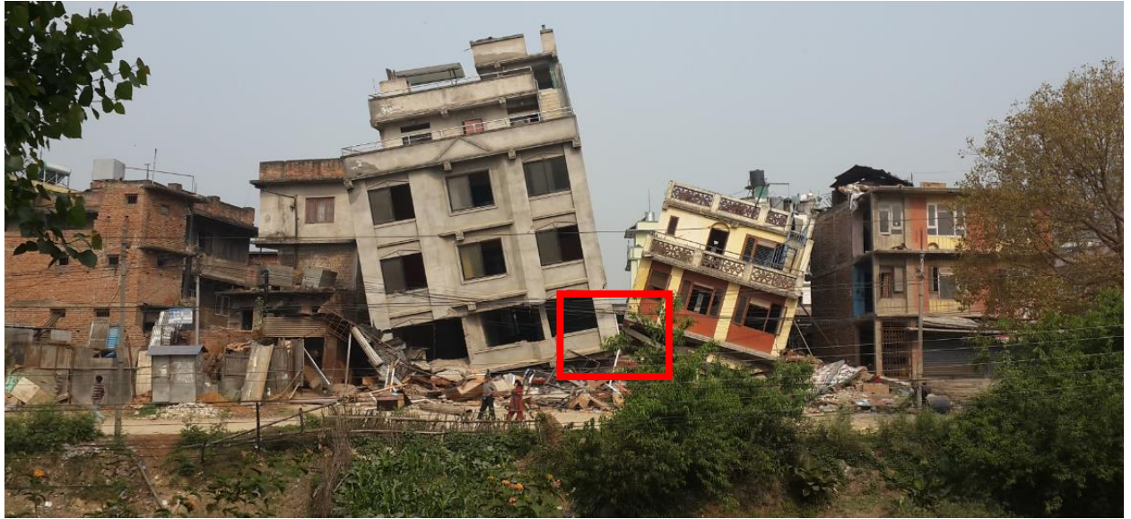
Collapsed buildings due to soft story effect, Sitapaila, Kathmandu ( Photo by Kiran )
