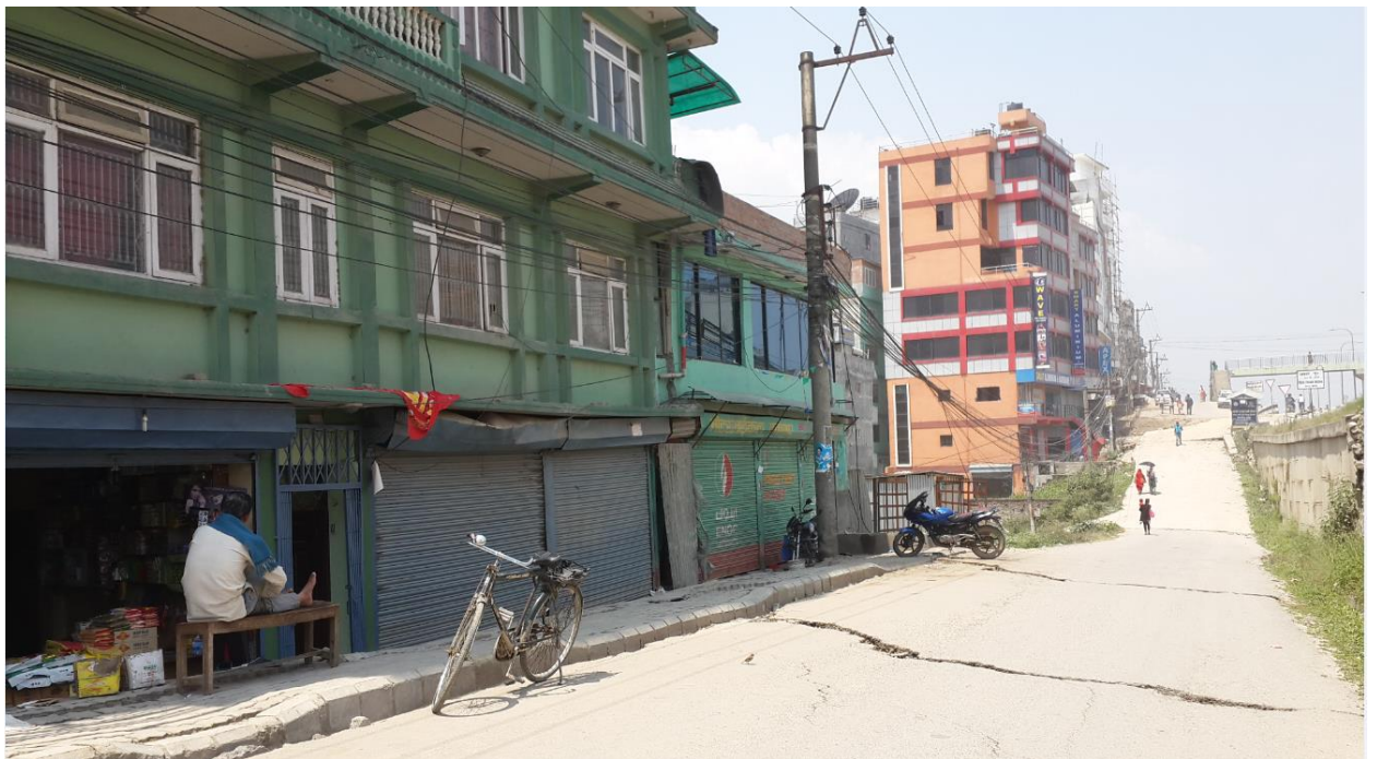
Surface ruptures in the settled part of the land (Photo by Kiran Acharya)
