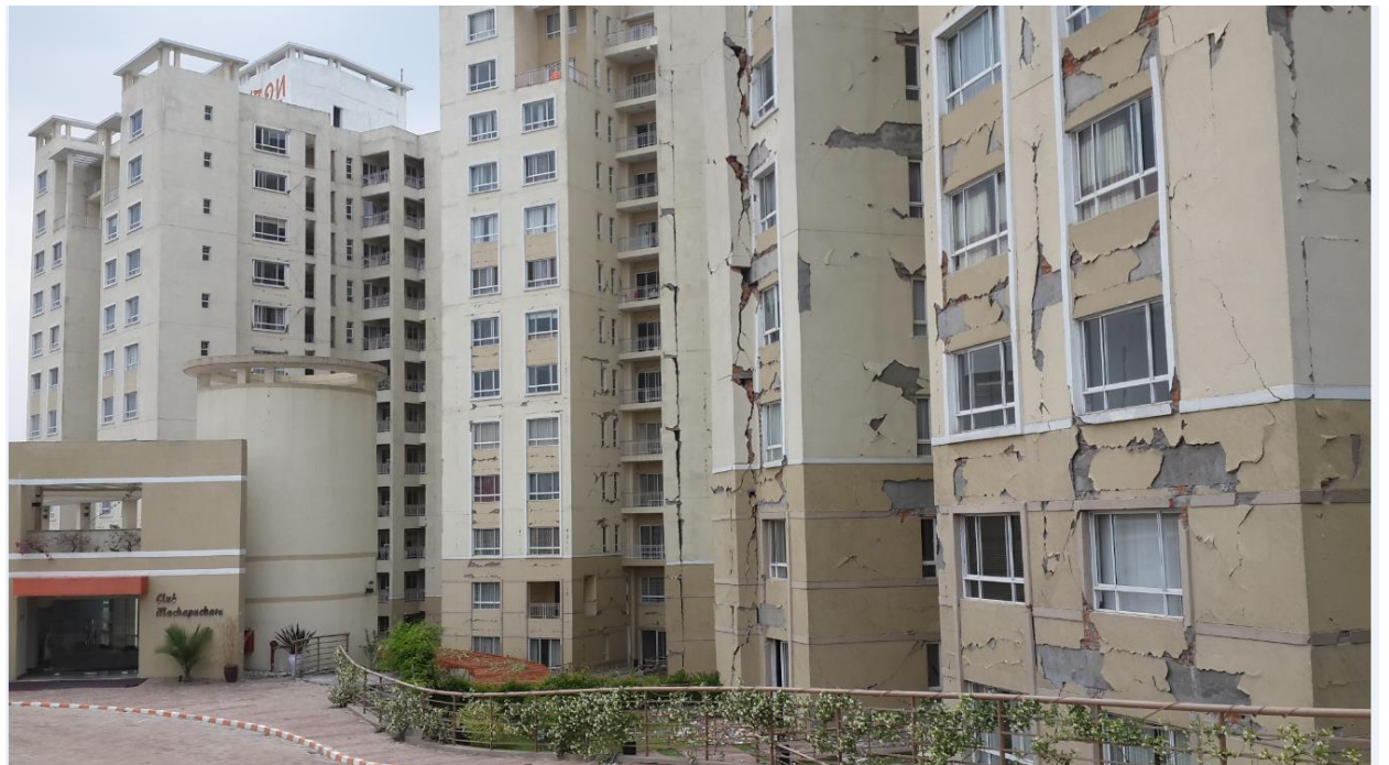
Left face of the building. Damage to the middle part of the structure may be attributed to the higher mode participation. (Photo by Kiran)
