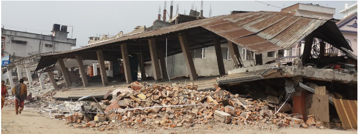
Collapse of a two story frame structure in Sitapaila, Kathmandu. Column bases on the upper story are also damaged. ( Photo by Kiran )
