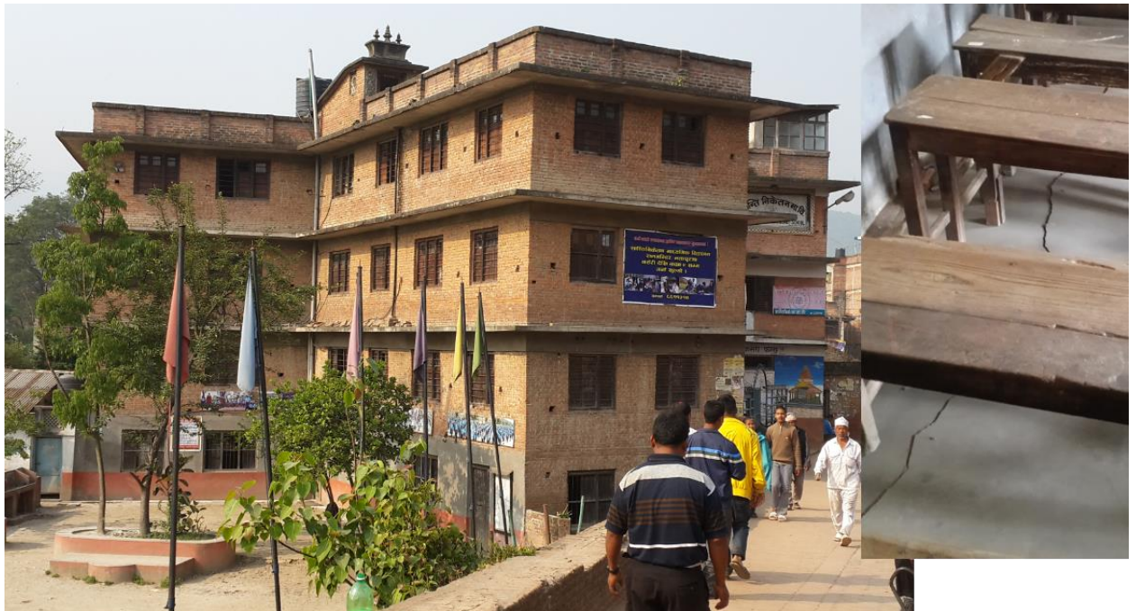
This "Y" Shaped 4 story school building has no cracks on the walls except on the floor of one room on ground floor, shown aside. (Photo by Kiran)
