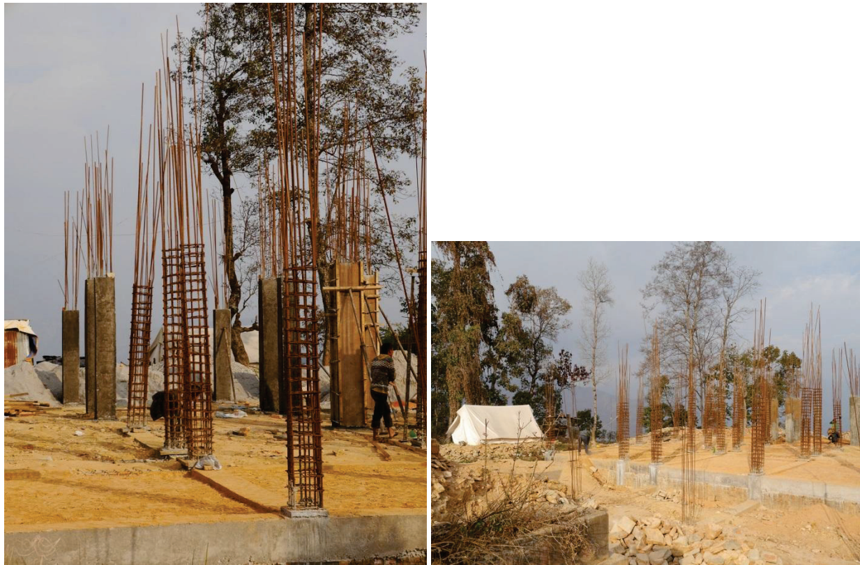
Figure 3 Photos of UNDP building under construction.
