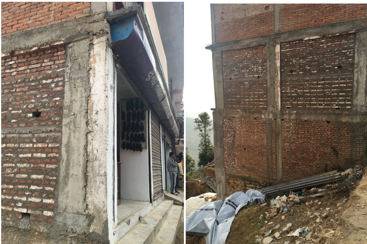
Figure 5 Photos of apartment building retrofitted with column jacketing on lower floors.
