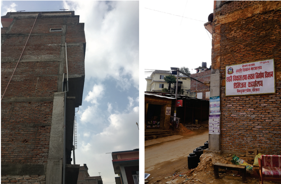
Figure 4 Photos of apartment building retrofitted with fiber-wrapped columns.
