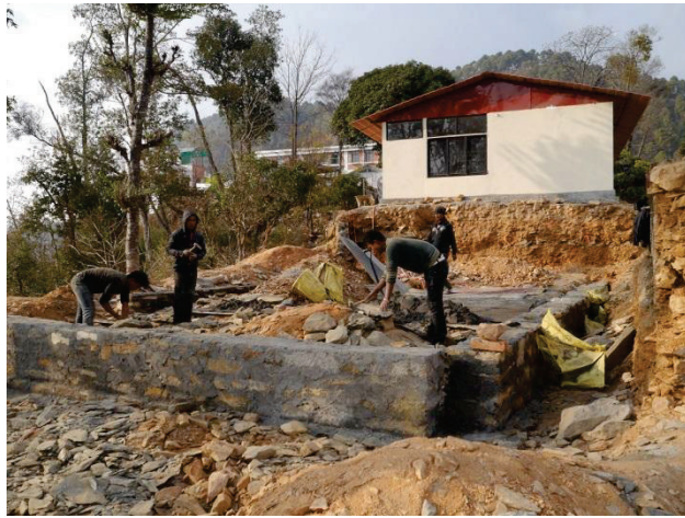
Figure 9 New eye clinic under construction.
