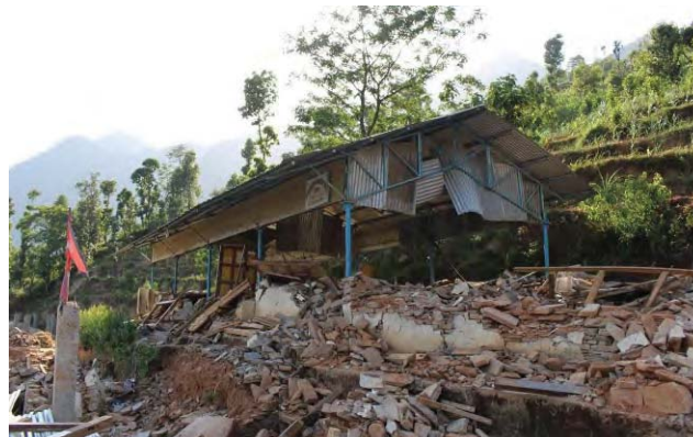
Figure 3. Collapsed school building
