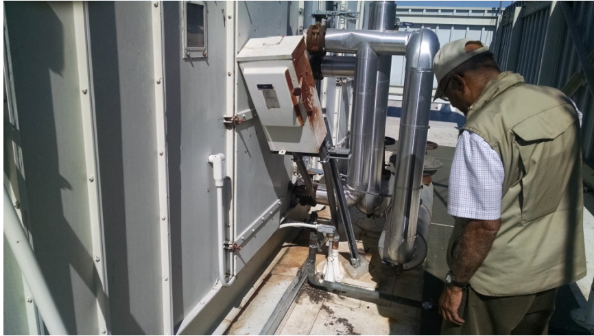
South Nursing Wing Roof electrical panel damage
