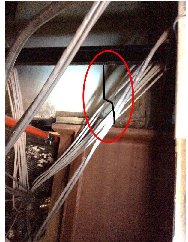
Main Hospital Crack in Precast Beam
