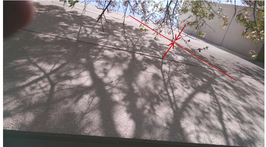
South Wing Nursing Tower ICU 2nd floor exterior wall (stucco on stud walls) leaning out ½"
