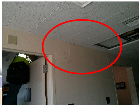
Crack in partition wall below cracked beam
