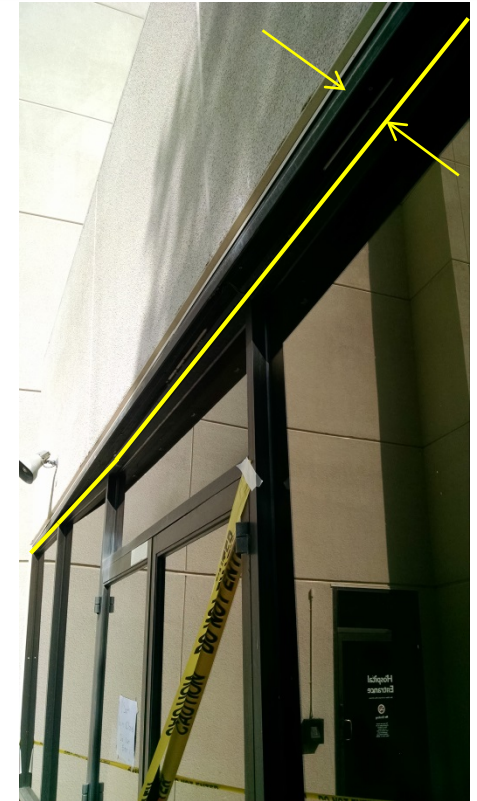
Damage with displacement of storefront entrance and window system
