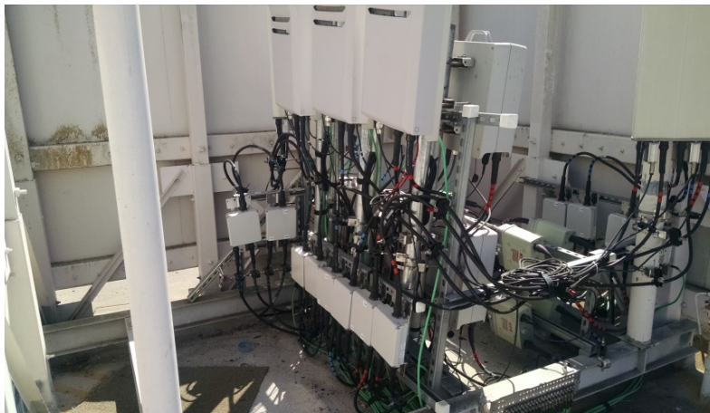
Main hospital roof telephone rack severely out of plumb
