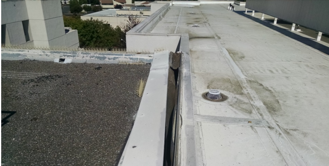
South Nursing Wing North Elevator Tower Seismic Joint Damage
