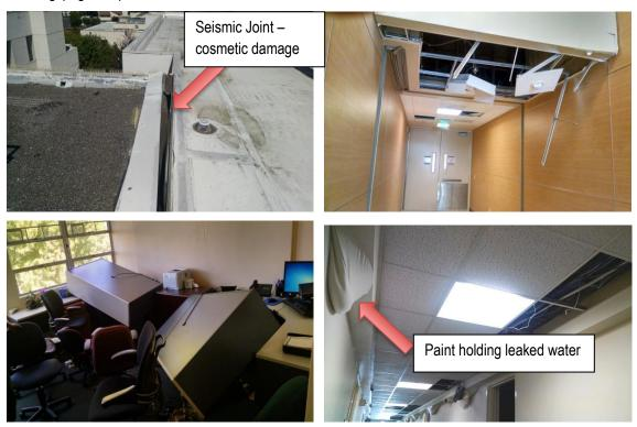
Figure 1: Observed damage in Queen of the Valley Hospital
