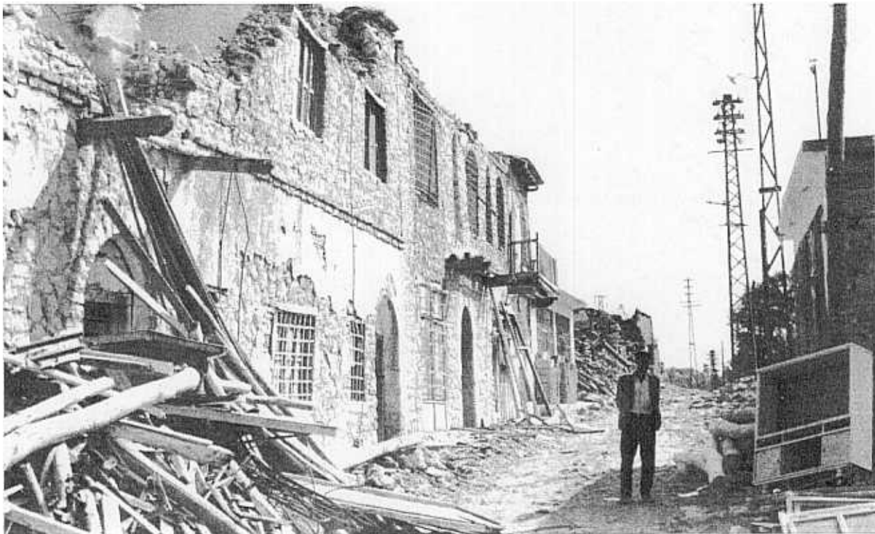
TY' DAL RE UT' DAMAGED SEC CEMENT MORT RAL
