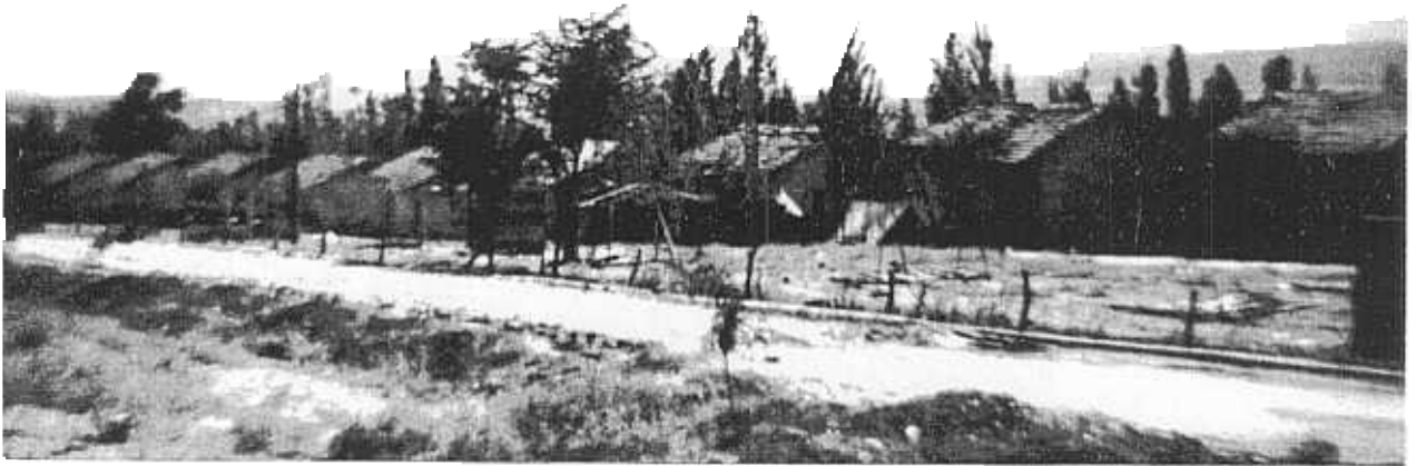
FIGURE 70 A ROW OF LIGHTLY DAMAGED EARTHQUAKE-RESISTANT HOUSES BUILT BY THE MRR AND ERI FOLLOWING THE 1971 BINGÖL EARTHQUAKE.
