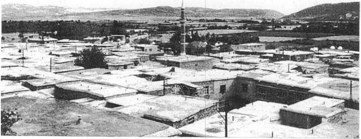
FIGURE 40 VIEW ACROSS MOSTLY UNDAMAGED DWELLING ROOFS IN HANI.
