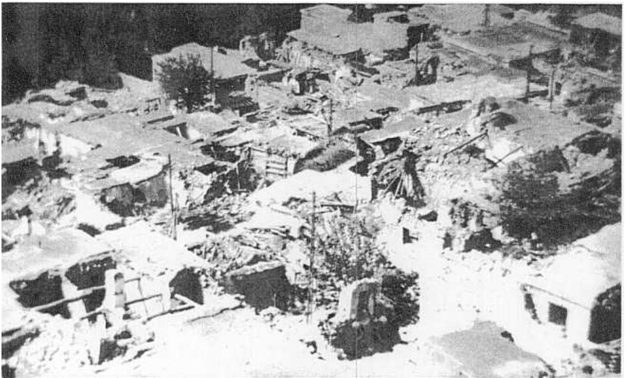
FIGURE 56 GENERAL VIEW OF A SECTION OF LICE THAT SUFFERED LESS DAMAGE TO THE MUD ROOFS.
