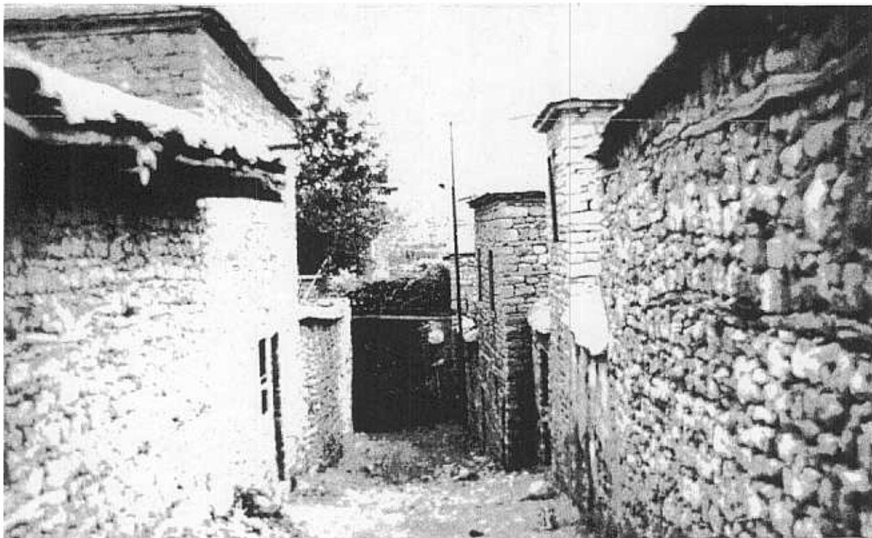
FIGURE 42 TYPICAL HOUSES IN HANI.
