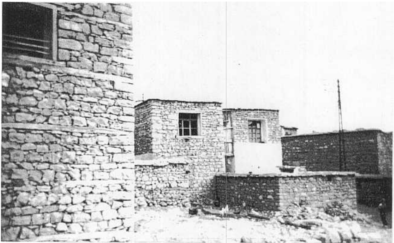
FIGURE 41 TYPICAL HOUSES IN HANI
