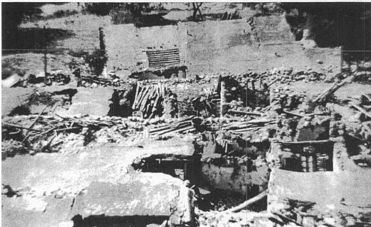
FIGURE 57 VIEW OF COLLAPSED ROOFS IN LICE. THE INTACT ROOFING TIMBERS HAVE BEEN PULLED OUT FROM THE RUINS, PRESUMABLY FOR RECONSTRUCTION.
