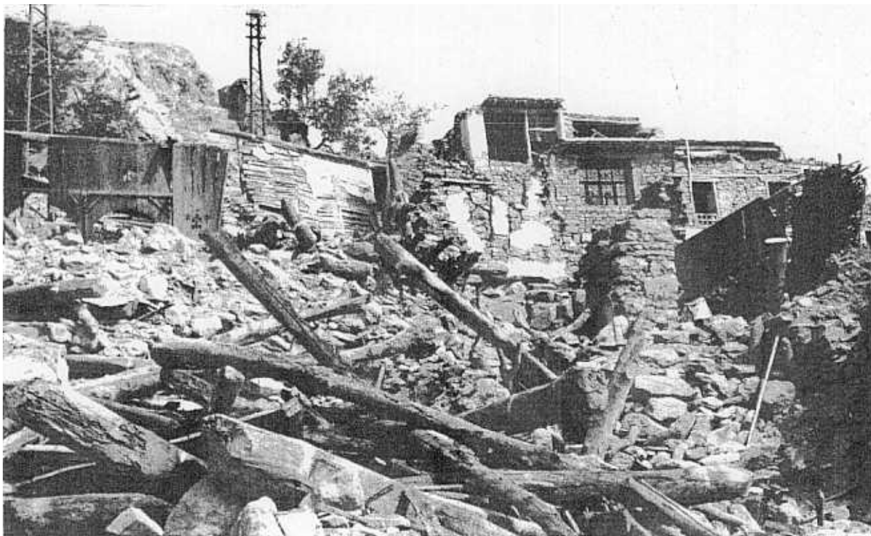
FIGURE TYPICAL VIEW OF TOTAL COLLAPSED HOUSE ICE
