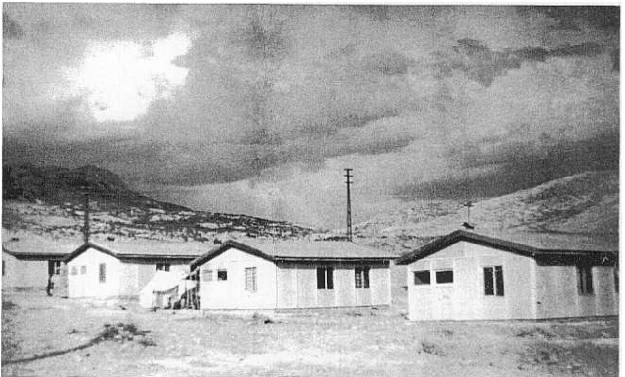
FIGURE 71 UNDAMAGED EARTHQUAKE-RESISTANT HOUSES IN HANI.
