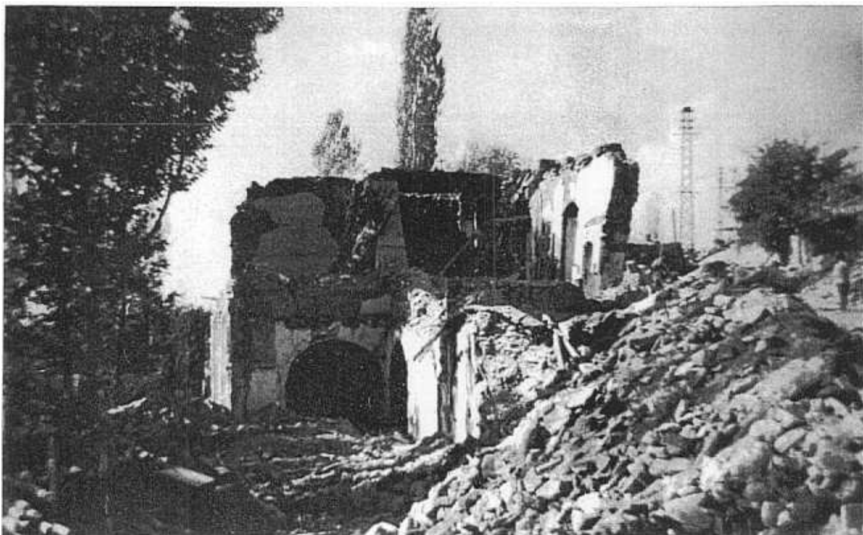
FIGURE 6 PARTIAL COLLAPSE OF AN ANCIENT BUILDING
