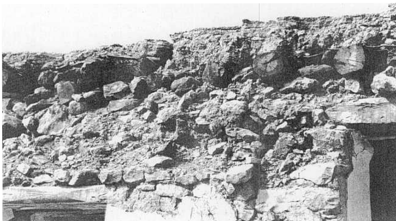
FIGURE 47 DETAIL OF A CONNECTION BETWEEN THE ROOFING TIMBERS AND AN EXTERIOR WALL.
