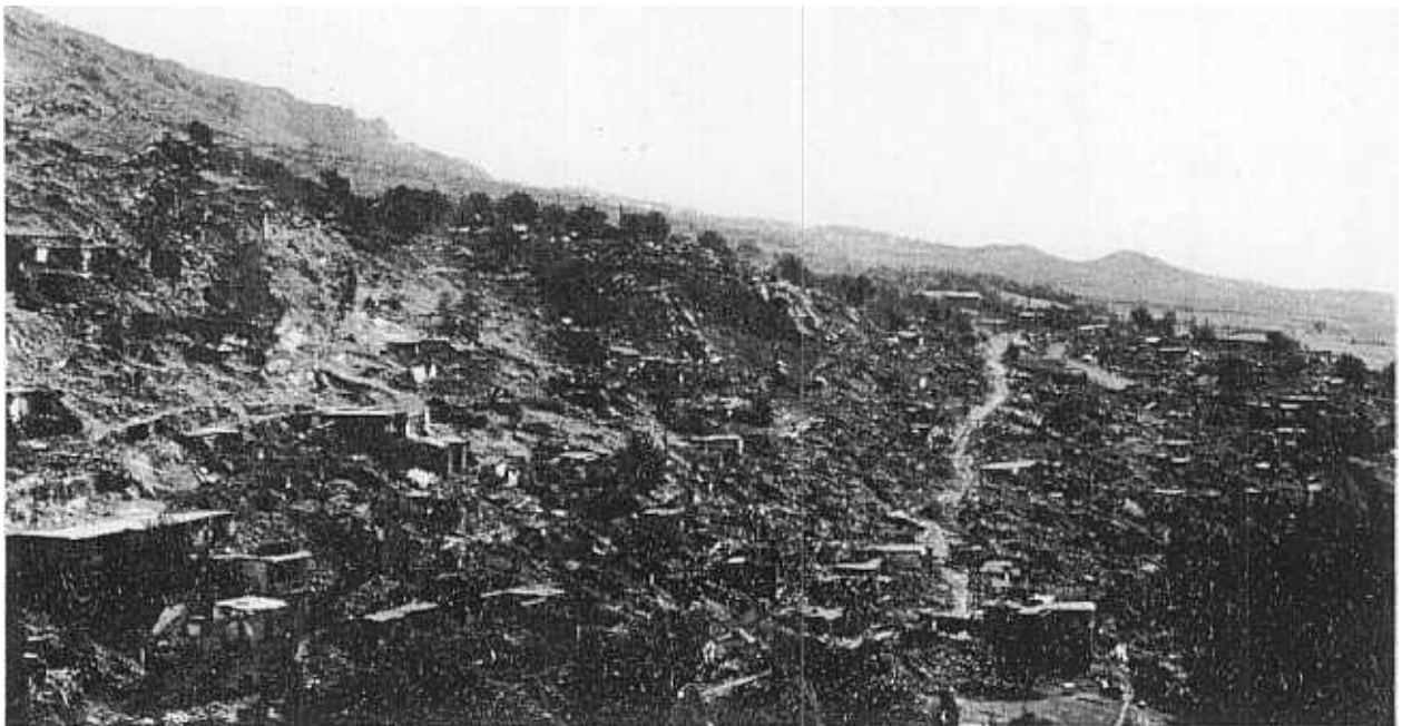
FIGURE 60 GENERAL VIEW ACROSS THE DEVASTATED EASTERN SECTION OF LICE.
