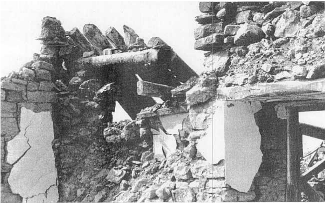
FIGURE 49 TYPICAL FAILURE OF A ROOF IN LICE.
