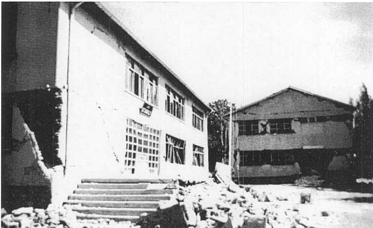
FIGURE 28 ANOTHER HIGH SCHOOL BUILDING THAT SUFFERED NEARLY TOTAL DAMAGE. NOTE THAT THE SECOND FLOOR WALLS ARE NOT AS SEVERELY DAMAGED.
