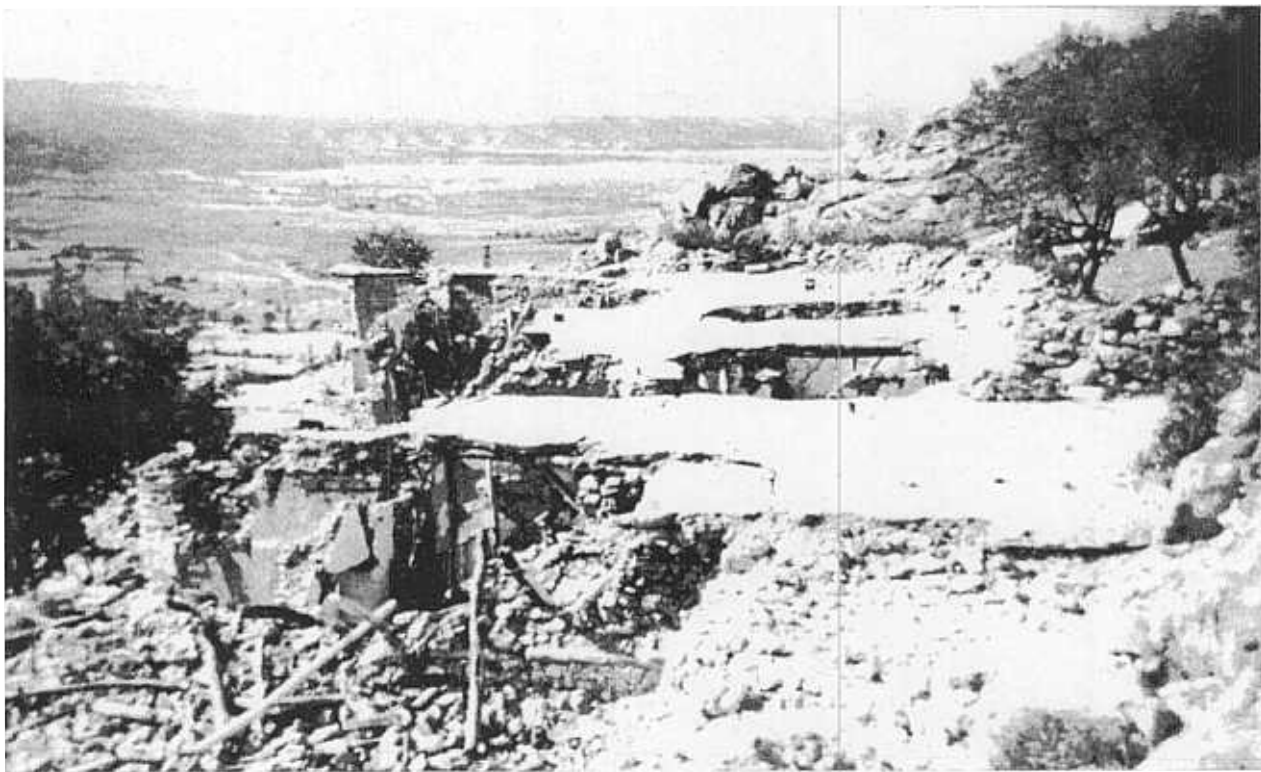
FIGURE 54 VIEW ACROSS SEVERAL PARTIALLY COLLAPSED ROOFS IN LICE.
