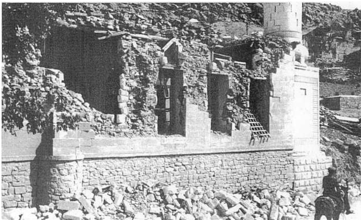
FIGURE 64 A PARTIAL COLLAPSE OF A MOSQUE
