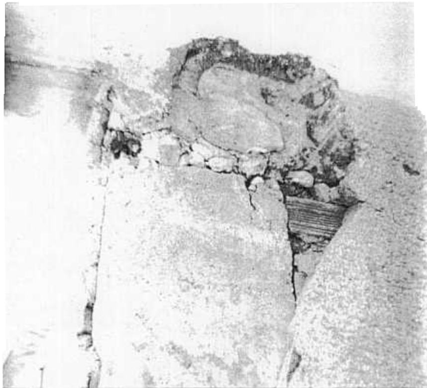
FIGURE 14 DETAIL OF A DAMAGED COLUMN IN THE MUNICIPAL BUILDING SHOWING DAMAGE IN AN AREA OF APPARENTLY POOR CONCRETE PLACEMENT.
