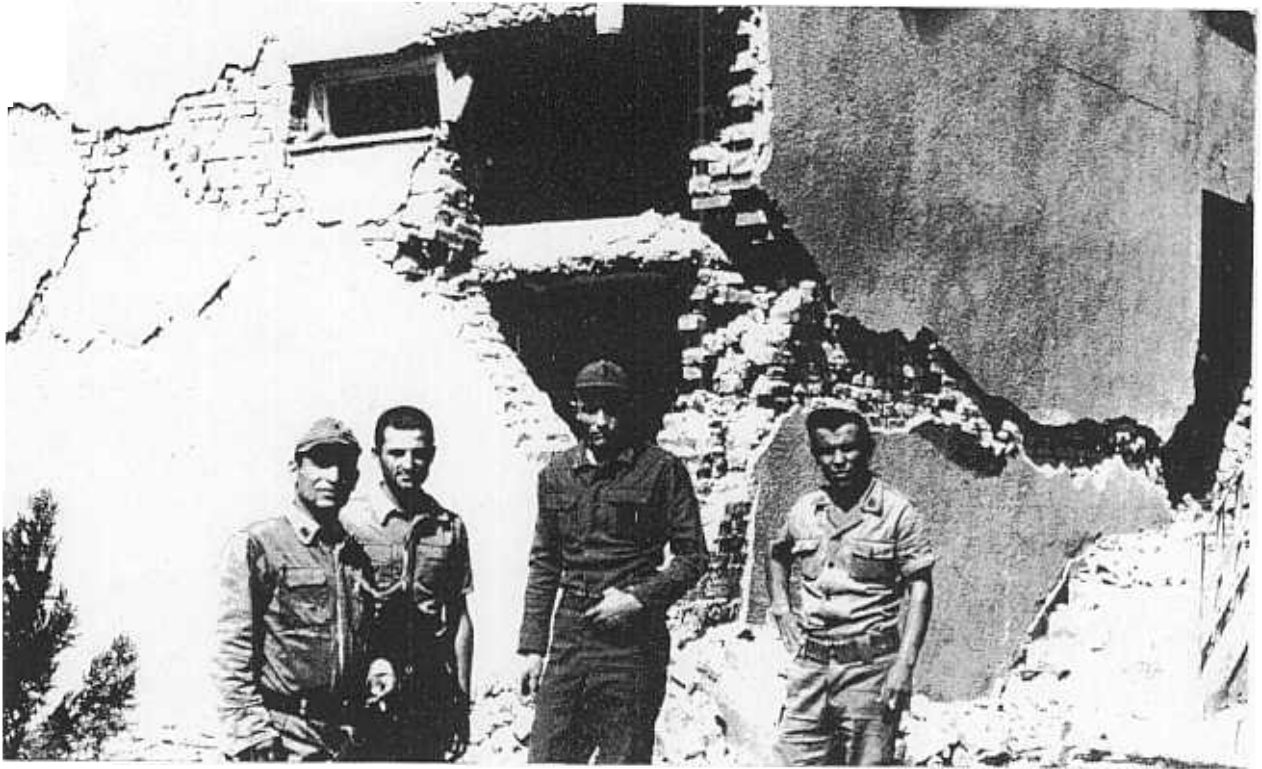
FIGURE ONE THE FIRST DOOR CORNERS THE POLICE BUILDING SHOWING WHAT SEEMS DAMAGE DUE TORSION AND POUNDING BETWEEN THE FLOOR SLABS AND THE WALLS
