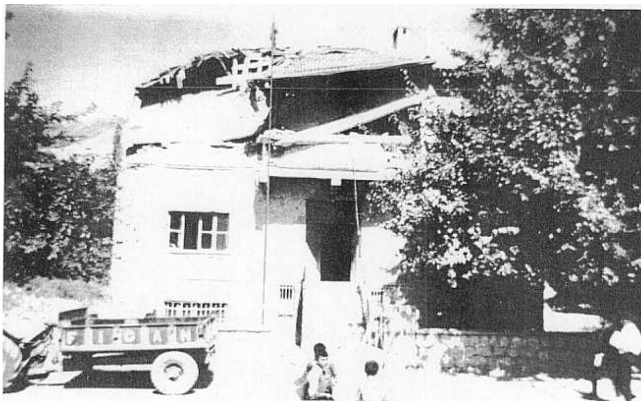
FIGURE 16 A PARTIALLY COLLAPSED MASONRY GOVERNMENT BUILDING IN LICE
