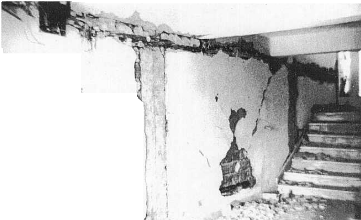
FIGURE 13 INTERIOR OF THE ENTRANCE HALL OF THE MUNICIPAL BUILDING SHOWING DAMAGE TO THE FRAME AND THE INFILL WALLS.
