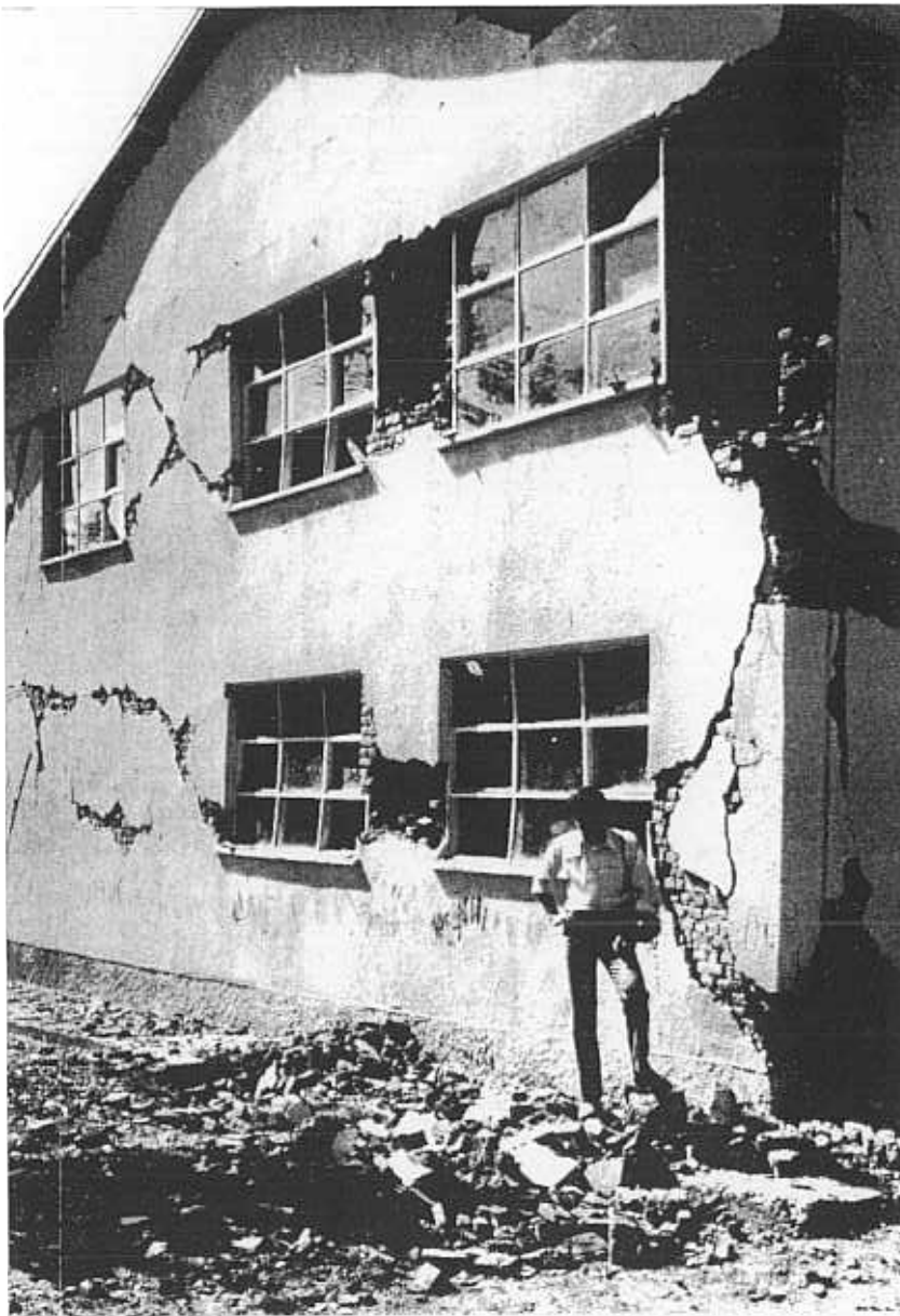
FIGURES 23 AND 24 THE EAST END WALL OF ONE OF THE HIGH SCHOOL BUILDINGS. ALL LATERAL RESISTING ELEMENTS OF THE WALL ON BOTH FLOORS WERE SHATTERED.
