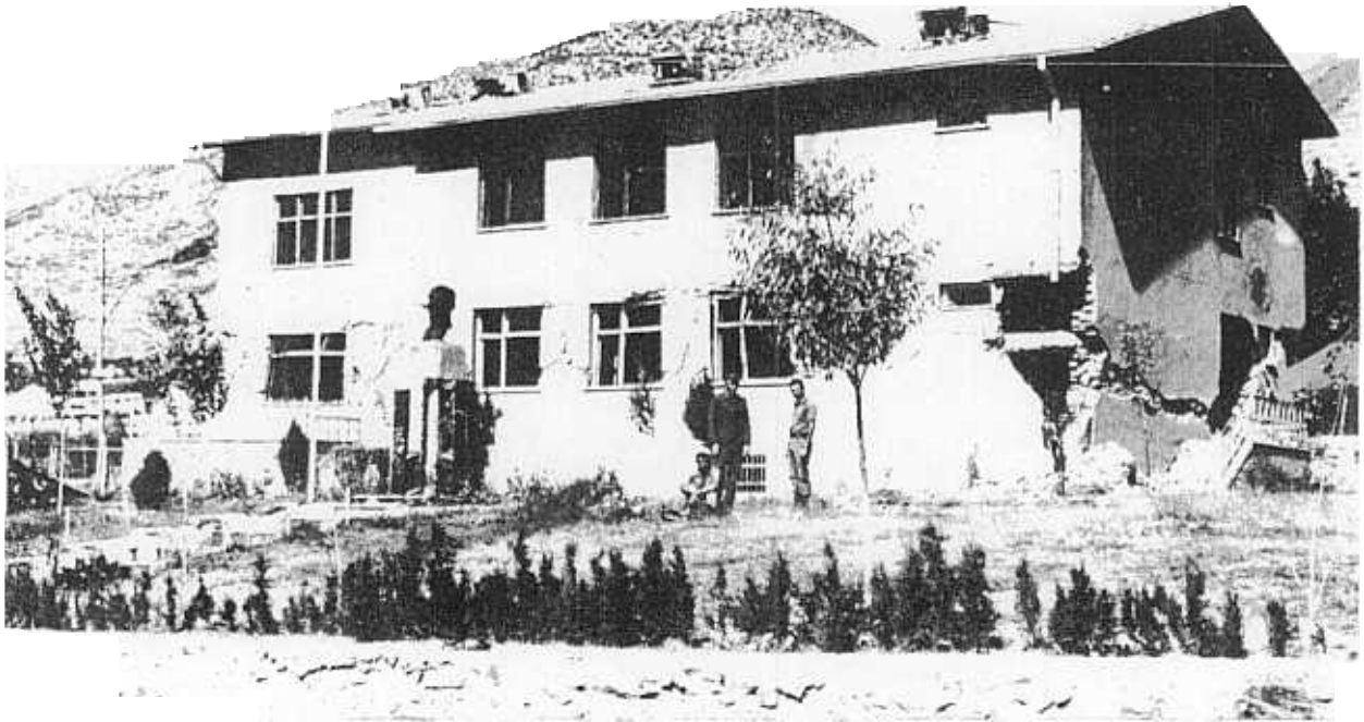
FIGURE 18 THE POLICE BUILDING IN LICE. THE LOWER STORY IS VERY SEVERELY DAMAGED, WHILE THE SECOND STORY IS LESS DAMAGED.
