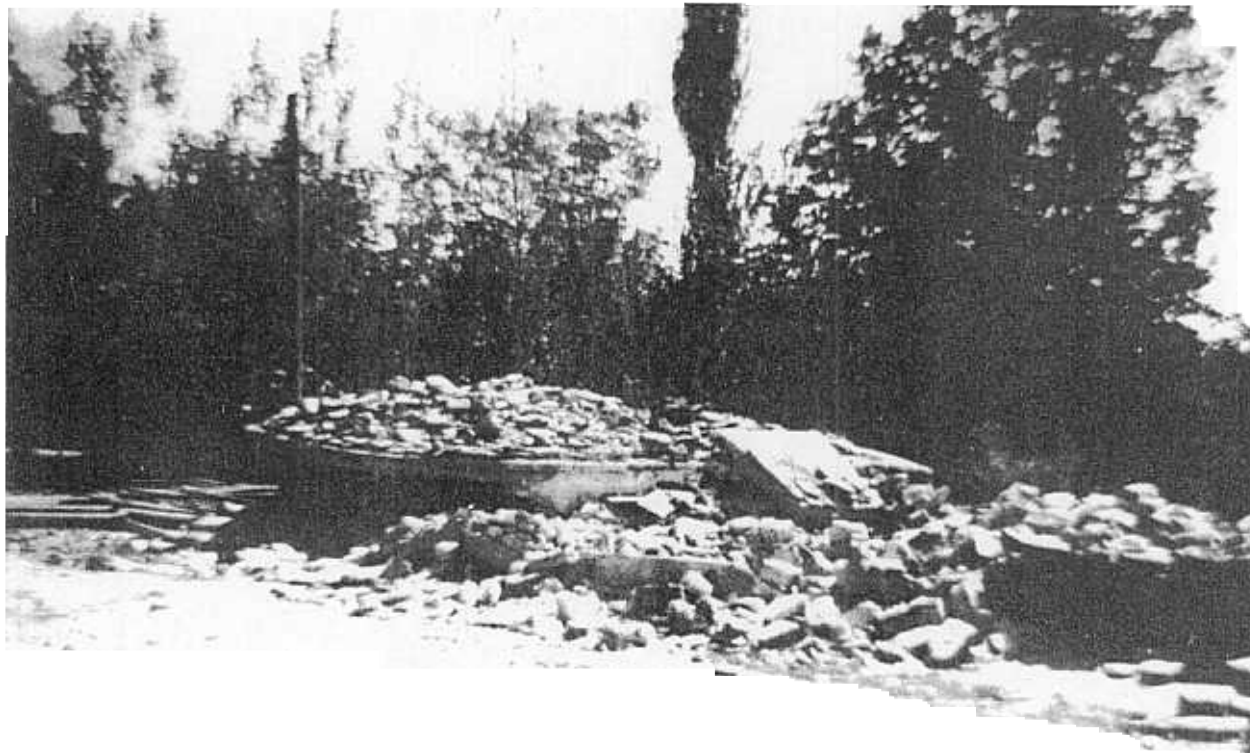
FIGURE 17 A COLLAPSED MASONRY STORE IN THE CENTER OF LICE.
