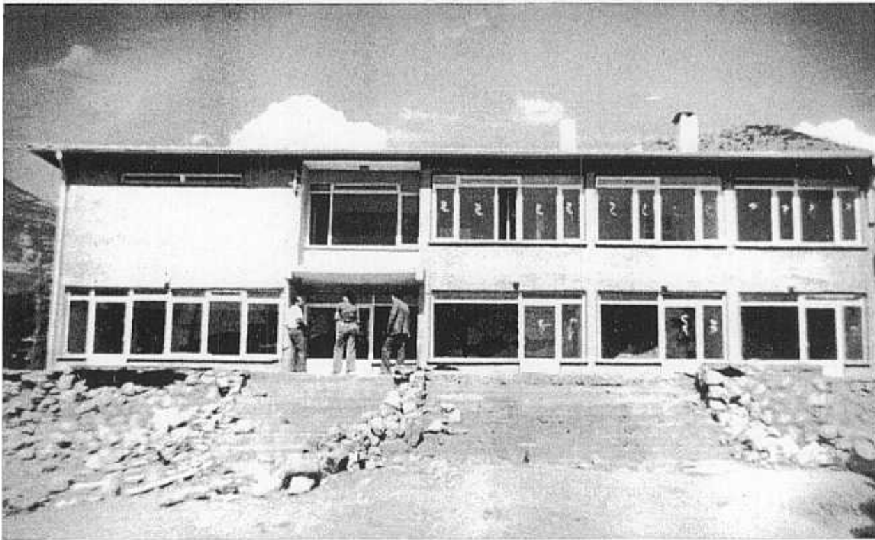
FIGURE 12 THE NEW REINFORCED CONCRETE MUNICIPAL BUILDING, ONE OF THE FEW ENGINEERED BUILDINGS IN THE AREA. IT SUFFERED MODERATE DAMAGE TO THE FRAME AND SIGNIFICANT DAMAGE TO ITS INFILL WALLS
