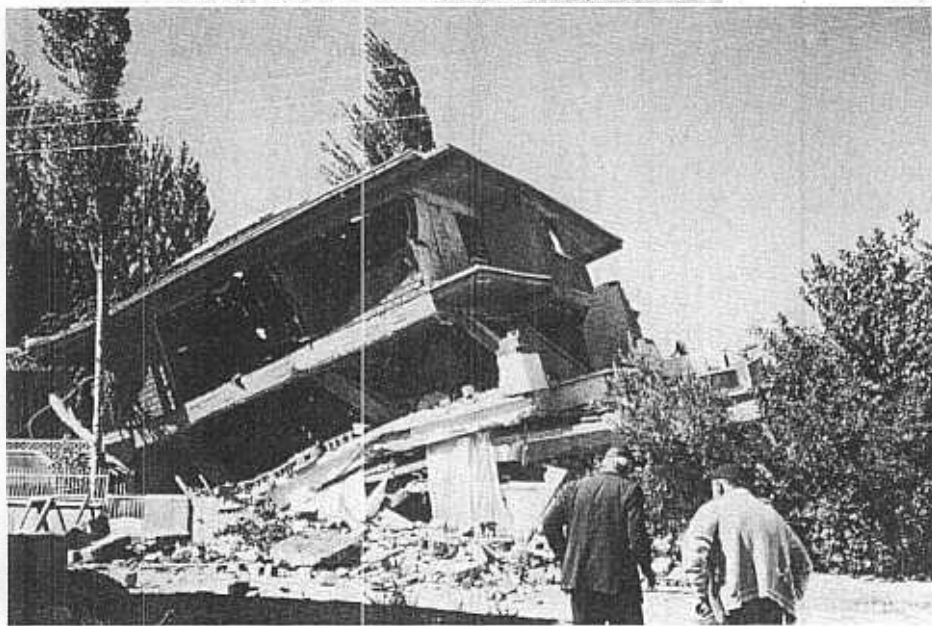
Figure 2 - Typical case of the total collapse of a four-story R/C building.
