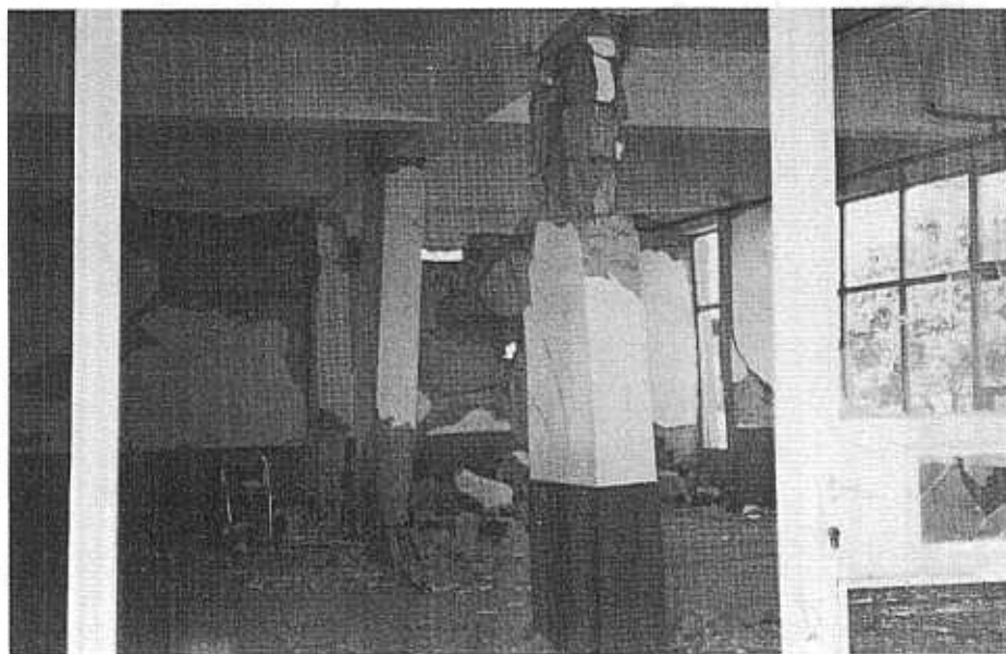
Figure 7 - Damage to soft story columns.
