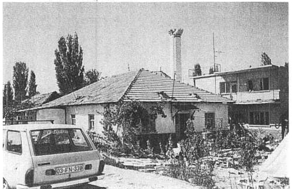
Figure 11 - Chimneys were chopped off in the downtown area.
