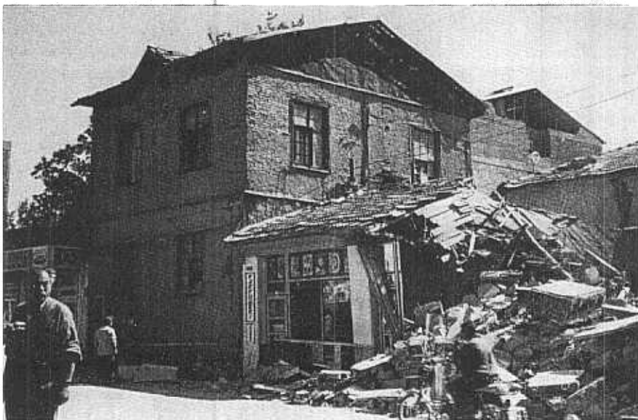
Figure 6 - Damage to an adobe building.
