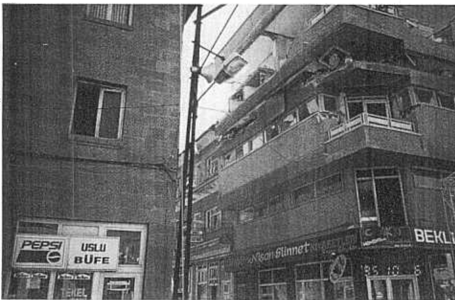
Figure 9 - Failure of middle story due to pounding.
