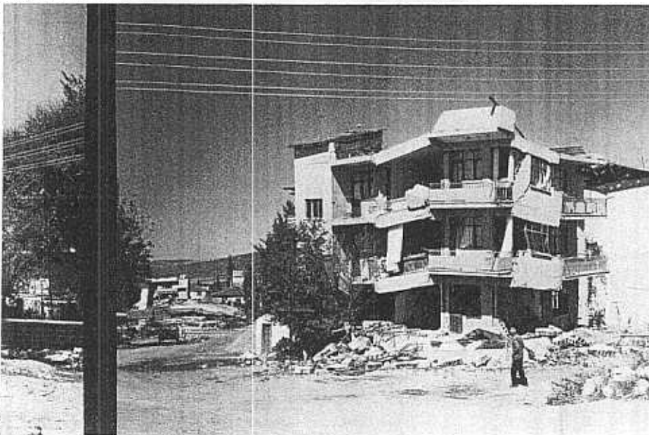
Figure 5 - Most R/C buildings in the downtown area collapsed or were severely damaged.
