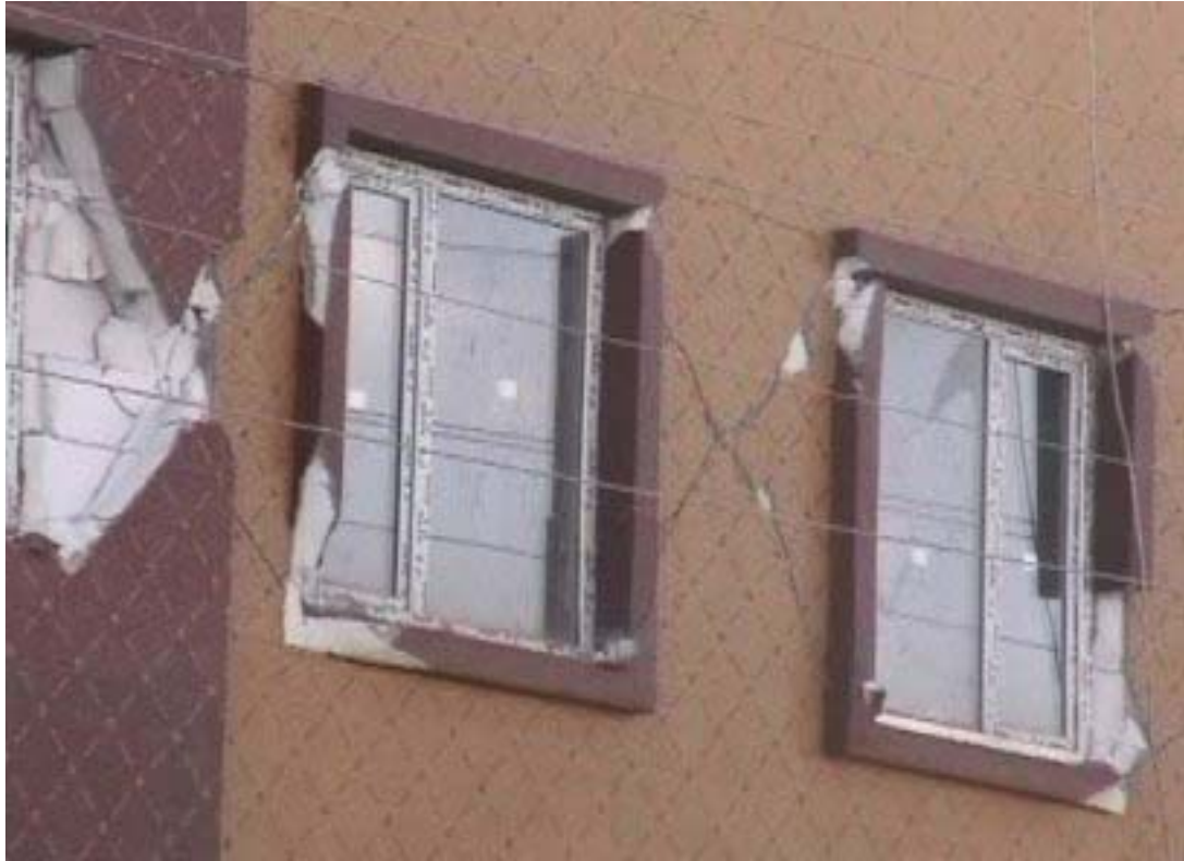
Figure 31. Typical shear crack in infill wall.
