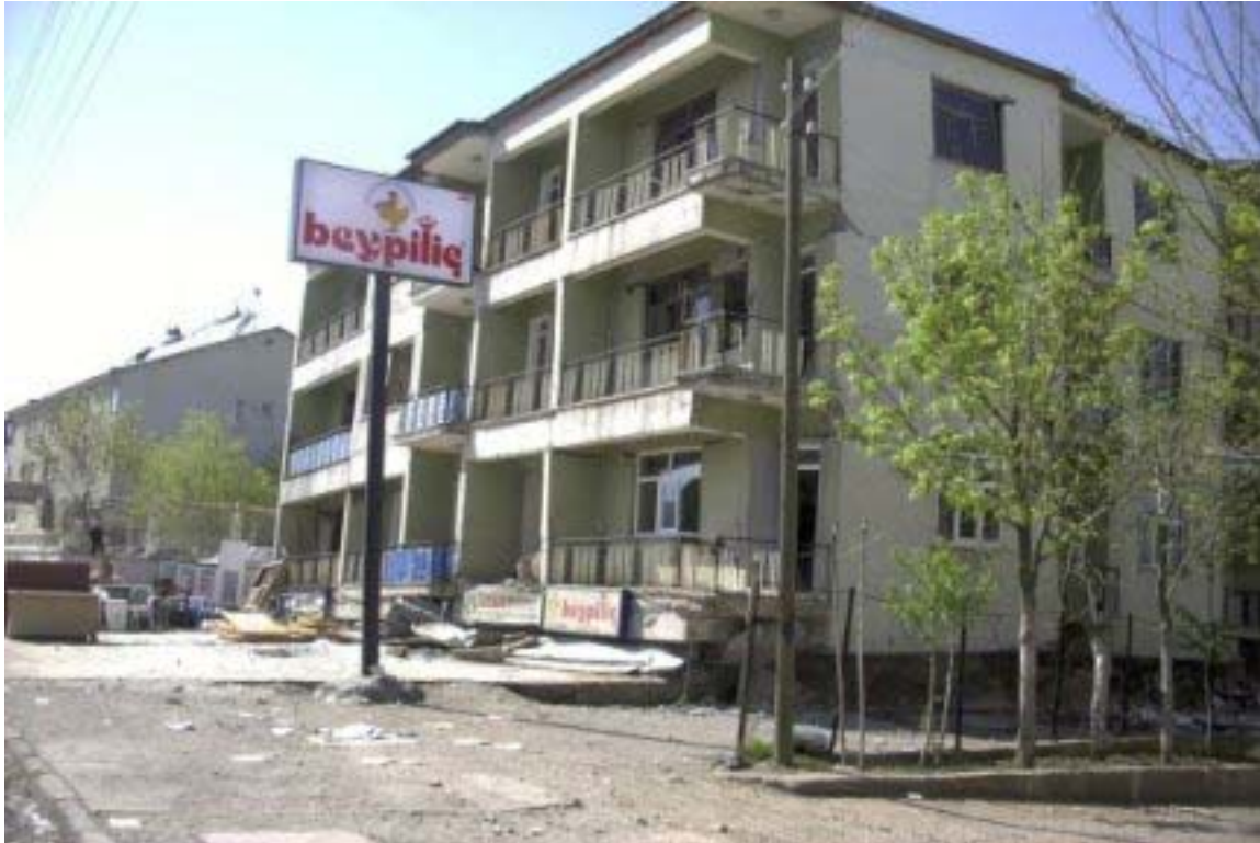
Figure 29. Collapsed 4-storey building due to soft storey.
