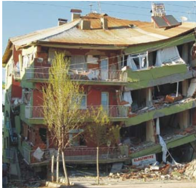
Figure 40. Typical First Story Collapses (After Emre et.al, 2003)
