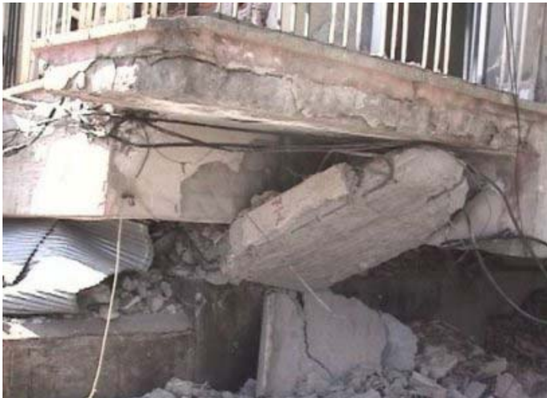
Figure 31. Typical shear crack in infill wall.
