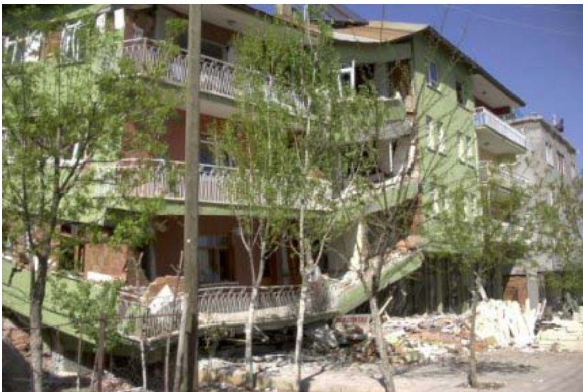
Figure 29. Collapsed 4-storey building due to soft storey.
