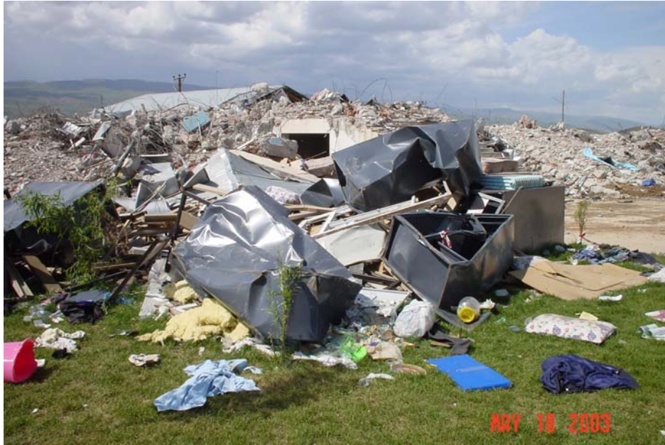
Figure 13. The remains of steel lockers and beds which partially supported some of the fallen material in the Celtiksuyu Boarding School
