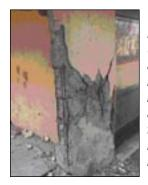
Figure 9. Shear failure at column base due to insufficient amount of transverse reinforcement.
