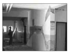
**Figure 10.** Observed shear failure at shear wall due to insufficient transverse reinforcement and poor concrete quality.
