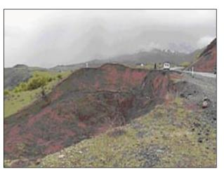
*Figure 7.* One of the most significant seismically induced landslides along the Sogukcesme section of the country roadway extending from Bingöl to Karliova.
