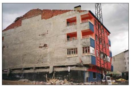
*Figure 16.* A collapsed building in the close vicinity of the southern cliff crest of the Gayt Stream valley.
