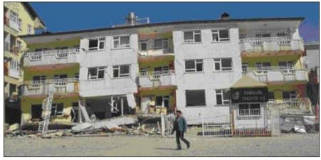
Figure 17. Typical first-story collapse.
