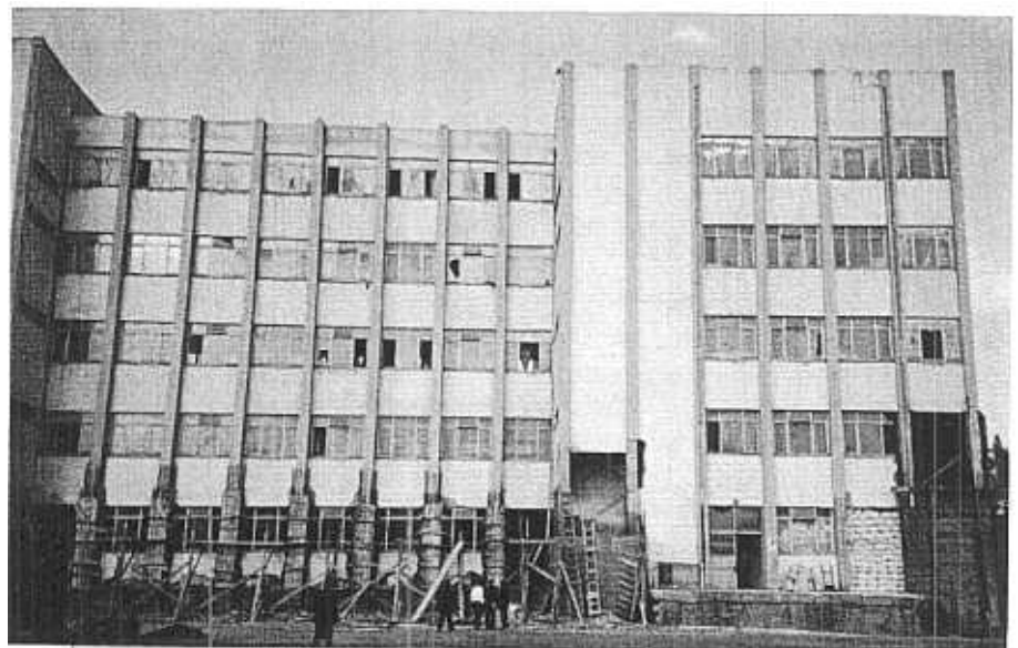
Figure 3 - Unsan Flour Mill during repair and retrofit
