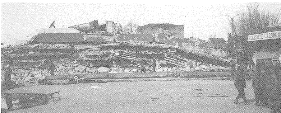
FIGURE 5 - Complete collapse of a five-story, concrete frame hotel building
