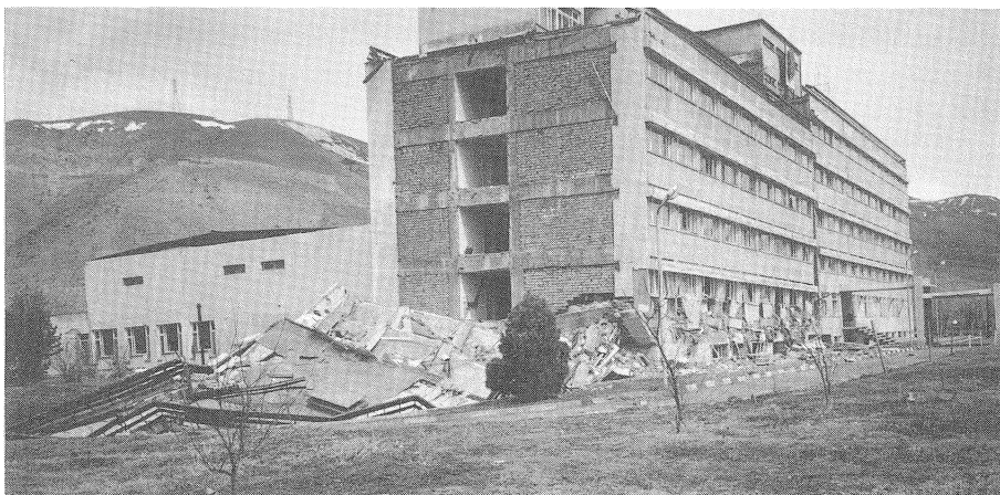
FIGURE 6 - First story short column shear failure at military hospital
