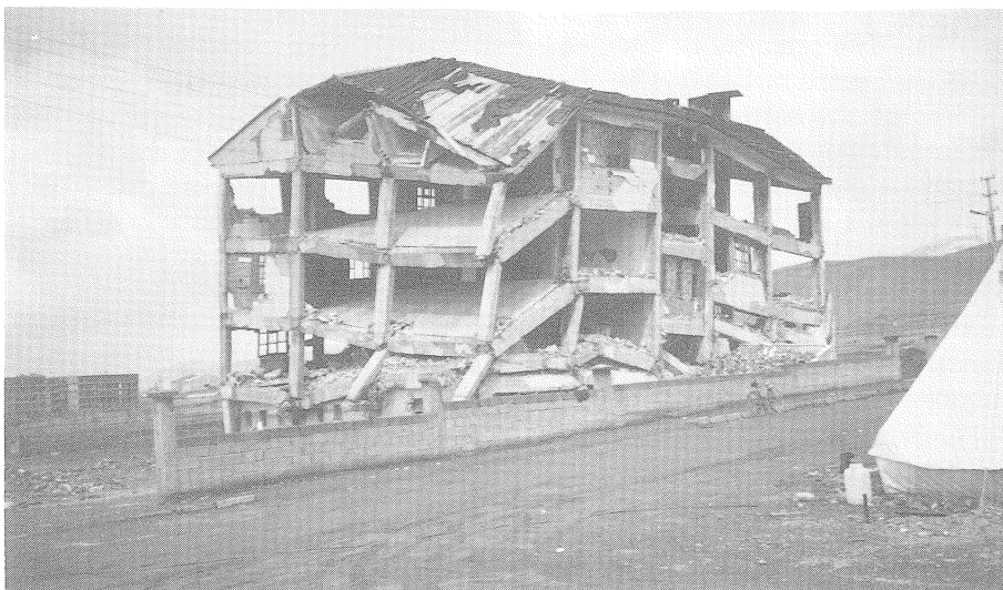
FIGURE 4 - Partially collapsed mid-rise residential building
