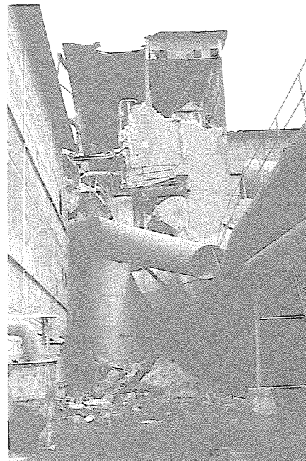
FIGURE 7 - Collapsed stack at a sugar refinery
