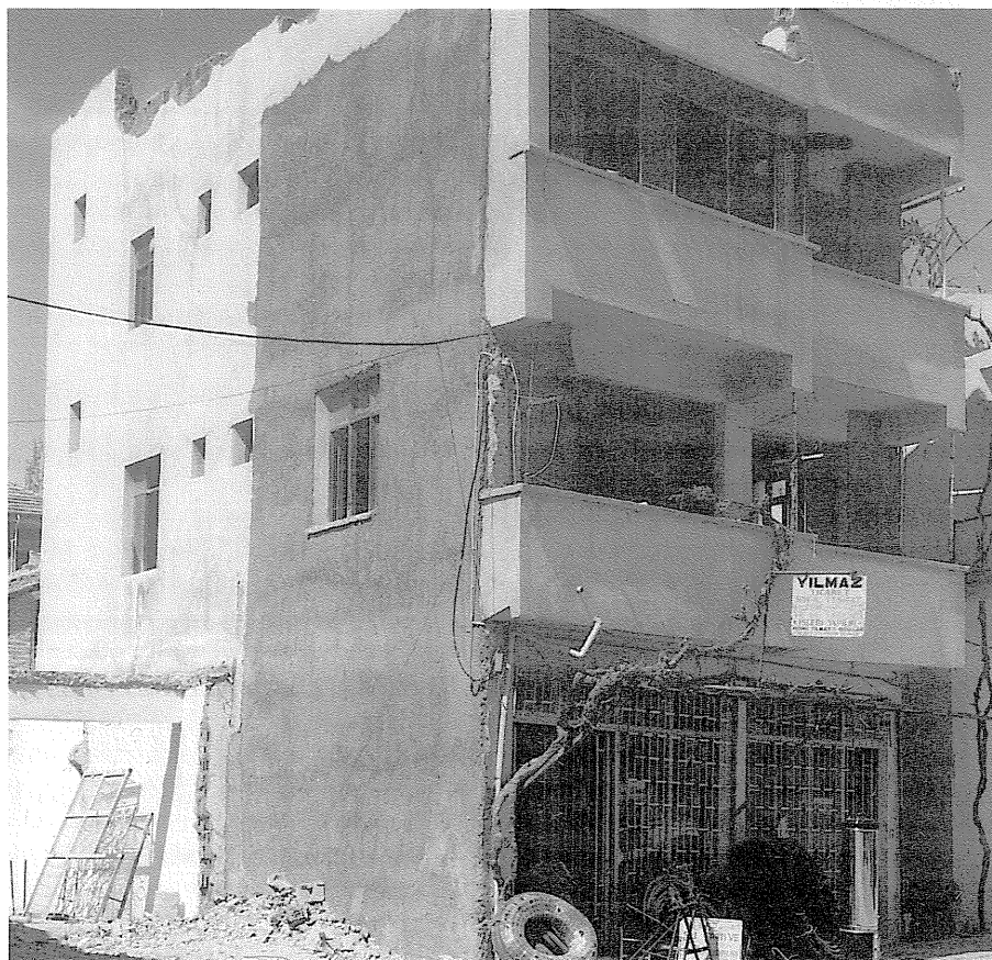
Figure 13 - Masonry building retrofitted by bonding a layer of R/C grout shell on the outside walls. Pre-existing fourth story removed for weight.
