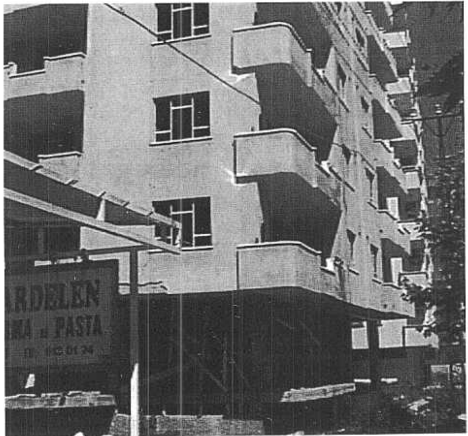
Figure 9 - Soft first story of new construction resulted in cracks in columns.
