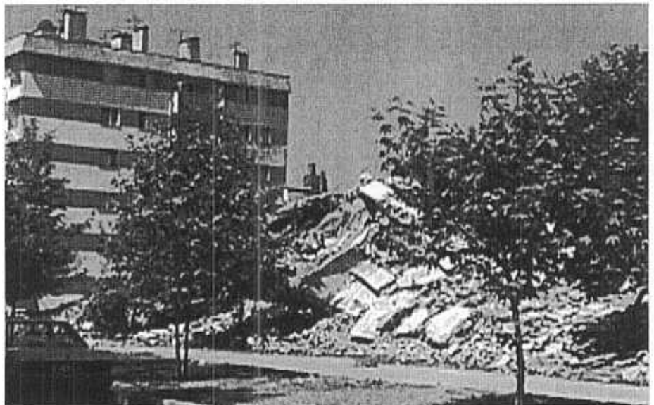
Figure 5 - Ceyhan: unoccupied new eight-story structure pancaked.
