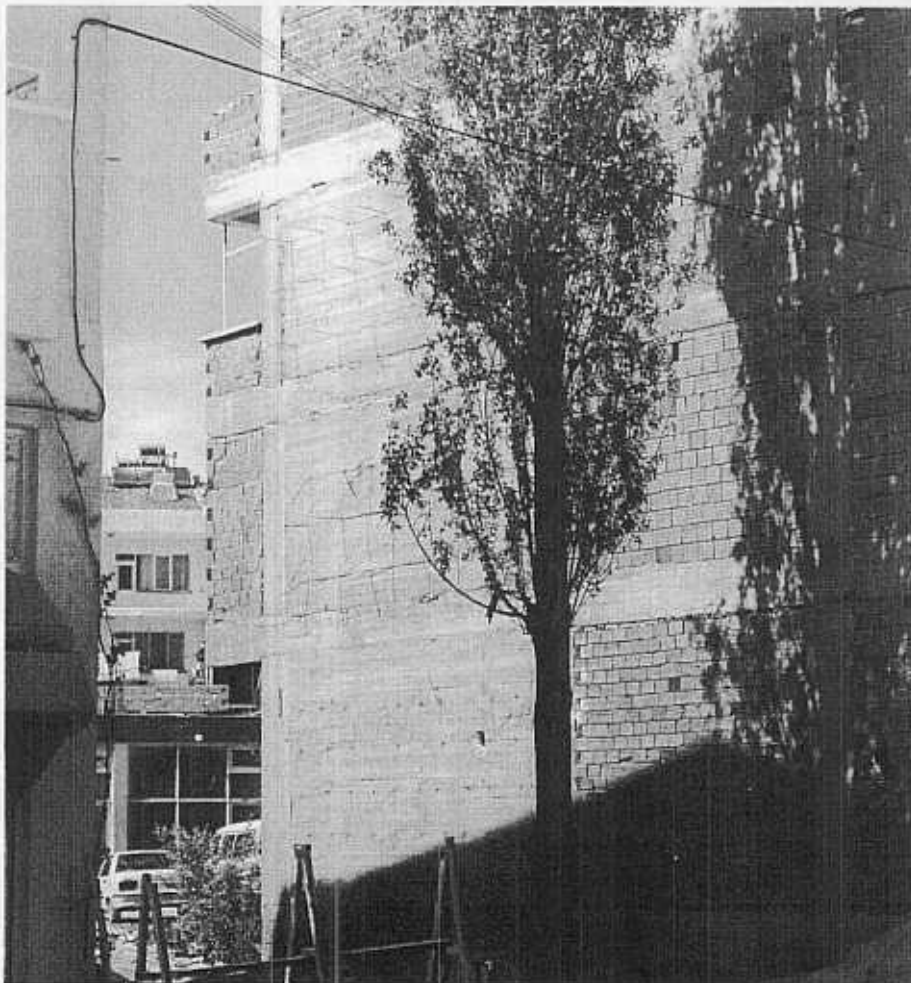
Figure 10 - Reinforced concrete building retrofitted by shear wall insertion.
