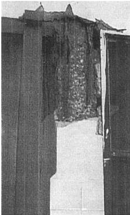
Figure 6 - Deficient shear reinforcement at top end of column at Çukurova University. Photo: Çelebi
