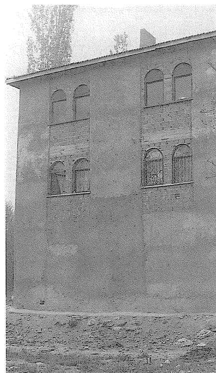
Figure 12 – Masonry house retrofitted by grout shell on outside walls.
