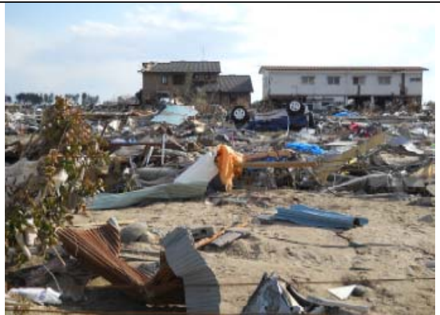
Photo 14: Steel construction remained standing in Arahama District
