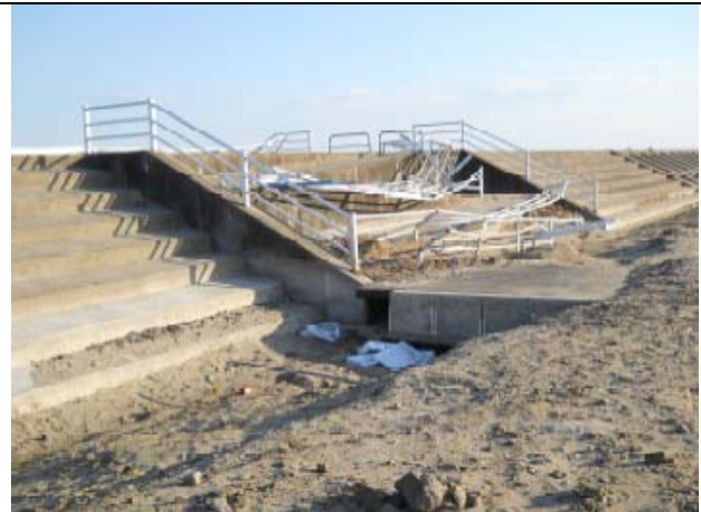
Photo 20: Damage of rails on the embankment (1).
