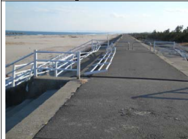
Photo 21: Damage of rails on the embankment (2).
