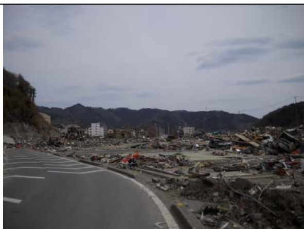
Photo 27: Totally destroyed houses in Zone C (3)
