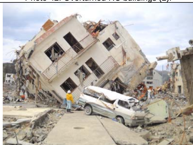
Photo 44: Overturned RC buildings (4).
