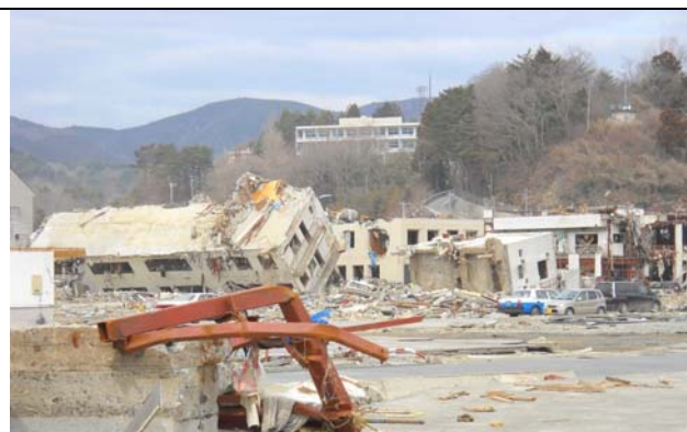
Photo 42: Overturned RC buildings (2).
