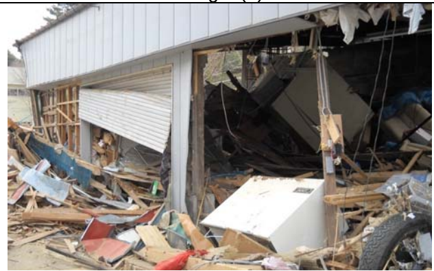
Photo 15: In the area where tsunami wave reached 1.8 m high, the first story was wrecked.
