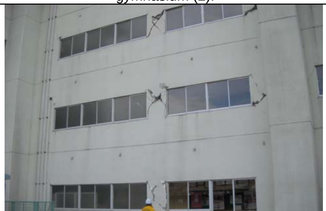
Photo 11: Shear cracks in mullion walls in the north.
