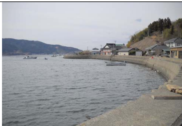
Photo 1: Tsunami wave flowed over 4-m high breakwater.
