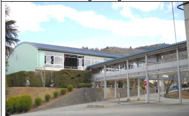
Photo 8: Window glasses were broken in the gymnasium (1).
