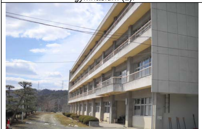
Photo 10: The school building suffered no damage.
