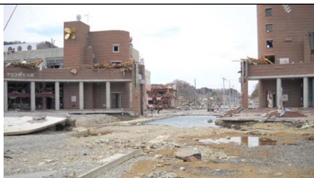
Photo 31: The corridor between the two buildings was washed away.
