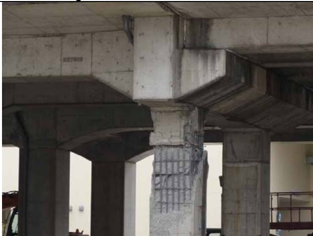
Photo 5: Viaduct of the Shinkansen Line, shear failure penetrated to the concrete core of the pier. Asuto Nagamachi 2-chome
