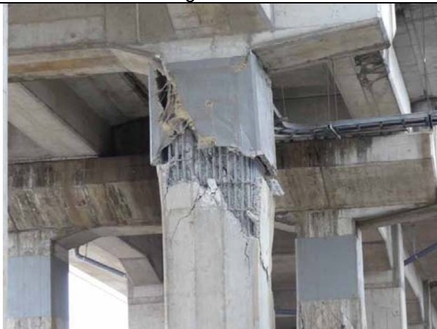
Photo 7: Fracture of retrofit fiber reinforcement sheet of a pier of the Shinkansen Viaduct Asuto Nagamachi 2-chome, Taihaku-ku
