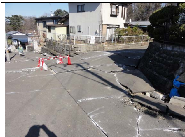
Photo 5: Failure of road surface. Oritate 5-chome, Aoba-ku
