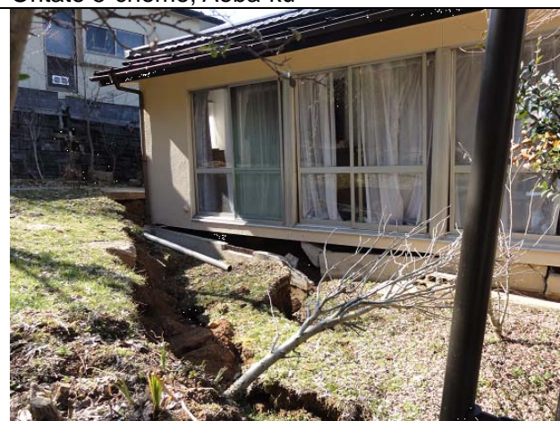
Photo 8: Ground settlement (80 cm). Oritate 5-chome, Aoba-ku
