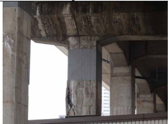
Photo 8: Shear failure of a pier below the fiber reinforcement retrofit of the Shinkansen Viaduct Asuto Nagamachi 2-chome, Taihaku-ku
