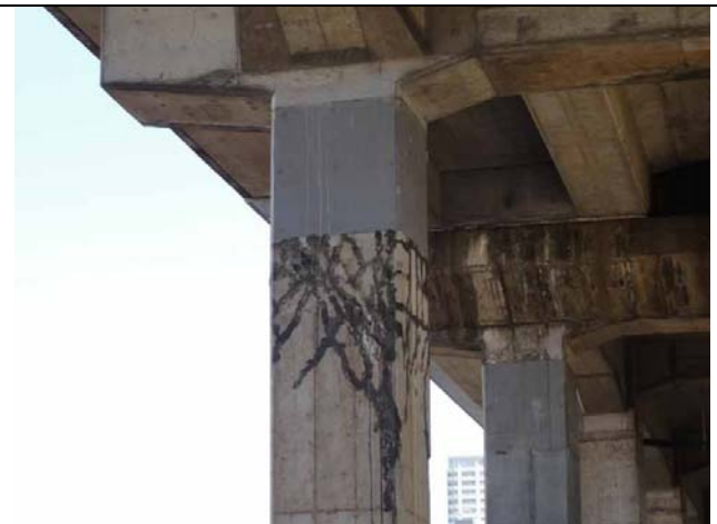
Photo 10: Shinkansen Viaduct, repair work (injection of plastic resin) below previous fiber reinforcement retrofit.
