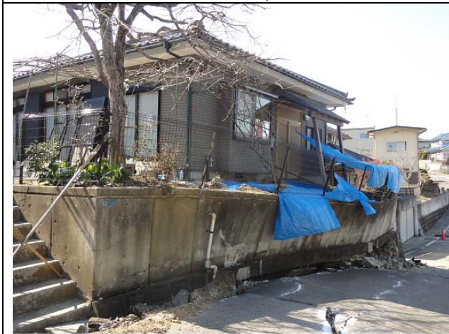
Photo 3: Failure of retaining walls. Oritate 5-chome, Aoba-ku
