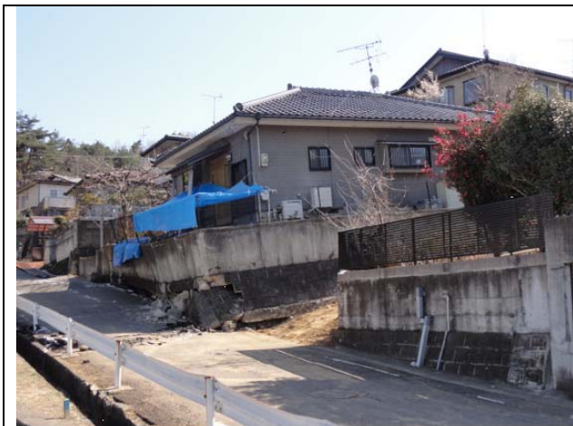
Photo 1: Failure of retaining walls. Oritate 5-chome, Aoba-ku
