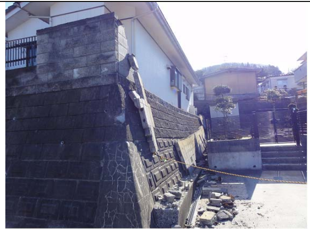
Photo 12: Fall of concrete block walls. Oritate 5-chome, Aoba-ku
