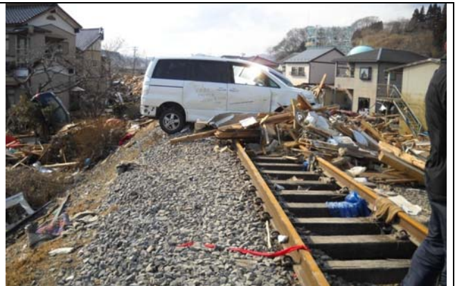
Photo 16: A car was left on the rail.
