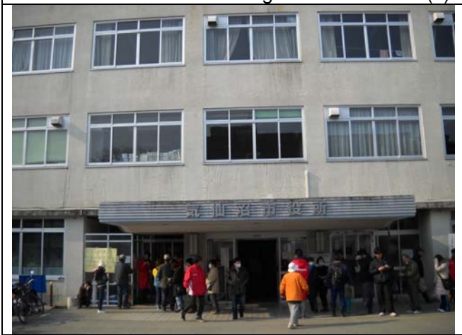
Photo 8: Kesen-numa City Municipal Building (1)
