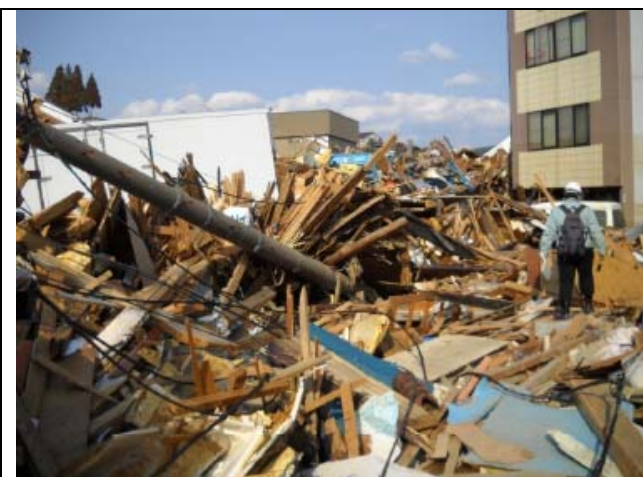
Photo 18: Damage in Kesen-numa City (1)
