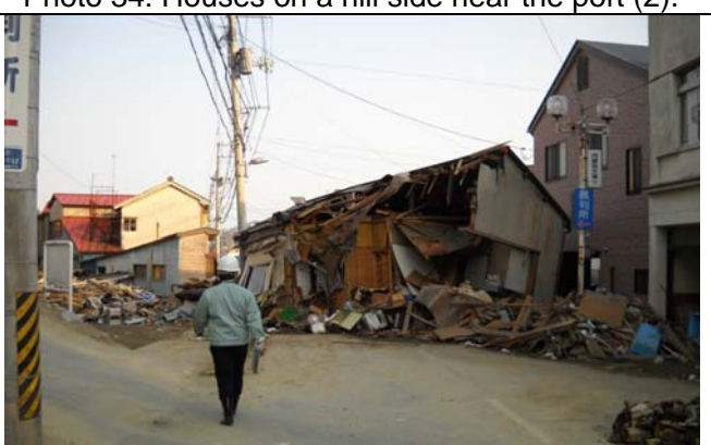
Photo 36: A collapsed traditional timber house due to ground shaking.
