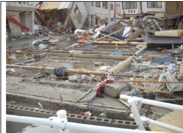
Photo 30: Total loss of timber houses above the foundation in the port area.
