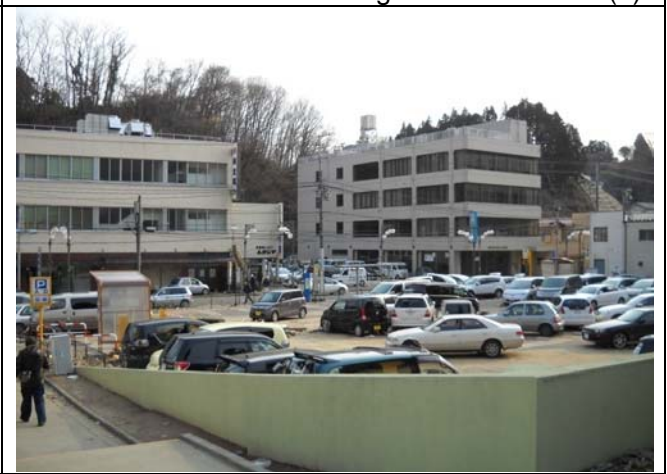
Photo 9: Kesen-numa City Municipal Building (2)
