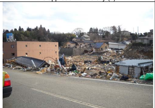
Photo 4: Damage was observed in the area lower than the route.
