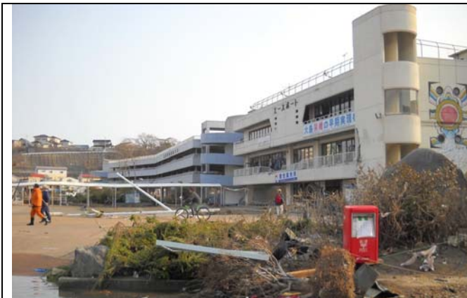
Photo 26: Sight-seeing Pier Building.
