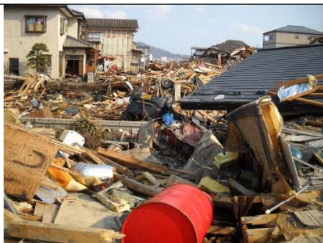
Photo 21: Damage in Kesen-numa City (4)
