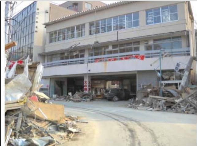
Photo 31: Overall view of the fire station building, no structural damage.
