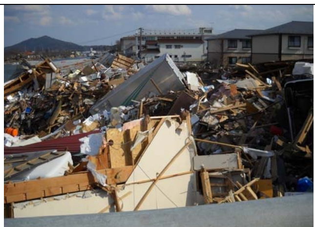
Photo 12: Damage of houses on both sides of the river (2)
