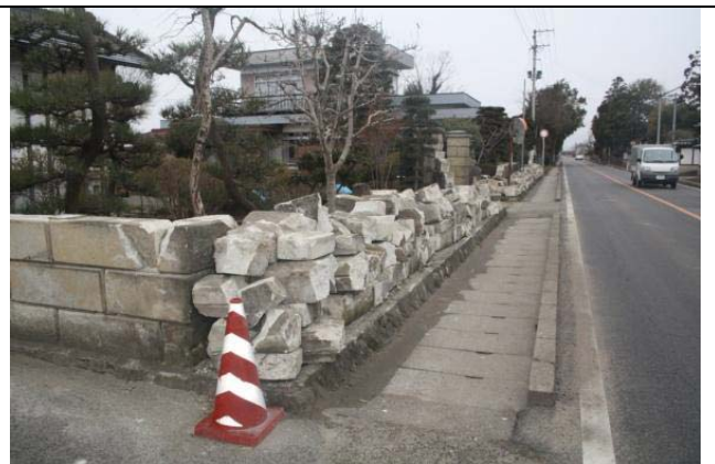
Photo 5: Fall of masonry walls
