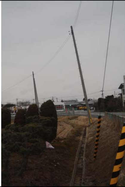
Photo 13: Tilting of utility poles
