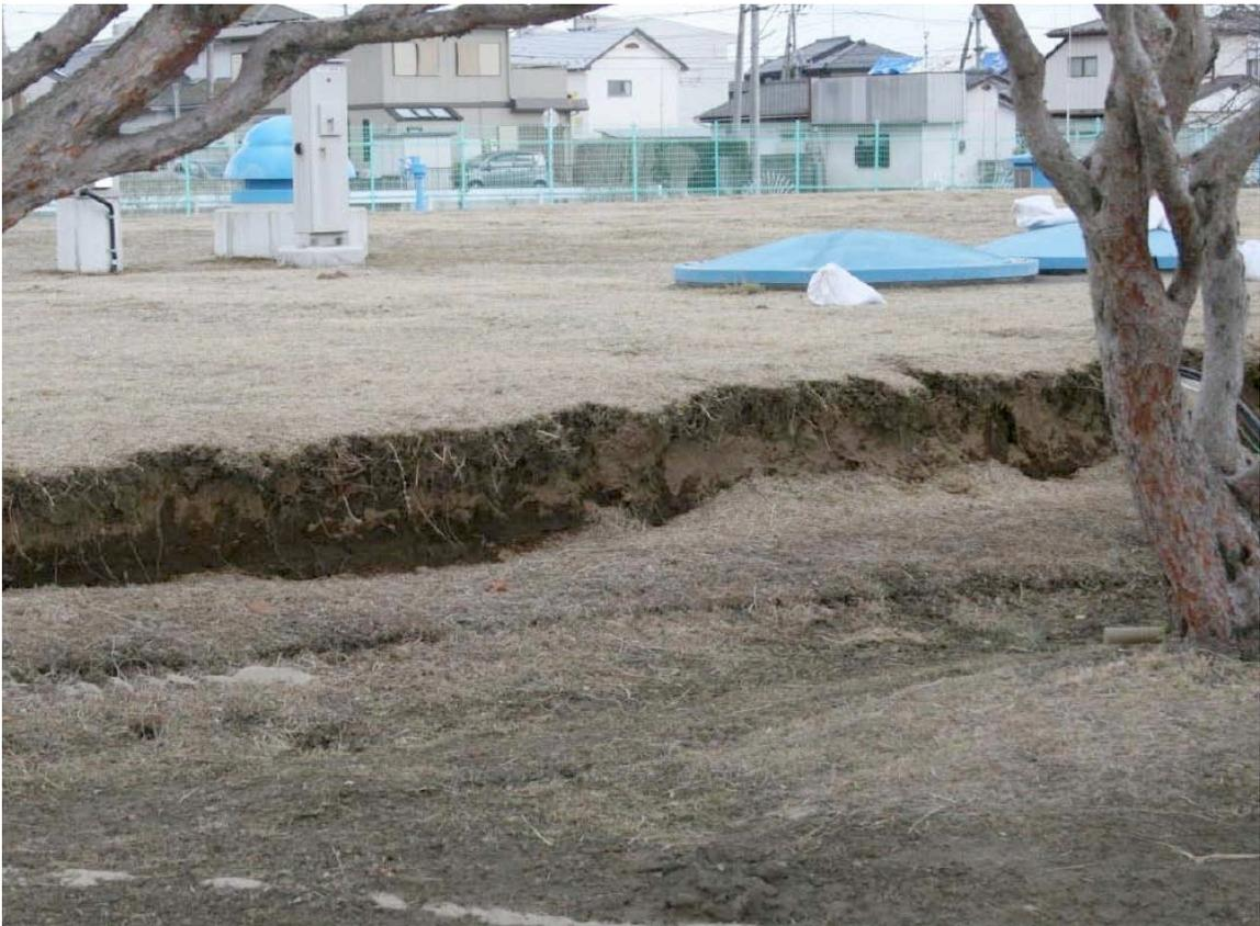
*Figure 3-31. Ground Deformation, Abuta WTP, Ishinomaki City*
