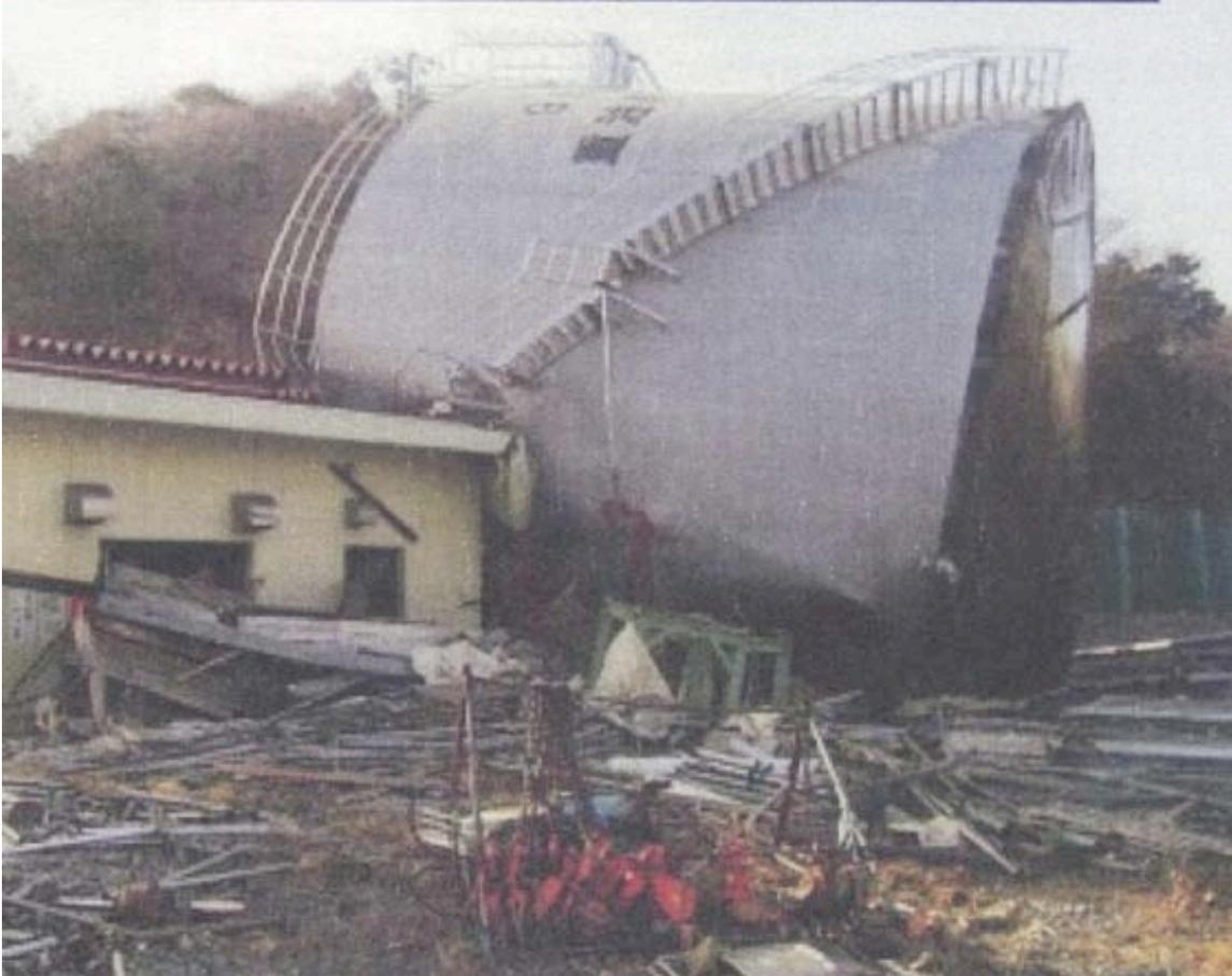
*Figure 4-67. Oil Tank for Unit 1 (Non Safety Related) – Onegawa*
