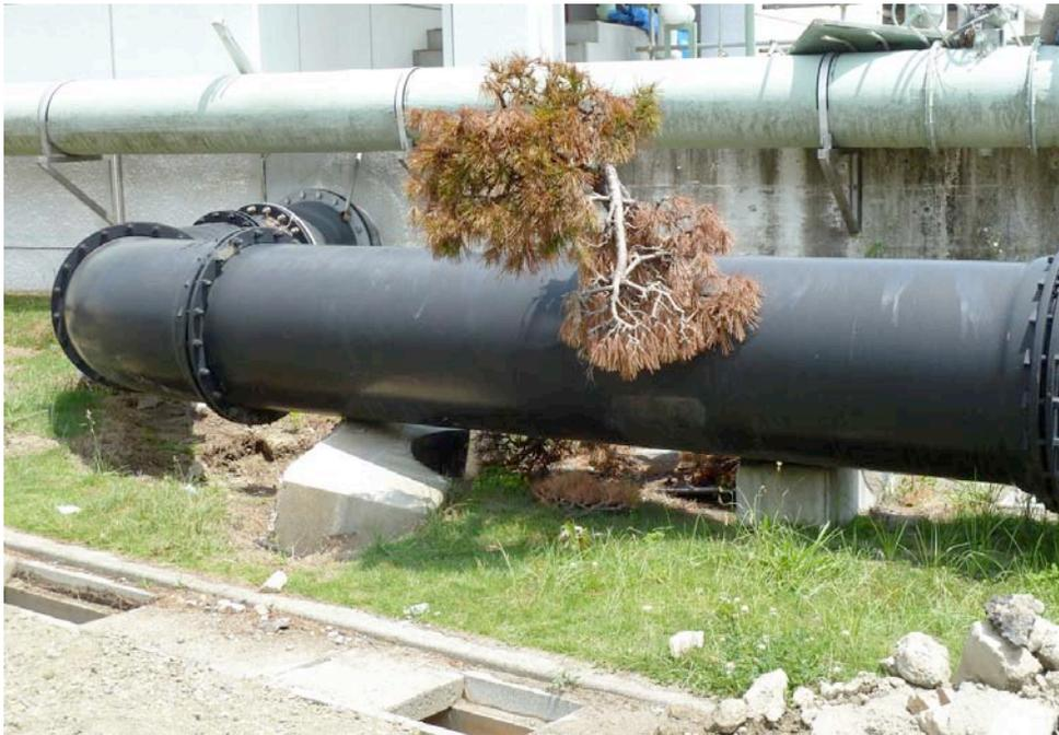
*Figure 3-49. Movement of Pipe Concrete Saddle Supports due to Tsunami Velocity Effects*
