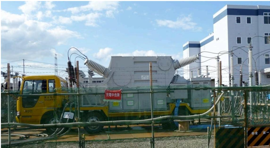
*Figure 4-36. Portable Transformer at Tagajyo Substation, June 14, 2011*
