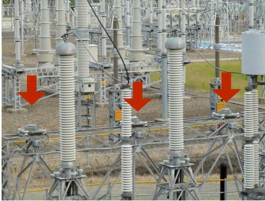
*Figure 4-46. 275 kV CVT Damage, Sendai Substation*
