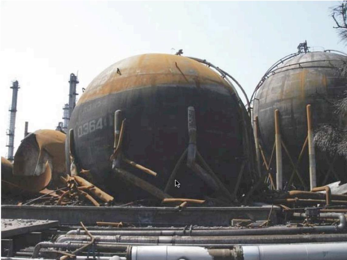
*Figure 3-56. Collapsed tank, after fire*
