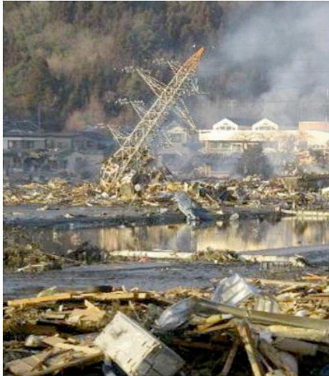
*Figure 4-62. Collapsed Transmission Tower – Tsunami Debris*
