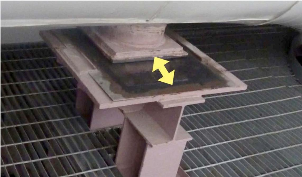
*Figure 4-27. Sliding Movement on pipe Support*
