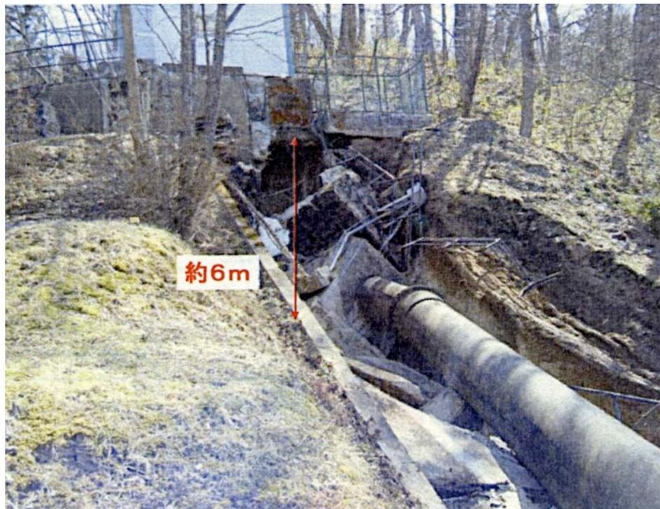
*Figure 4-9 Damaged Penstock and Forebay – Tohoku EPCo*
