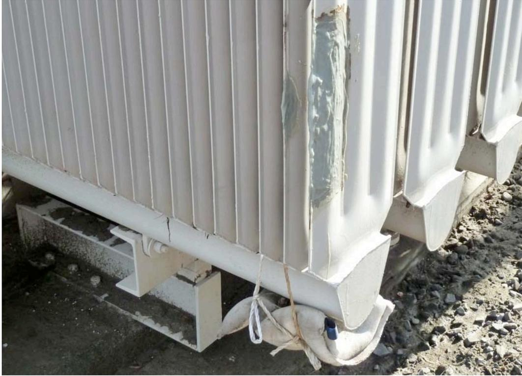
*Figure 4-40. Transformer Radiator Damage at Tagajyo Substation*
