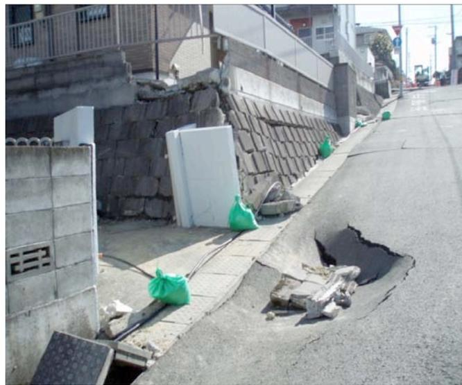
Figure 3-22. Damage to Road – Hillside Area, Nakayama, Sendai
