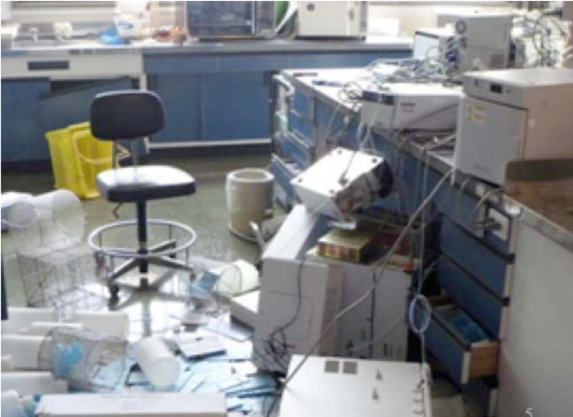
Figure 3-14. Unanchored Laboratory Equipment Toppled, Fukuoka WTP
