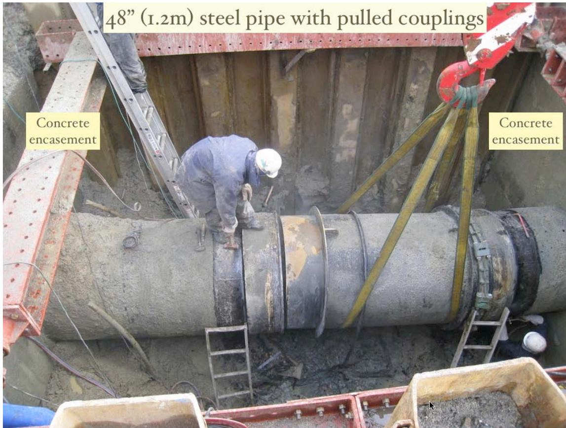
Figure 3-9. Pipe Under Repair, (48", 1200 mm Diameter Pipe) (Kuwata)
