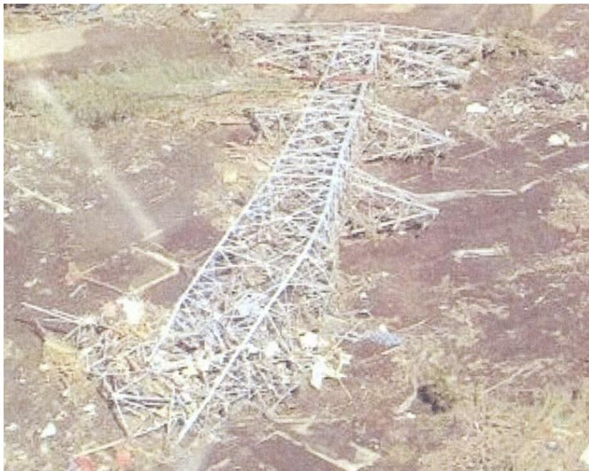
*Figure 4-61. Collapsed Transmission Tower – Tsunami Debris*
