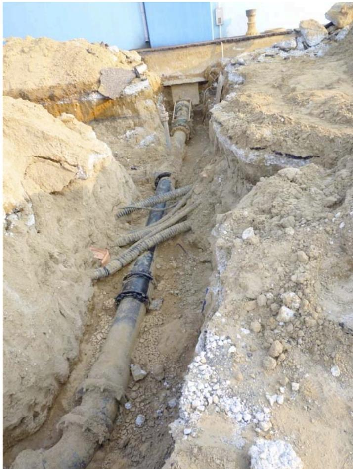
*Figure 3-40. Damaged 300 mm Pipe*
