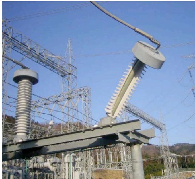
*Figure 4-81. Damaged 154 kV Instrument Transformer*
