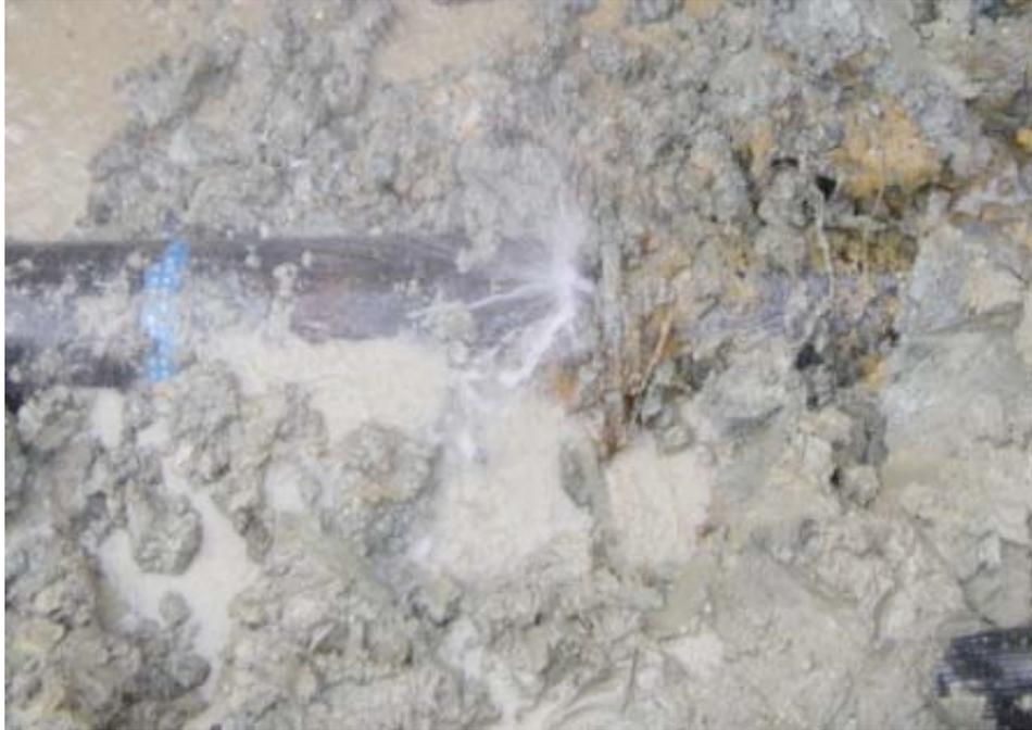
*Figure 3-18. Leaking Pipe, Sendai*
