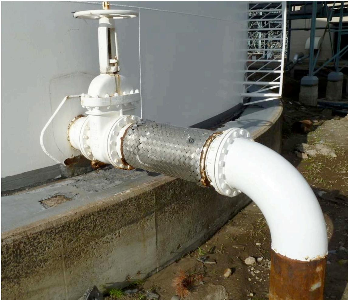
*Figure 4-17. Shin Sendai Power Station – Water Tank 1, Scour*
