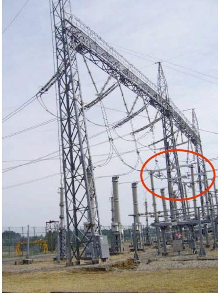
*Figure 4-82. Damaged 275 kV Disconnect Switch*
