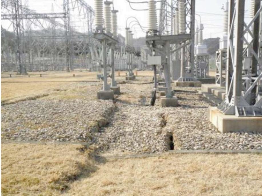
*Figure 4-80. Ground Deformations Near a 154 kV Pothead*
