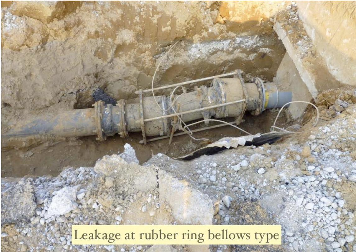
*Figure 3-41. Leakage at the Flexible Joint Next to the Tank (Not Flexible Enough)*
