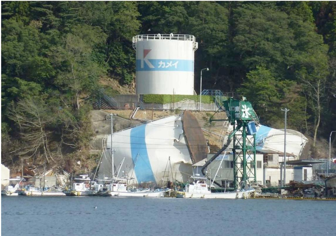
*Figure 2-12. Two Floated Tanks, One OK Tank (Onegawa)*
