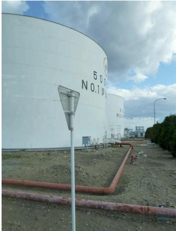
*Figure 2-14. Two Water Tanks that were Inundated*
