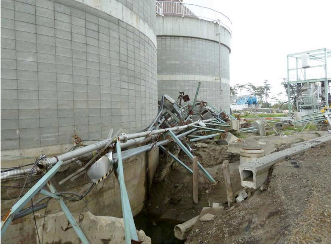
*Figure 3-47. Damage to Pipe Racks Next to Digesters, due to Erosion*
