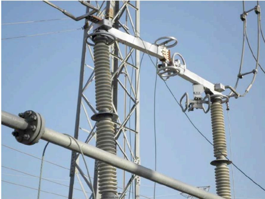
*Figure 4-83. Damaged 275 kV Disconnect Switch*
