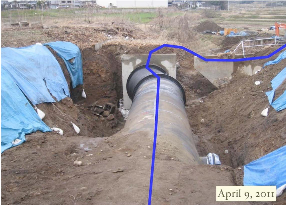
*Figure 3-8. Repaired Pipe, Point 1 (96", 2400 mm Diameter Pipe)*
