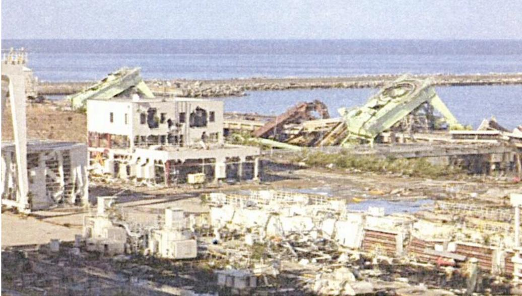
*Figure 4-32. Haramachi Power Station – Damaged Coal Unloader*
