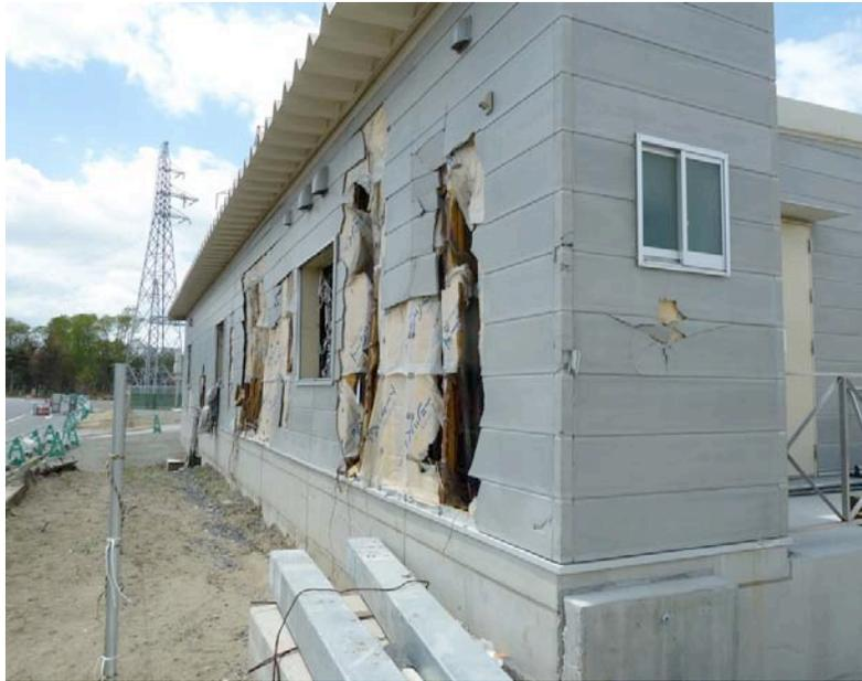
*Figure 4-55. Control Building Failed due to Inundation, Ishinomaki*
