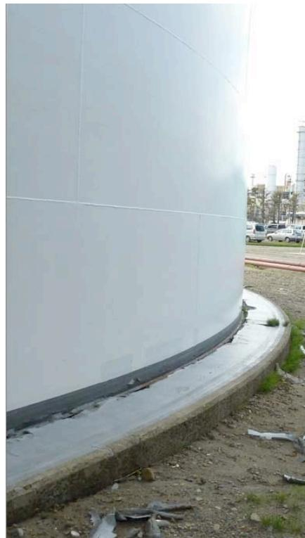
*Figure 2-15. Tank 1, Showing Evidence of Distress / Uplift*
