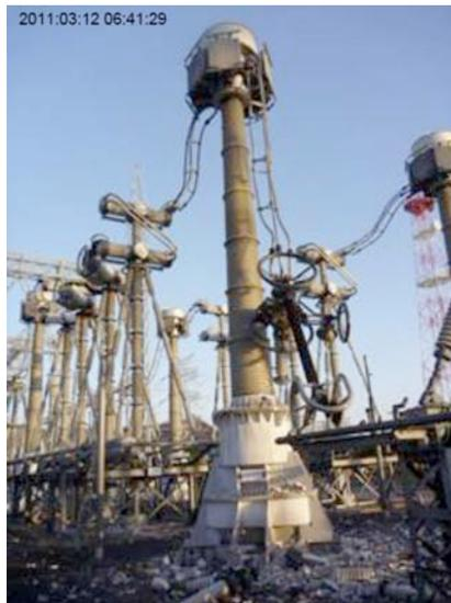
*Figure 4-87. 275 kV Current Transformers and Live Tank Circuit Breakers*
