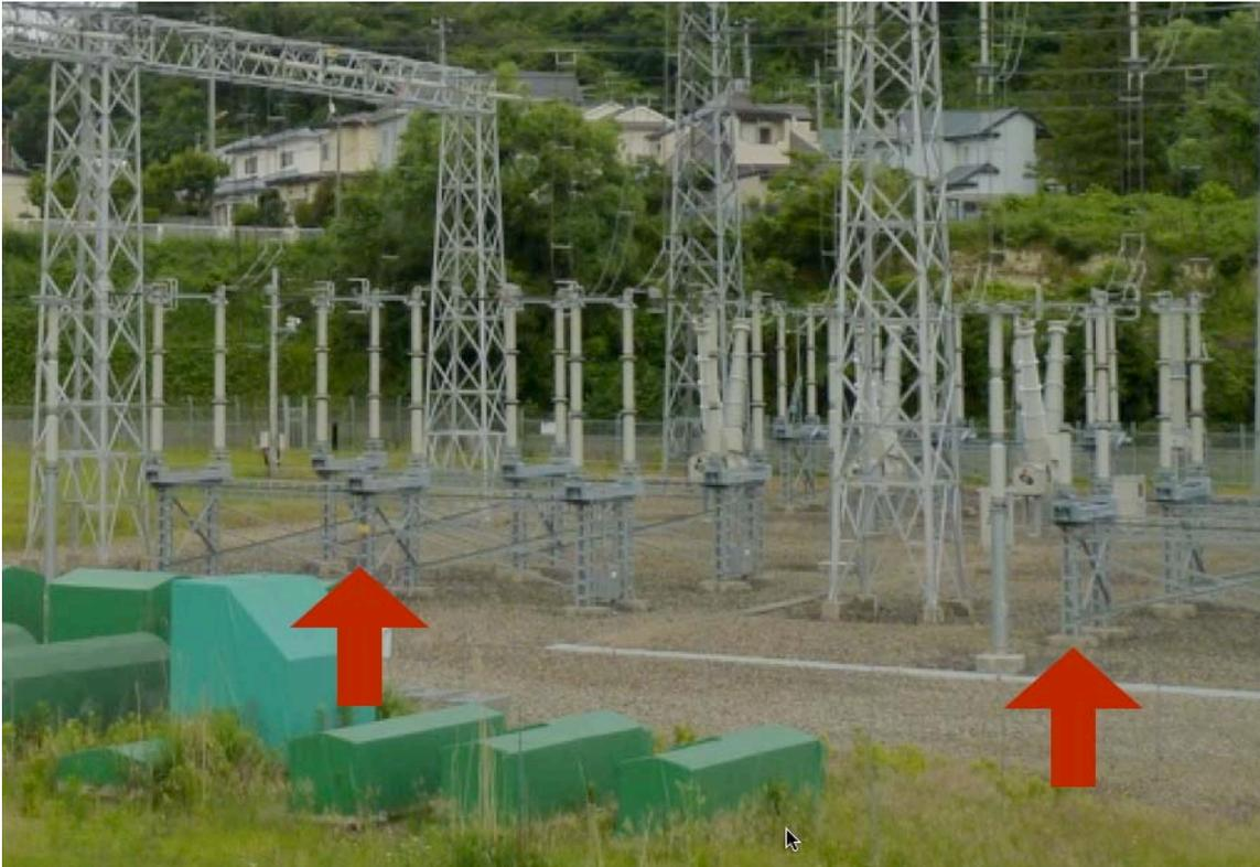
*Figure 4-48. 275 kV Disconnect Switch Damage, Sendai Substation*
