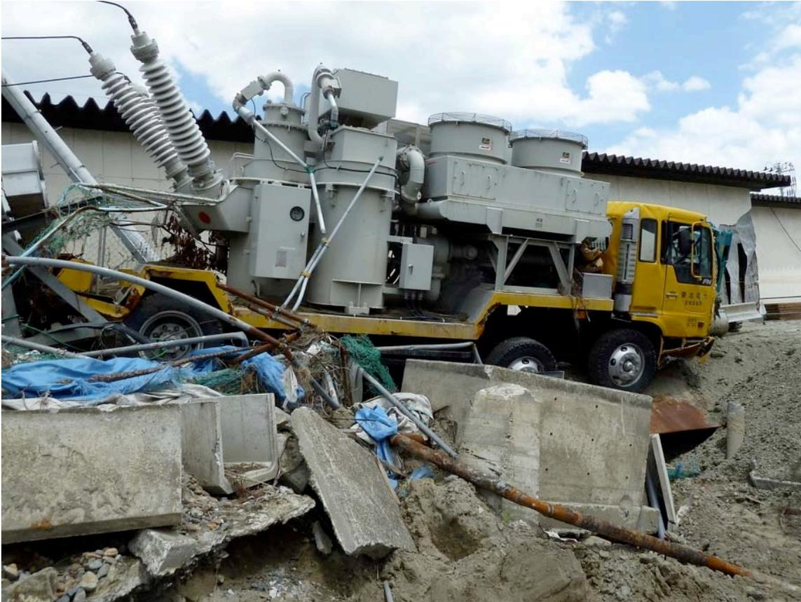
*Figure 4-57. Portable 66 kV Transformer Damaged by Inundation, Ishinomaki*
