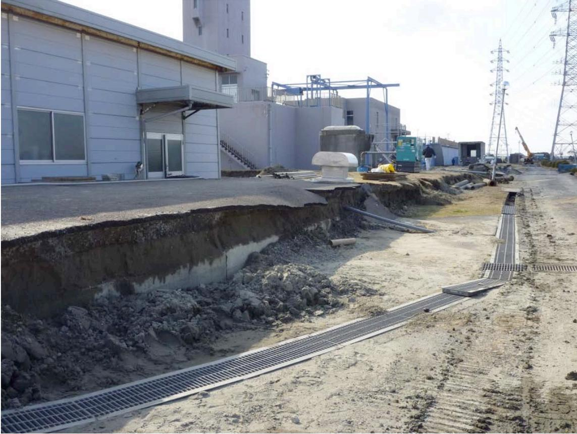
*Figure 3-36. Wanagawa Water Treatment Plant, Uplifted Utility Corridor*
