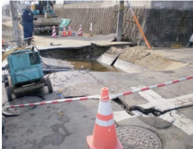
Figure 3-23. Damage to Road – Hillside Area, Nakayama, Sendai
