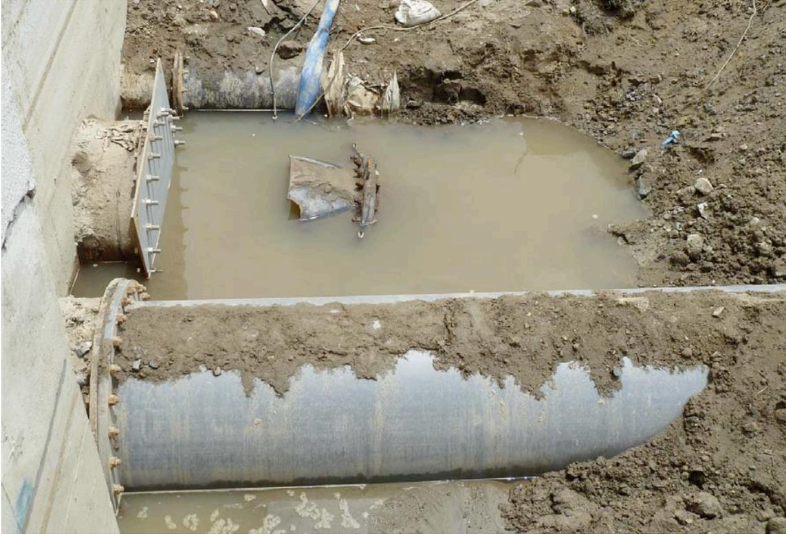
*Figure 3-46. Three Large Diameter Pipes Damaged due to Tsunami-Caused Erosion*
