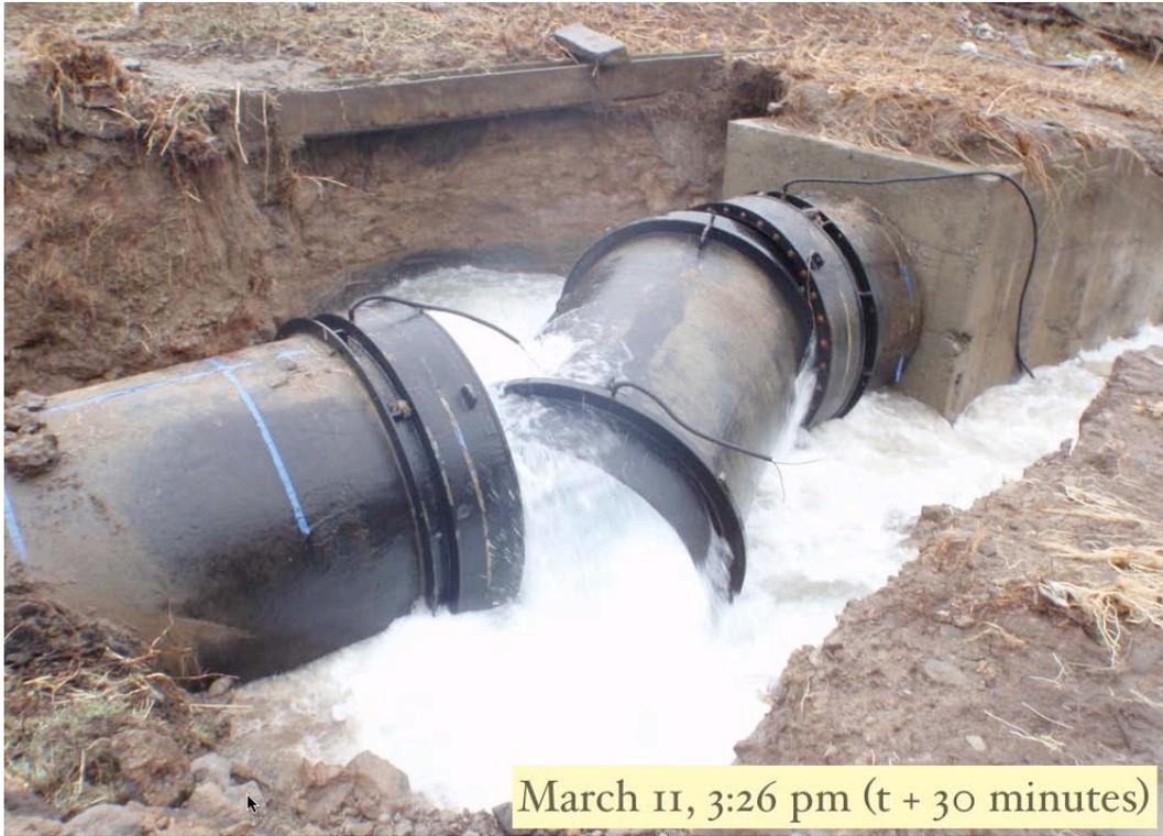
Figure 3-4. Damage Point 1, (96", 2400 mm Diameter Pipe)
