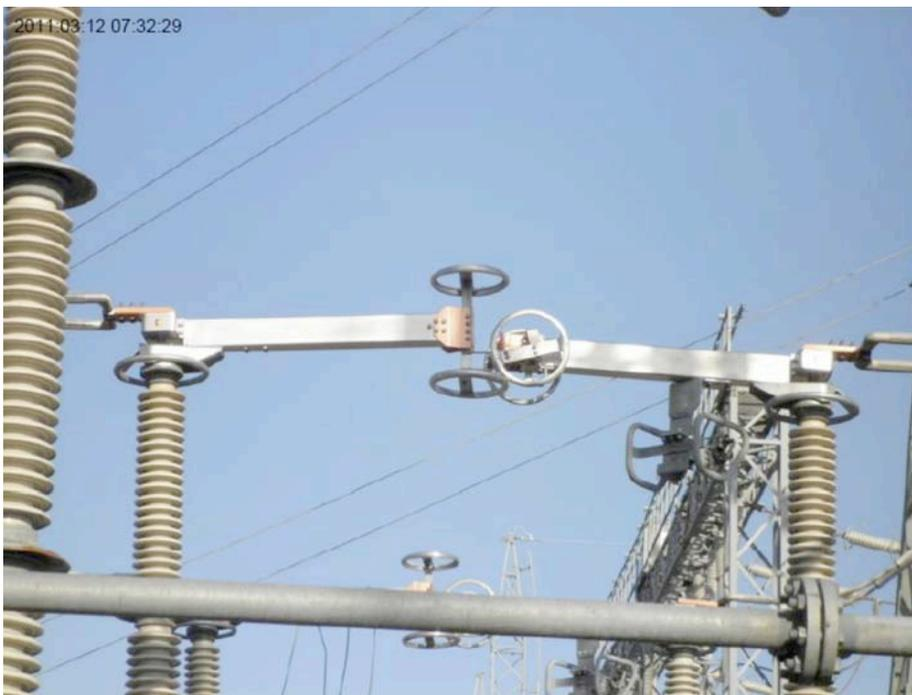
*Figure 4-84. Damaged 275 kV Disconnect Switch*
