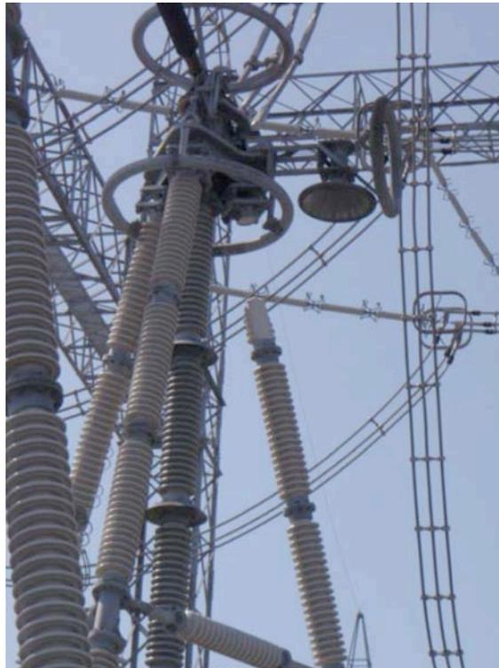
*Figure 4-90. 500 kV Disconnect Switch*
