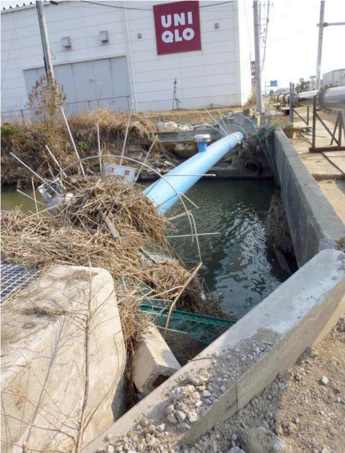
*Figure 3-43. Failed Water Pipe, Kamisu City (Temporary Pipe seen on right)*
