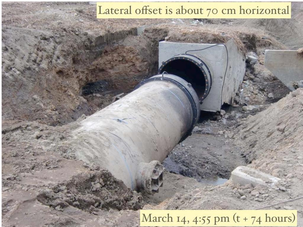
*Figure 3-6. Offset at Slip Joint*
