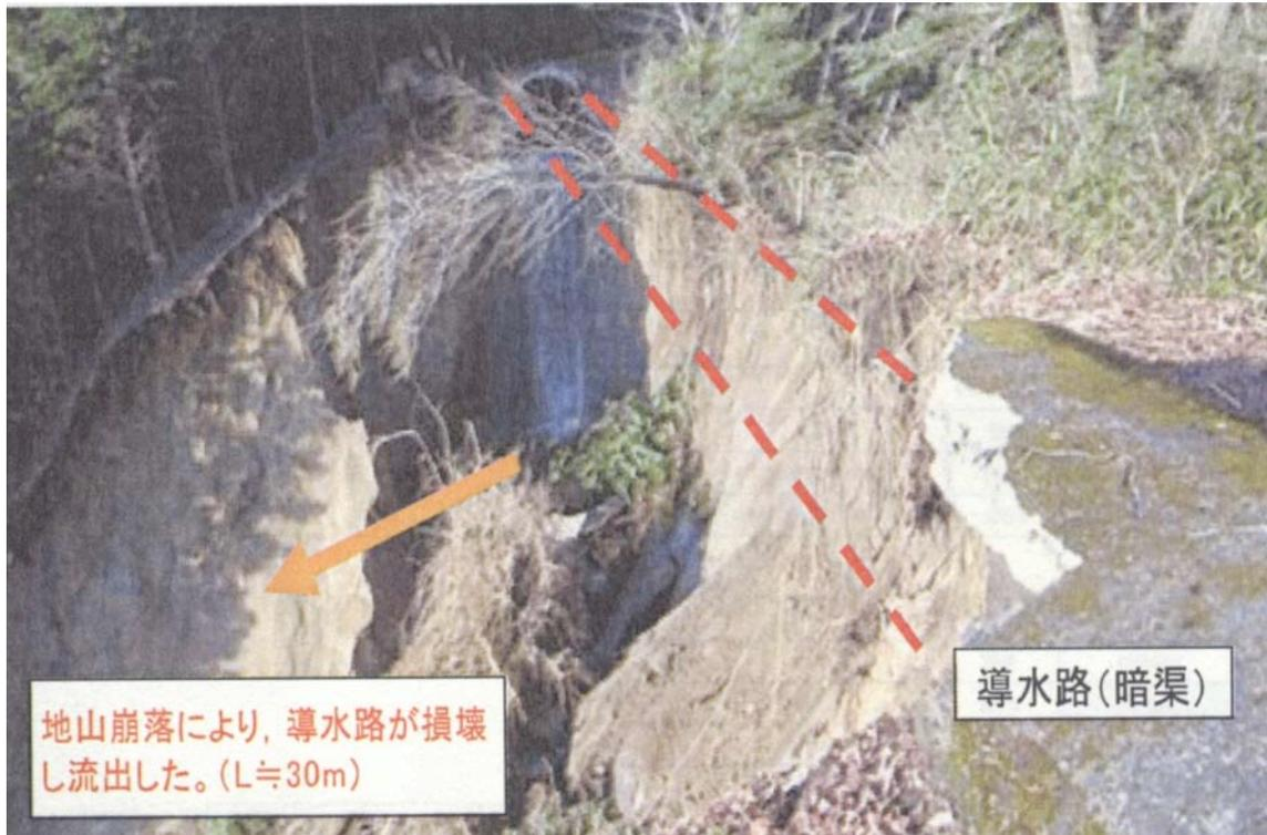
Figure 4-10. Damaged Headrace – Tohoku EPCo
