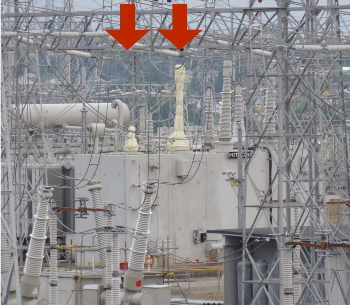
*Figure 4-45. 275 kV Bushing Damage, Sendai Substation*
