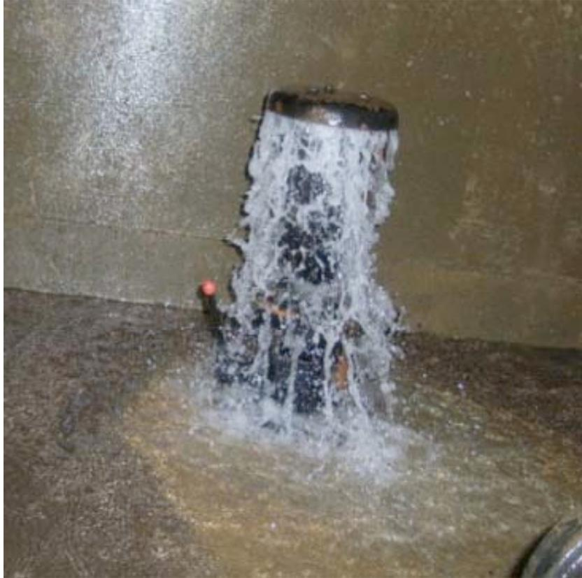
*Figure 3-20. Leaking Air Valve, Sendai*
