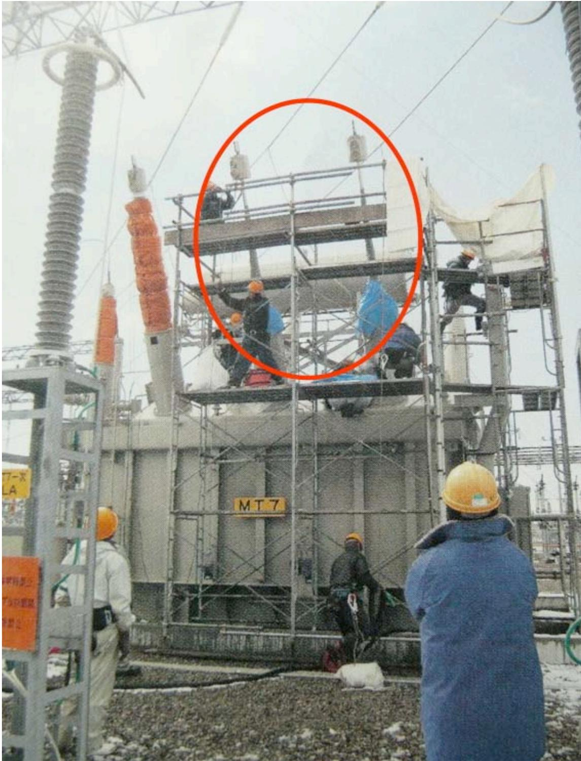
*Figure 4-53. Bushing Replacements on Transformer*
