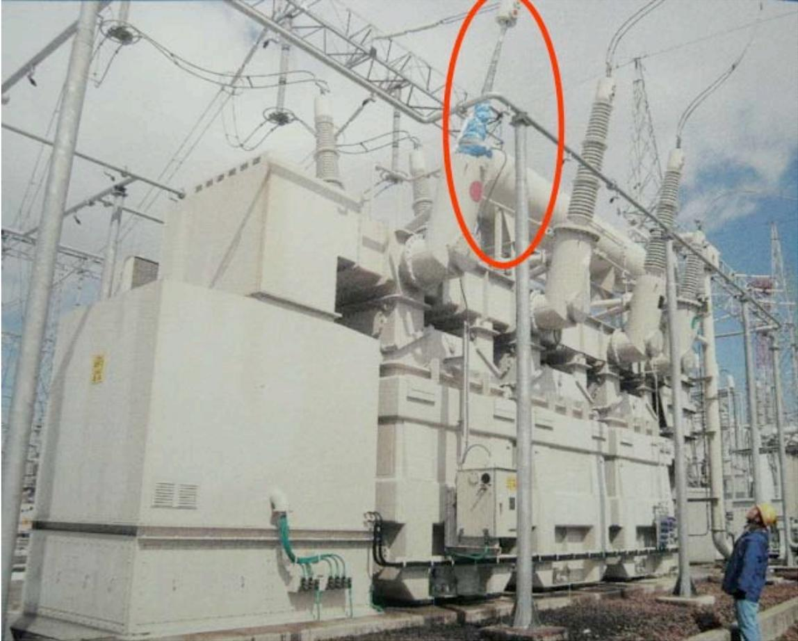
*Figure 4-54. Bushing Failure on Transformer*
