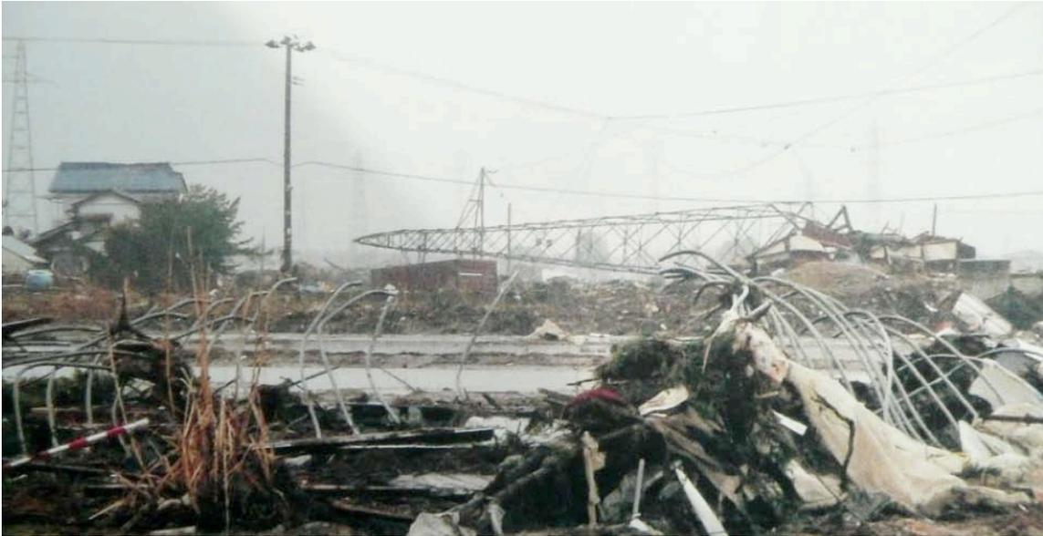
*Figure 4-60. Collapsed Transmission Tower – Tsunami Debris*
