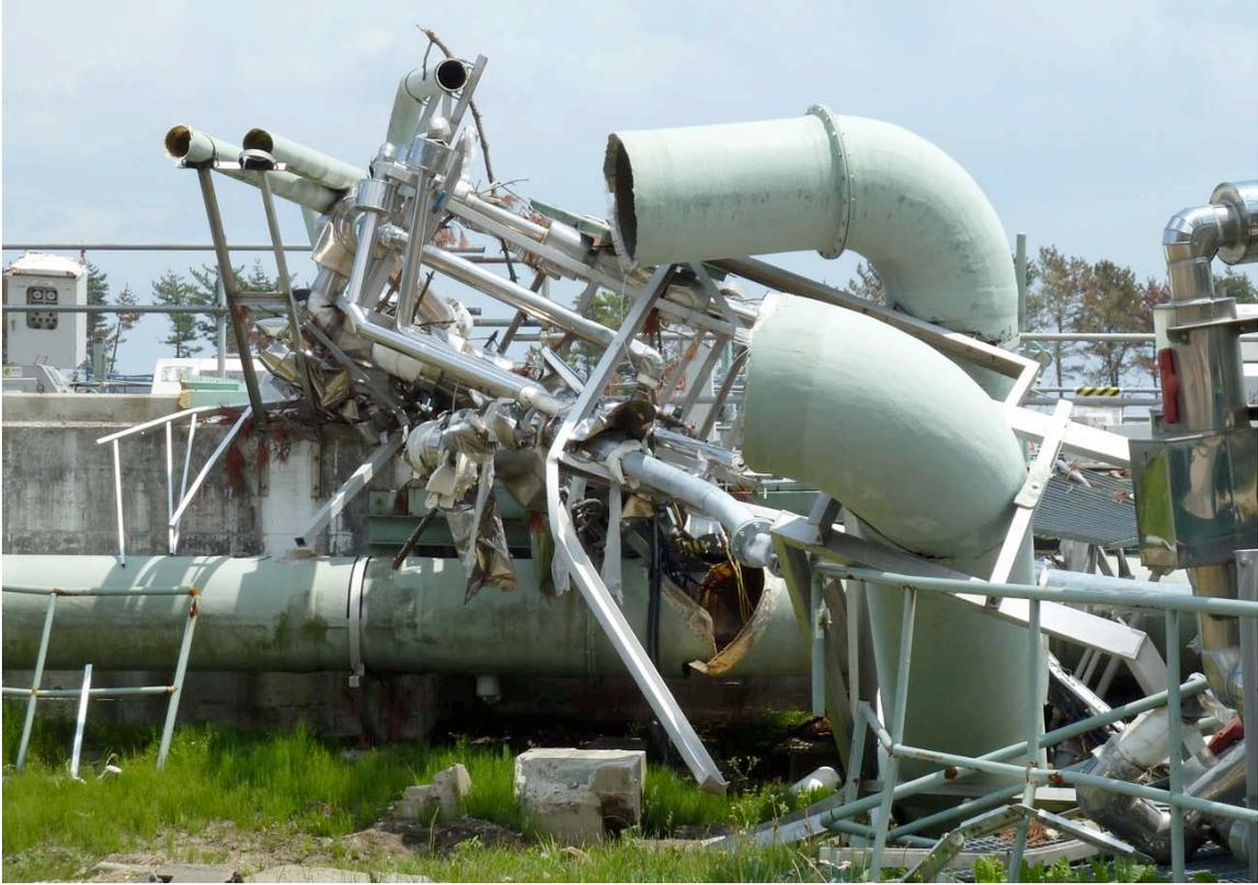
*Figure 3-48. Damage to Air Pipes due to Tsunami Velocity Effects*
