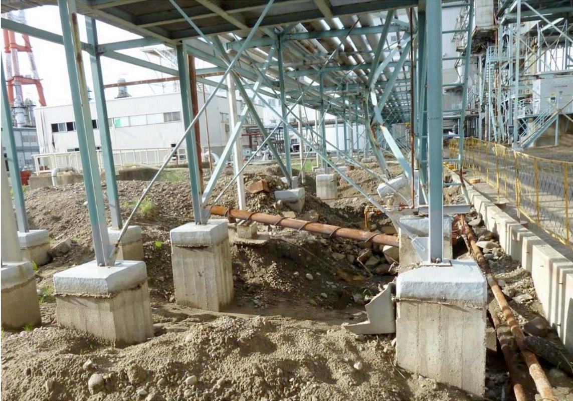
*Figure 4-18. Shin Sendai Power Station – Pipe Chase, Scour, Bracing Damage*
