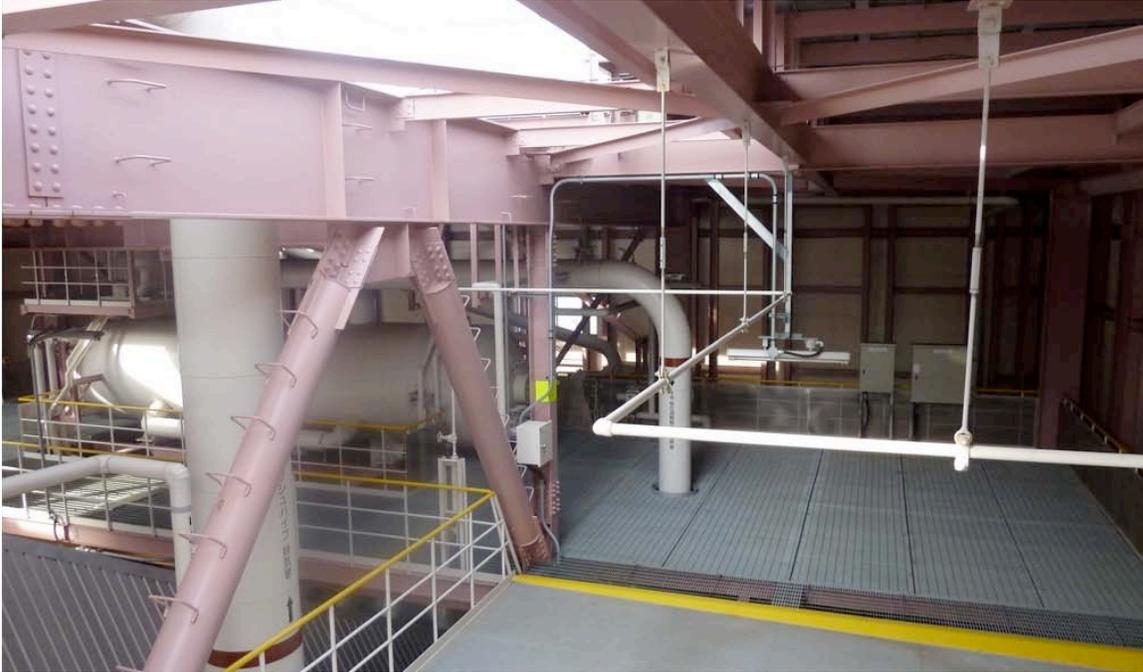
*Figure 4-28. Small Bore Pipe with Rod Hanger Supports had Good Performance*
