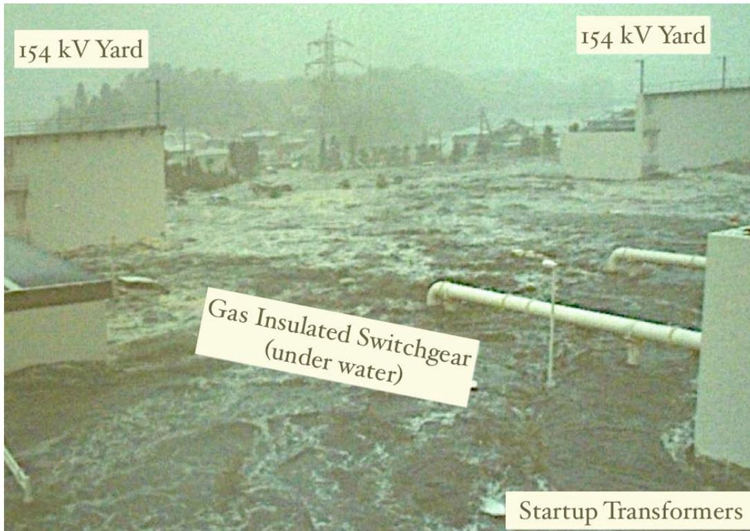
Figure 4-22. Tsunami Inundating the Switchyard
