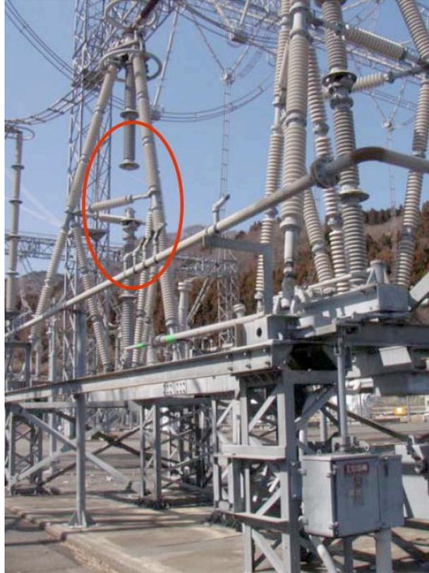
*Figure 4-89. 500 kV Disconnect Switch*
