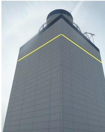
*Figure 4-29. Enclosure Around Chimney Stack. Yellow Lines Indicate Lateral Braces for Chimney Within*
