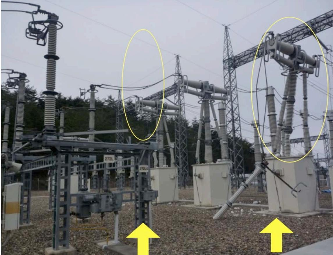
*Figure 4-50. 275 kV Live Tank Circuit Breaker*
