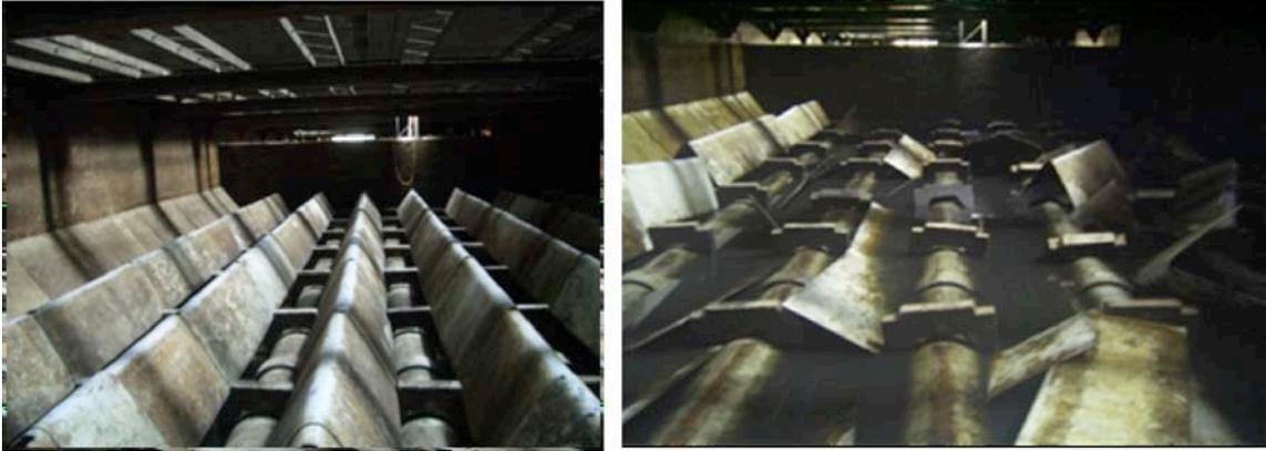
*Figure 3-12. Baffle Boards, Moniwa WTP (Left: before; Right: after)*
