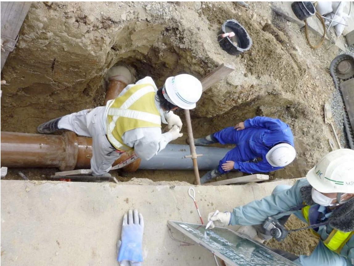
*Figure 3-19. Typical Distribution Pipe Repair being made in Sendai (Kuwata)*
