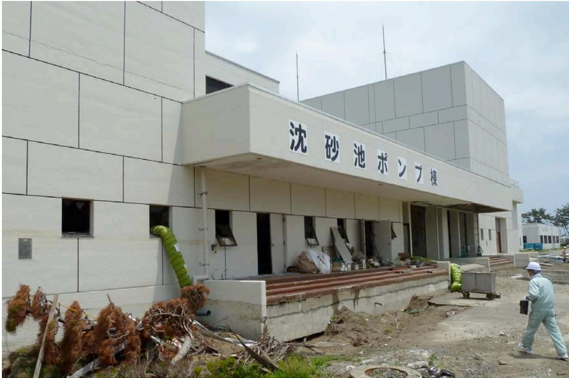
*Figure 3-45. Pump Station – Erosion Impacts due to Tsunami*
