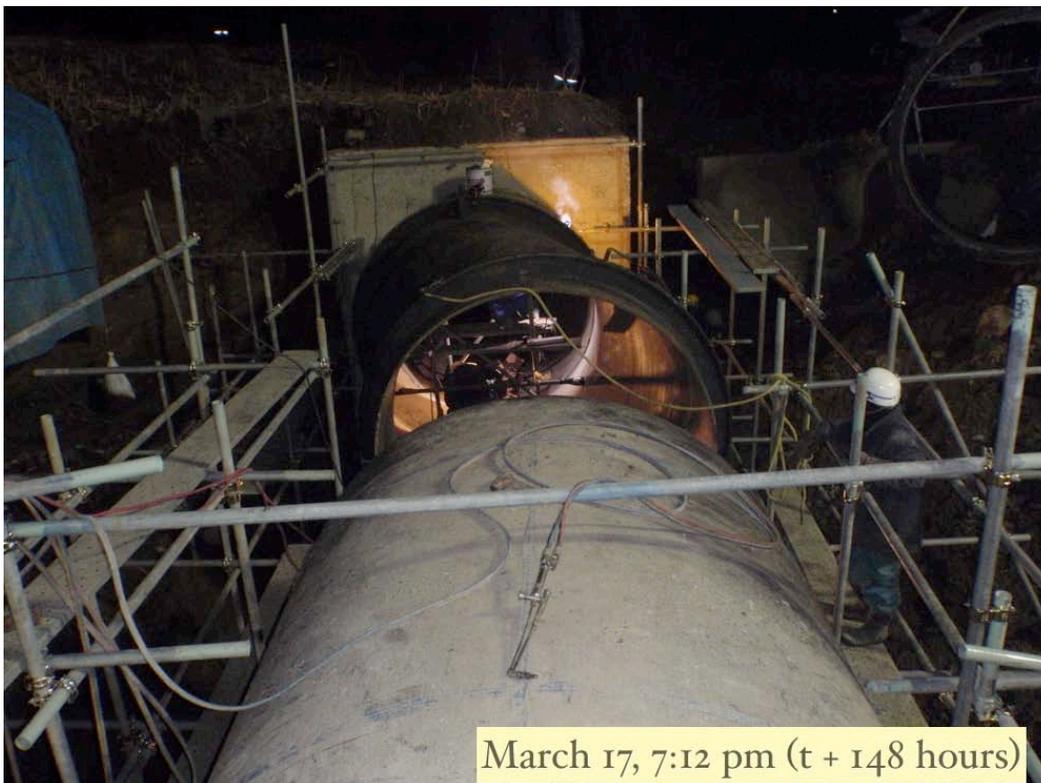
*Figure 3-7. Repair Efforts, Night time, (96", 2400 mm Diameter Pipe)*
