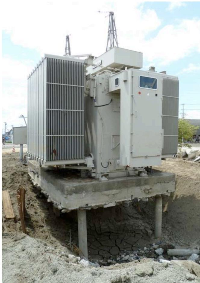
*Figure 4-56. Transformer Undermined by Scour, Ishinomaki*
