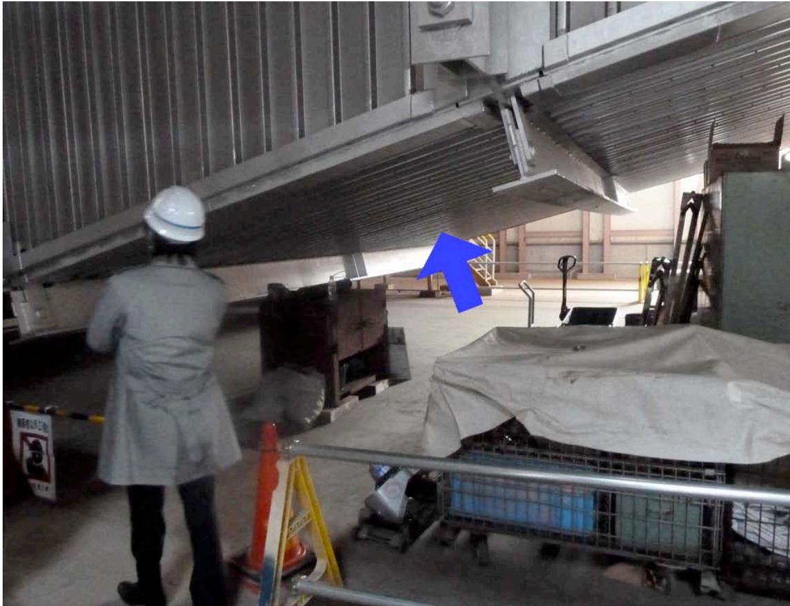
*Figure 4-31. Damage Location to Steam Generator Exhaust Manifold*
