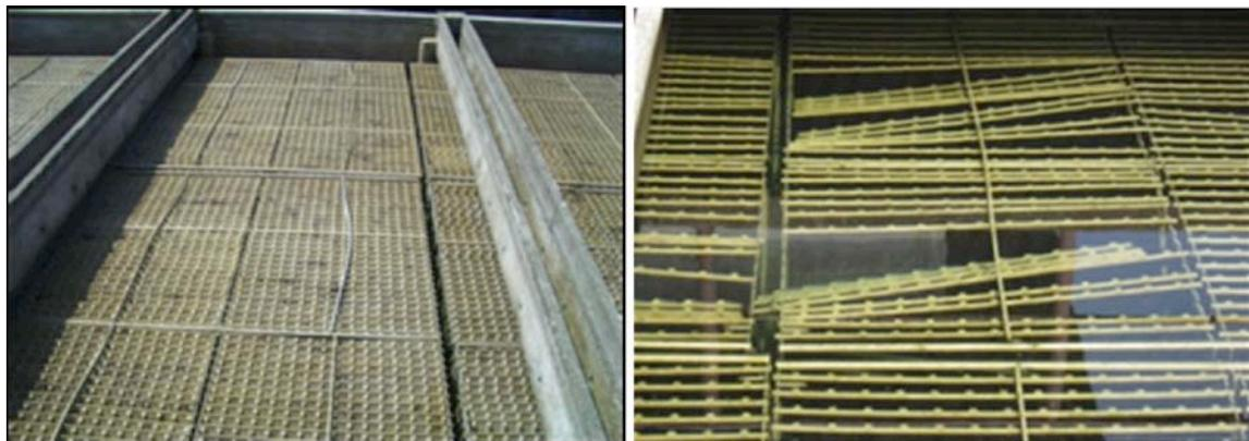
Figure 3-11. Inclined Basin Plates, Moniwa WTP (Left: before; Right: after)
