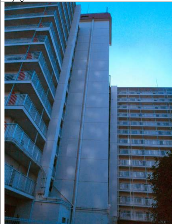
Photo 18: Expansion joint between two buildings (left on March 12, and right on March 16)
