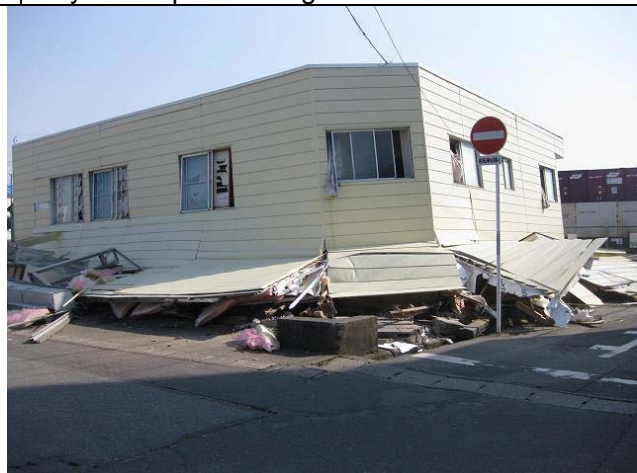
Photo 9: Collapse of a two-story house for combined use for shop and residence
