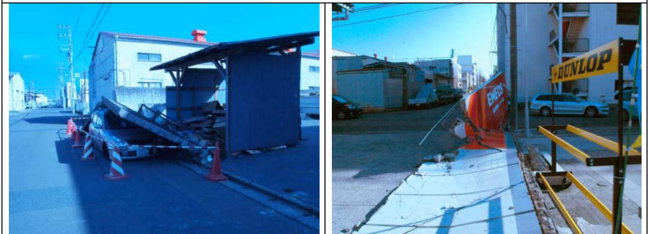
Photo 15: Overturned concrete block fences in Oroshi-machi, Wakabayashi-ku
