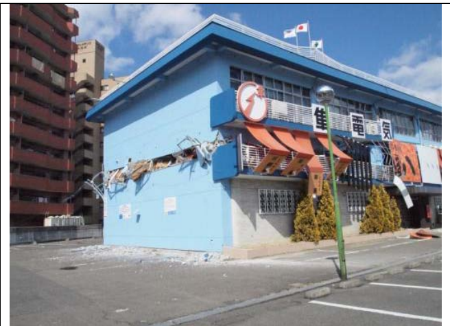
Photo 7: Collapse in the second story
