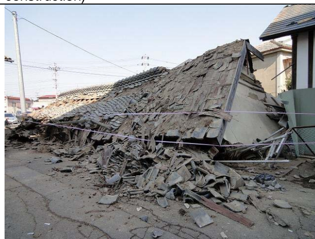
Fig. 7: Collapse of a Godown, adjacent to Ohsaki City Municipal Building
