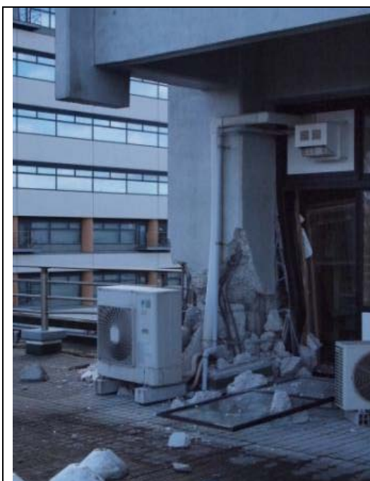
Photo 3: Damage of north-east corner column
