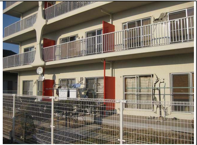
Photo 17: Shear failure of non-structural exterior walls
