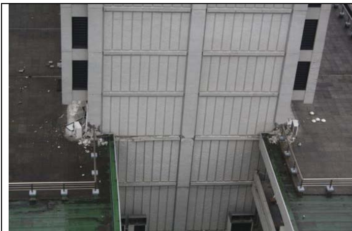
Photo 1: Damage of end walls from roof of the adjacent building
