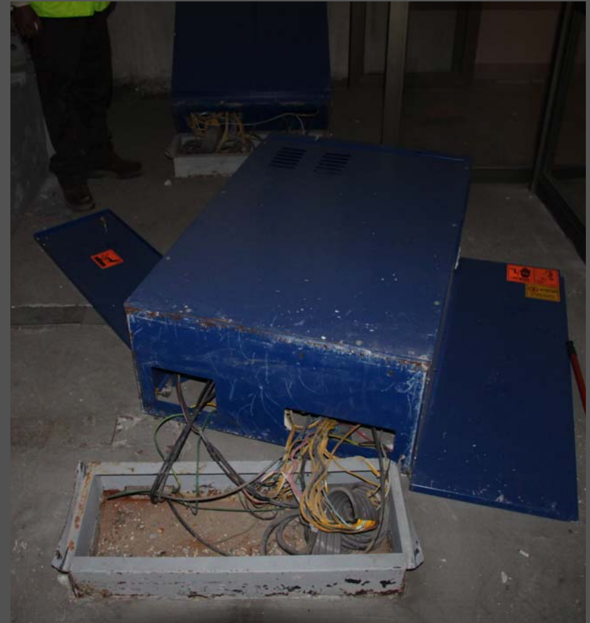
Overturned switch control panel
