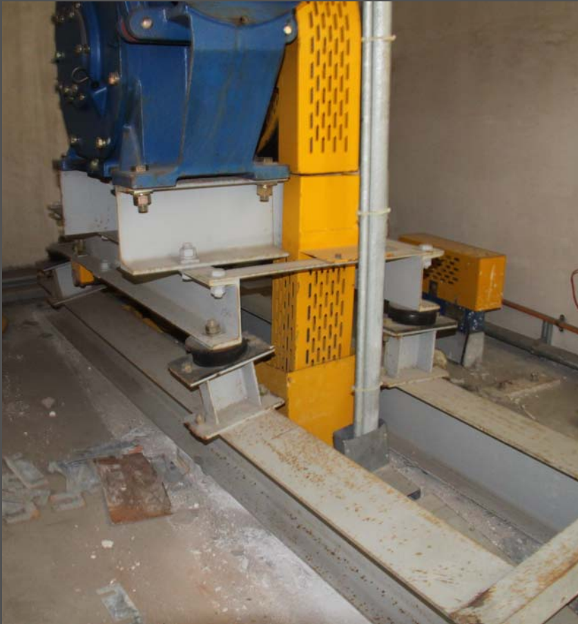
Nearly overturned elevator machine
