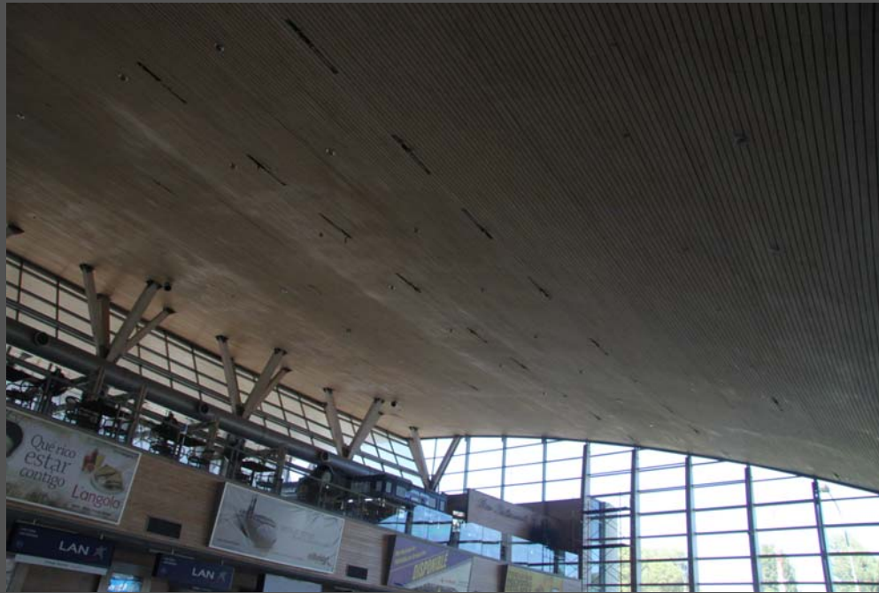
Overall view of wood ceiling
