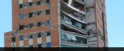
Foreground: collapsed older building with reinforced concrete beams and columns "confining" the masonry
