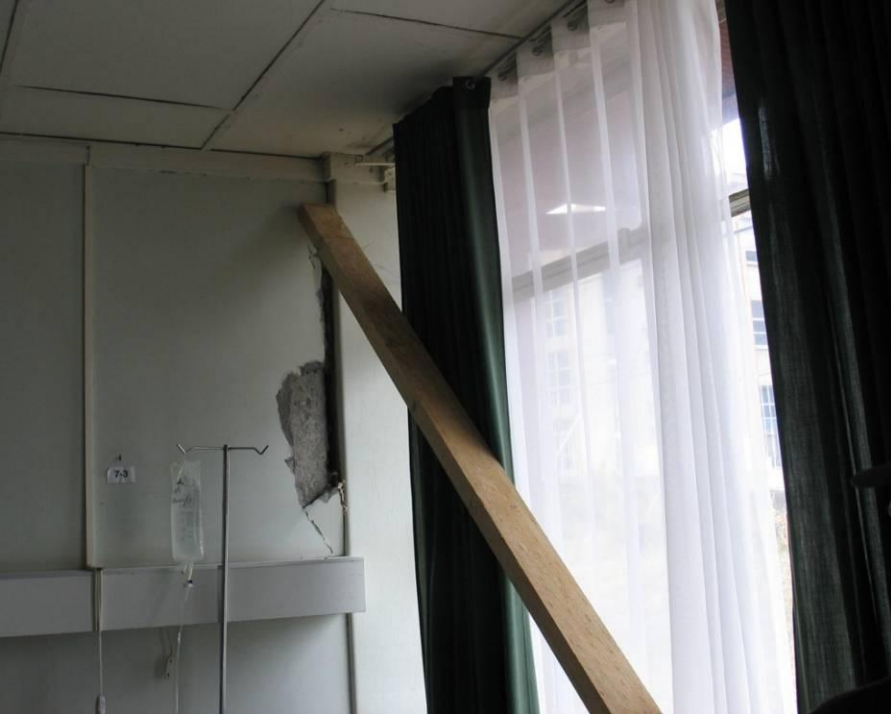
Temporary braces at loose precast partitions. Laja
