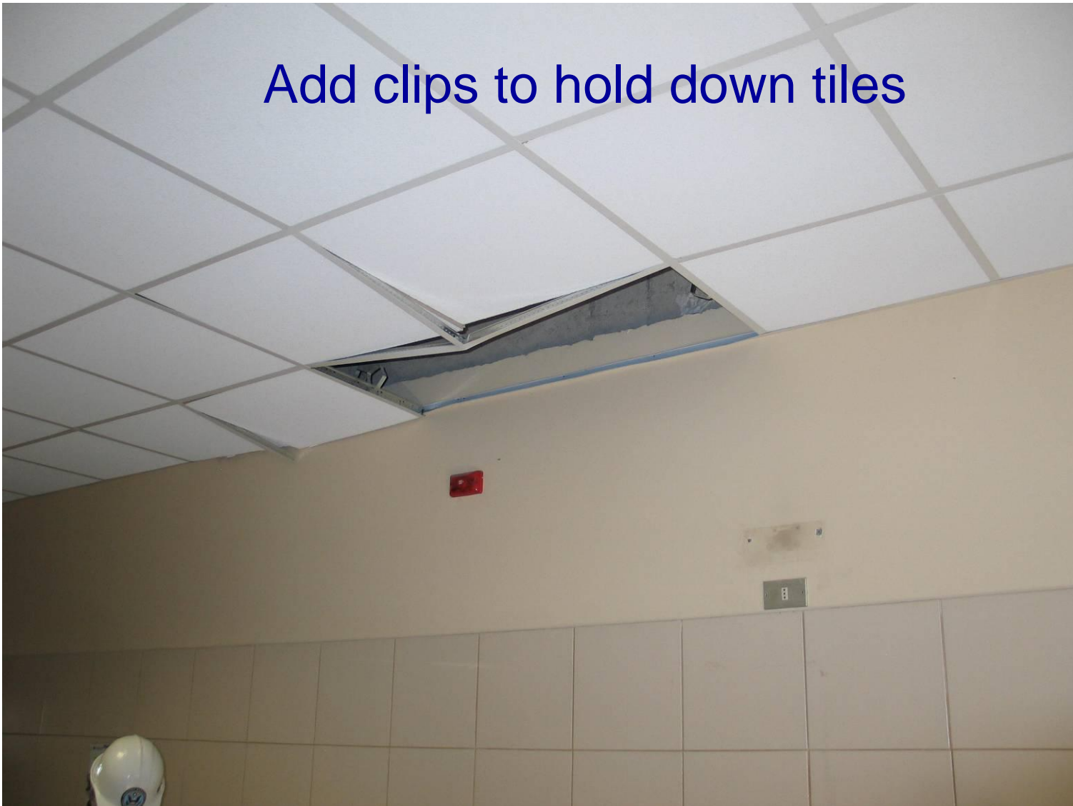
Fallen tile despite clips. Talca Hospital.
