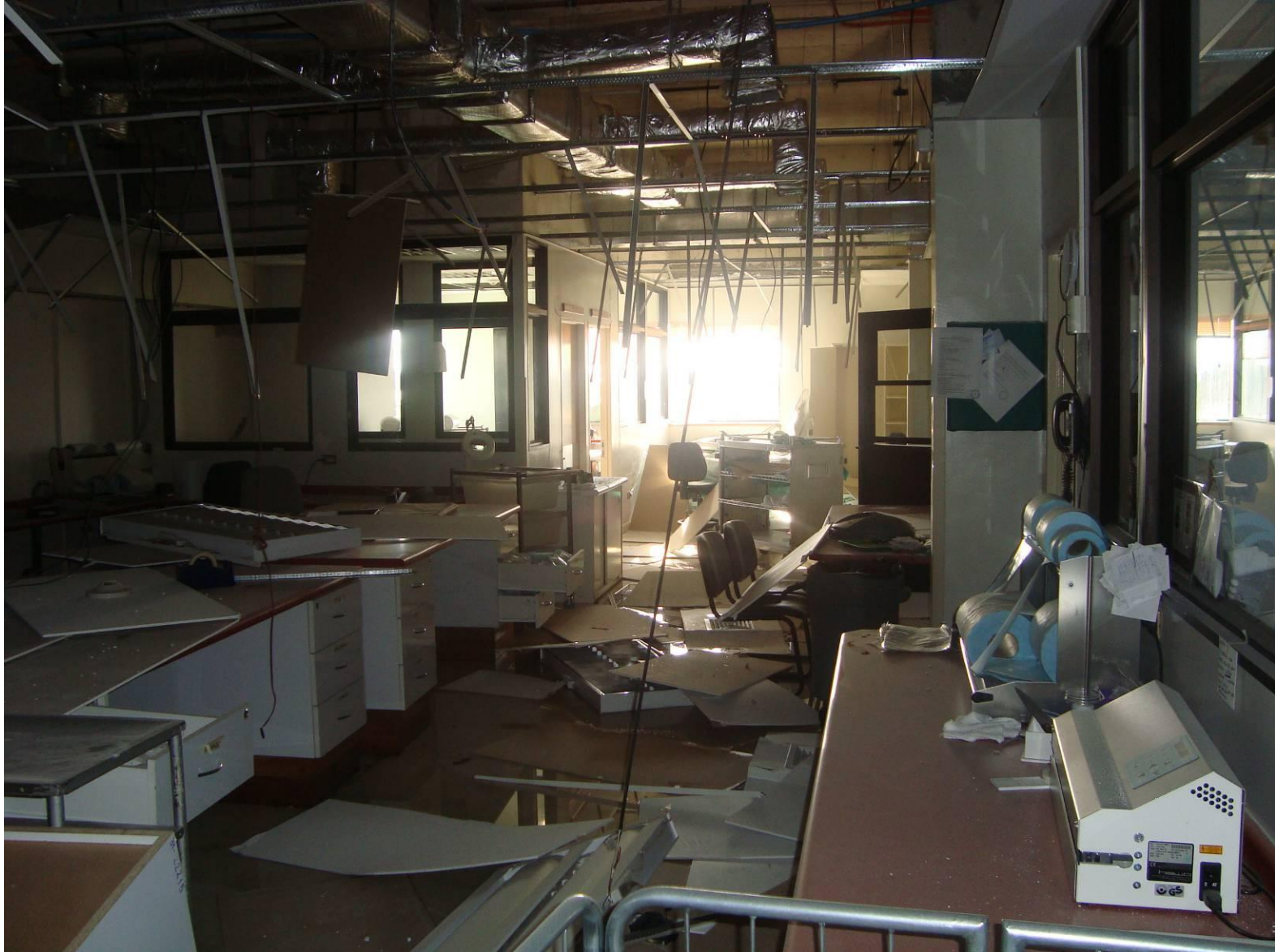
The morning after. Los Angeles Hospital. Note fallen light fixtures and mechanical registers, in addition to ceiling panels.
