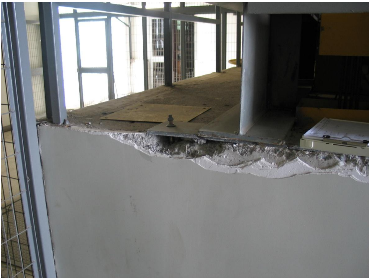
Anchor bolt failure of elevator generator set due to inadequate edge distance. Los Angeles Regional Public Hospital
