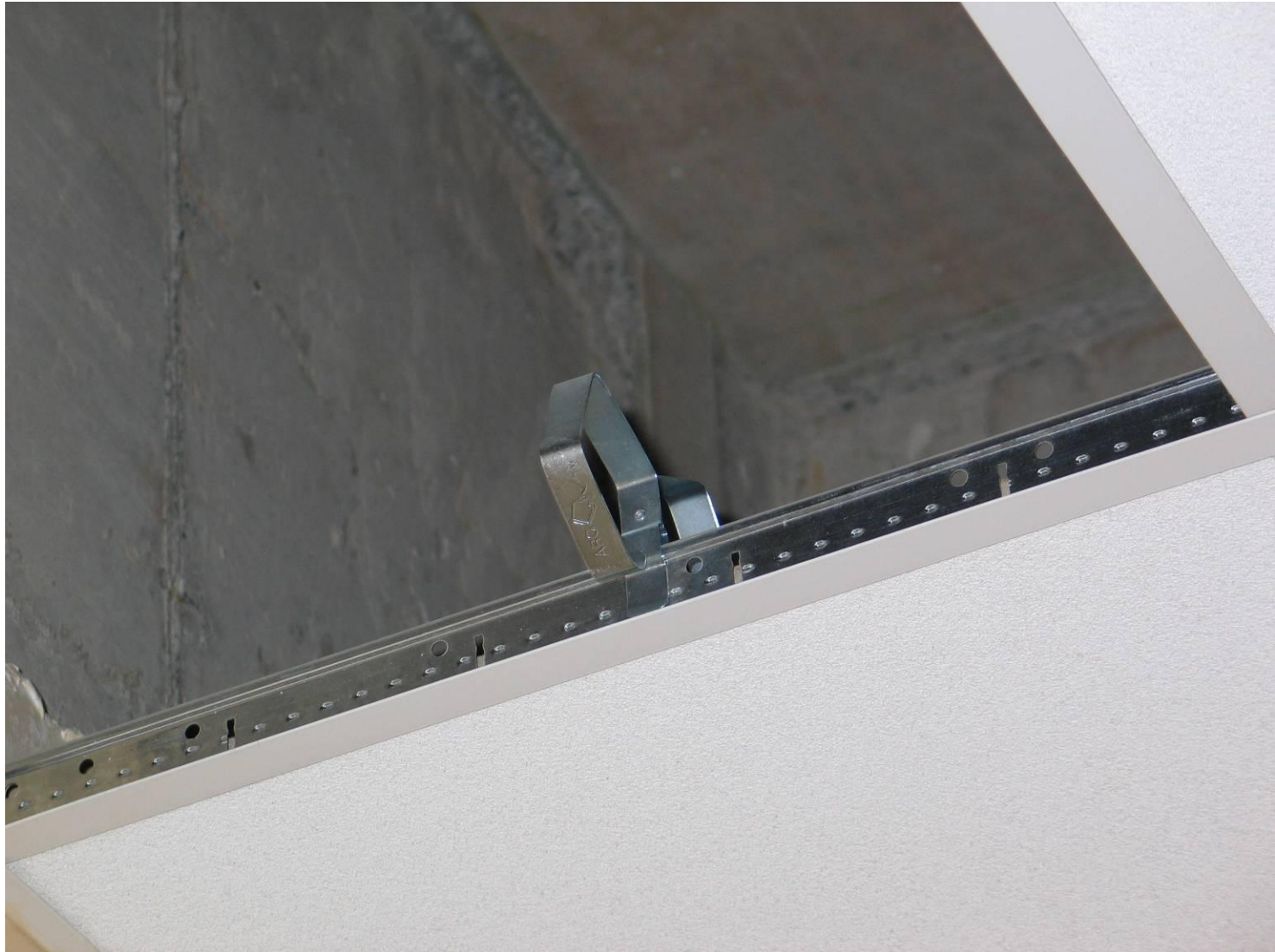
Close up of clips used at Talca Hospital in new building.
