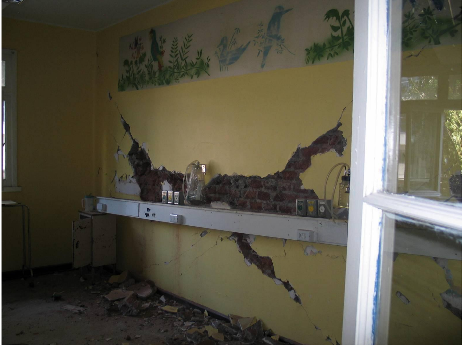
Cracked and spalled infill in patient room. Felix Bulnes (Santiago)
