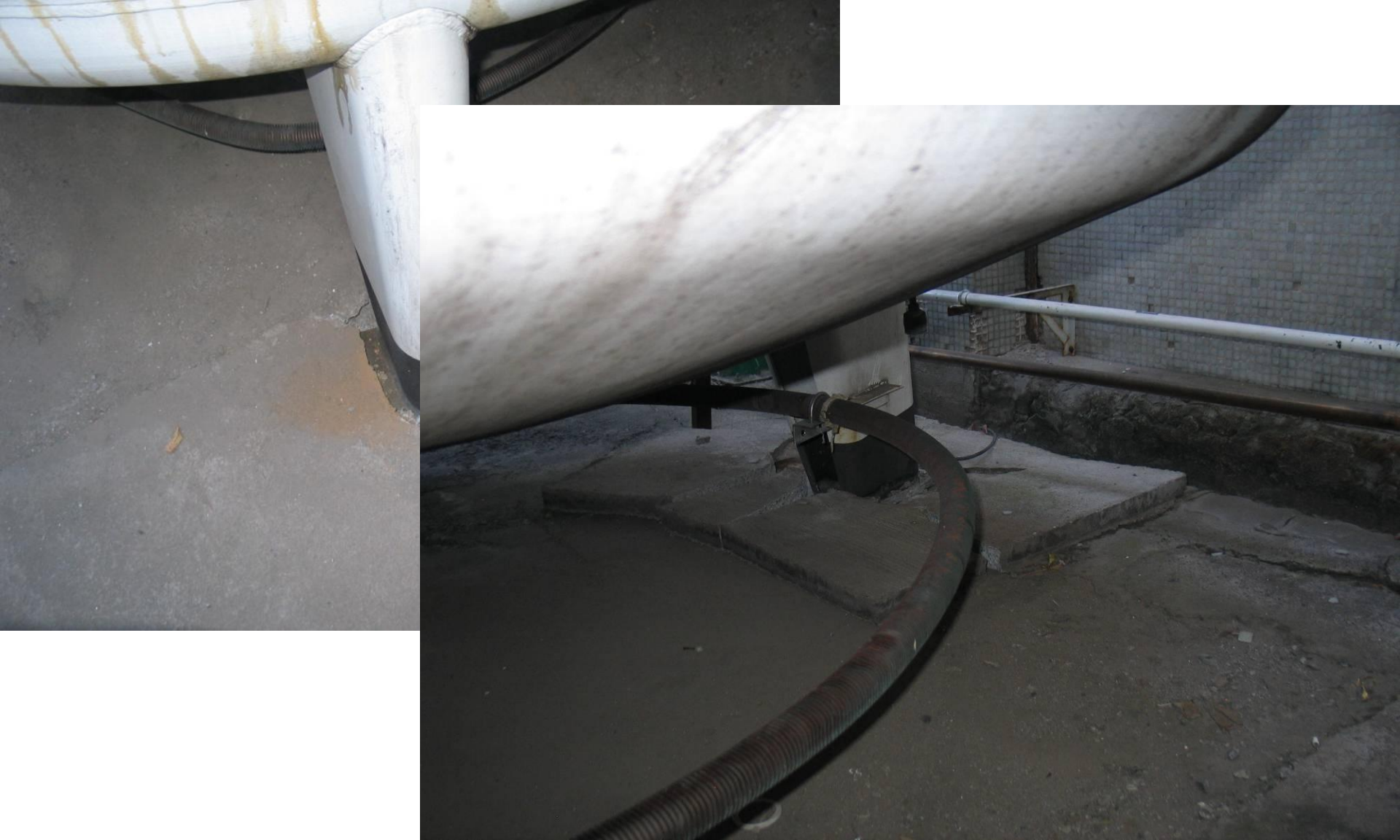
Oxygen tank legs punched through support slab but did not overturn and remained functional. Felix Bulnes-Santiago
