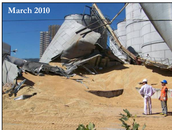
Concepción City Center: Collapsed grain bins have been removed but not yet replaced as shown in these two images taken in March and December of 2010. The 20-story residential tower in the background remains vacant. The right photograph includes the toppled Rio Alto tower (in the circle) which is still under investigation.
