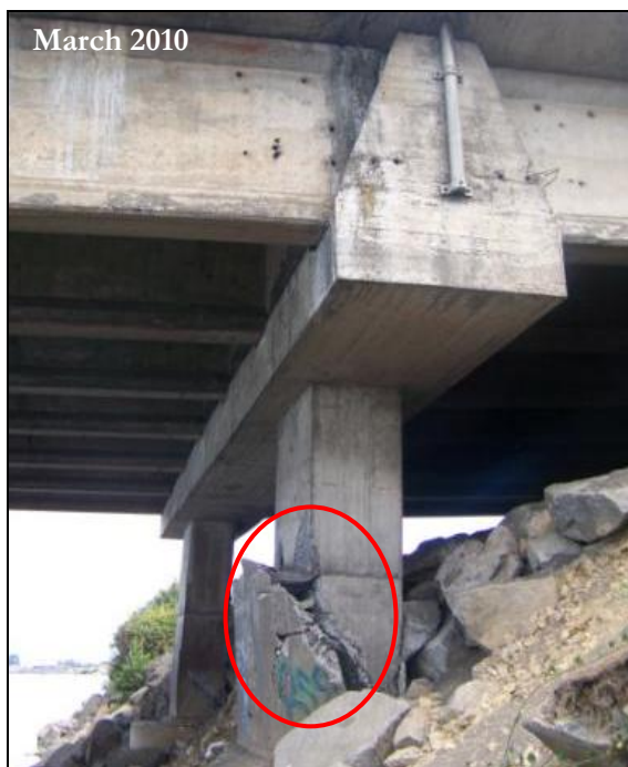
The photo on the left shows Juan Pablo II Bridge fractured column caused by soil liquefaction and lateral spreading along the Bío-Bío riverbank. The photo on the right depicts the new bridge girder and columns.
