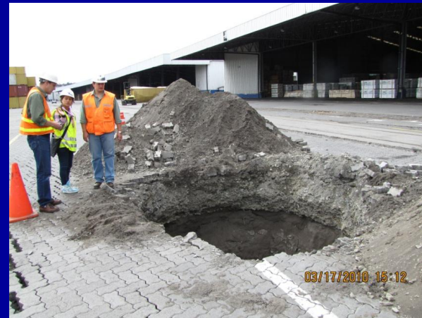
Coronel : a) Lateral Spreading/Settlement, b) Sediment Ejecta/Sinkholes, & c) Pile Damage
