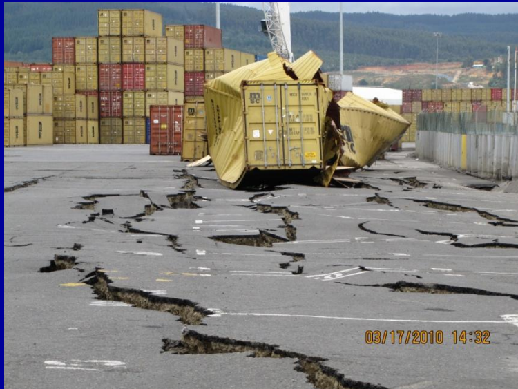
Coronel : a) Lateral Spreading/Settlement, b) Sediment Ejecta/Sinkholes, & c) Pile Damage
