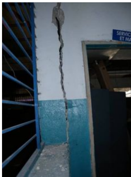
Figure 8 Part 5, single storey unreinforced masonry construction with light timber roof with metal roof sheeting.
