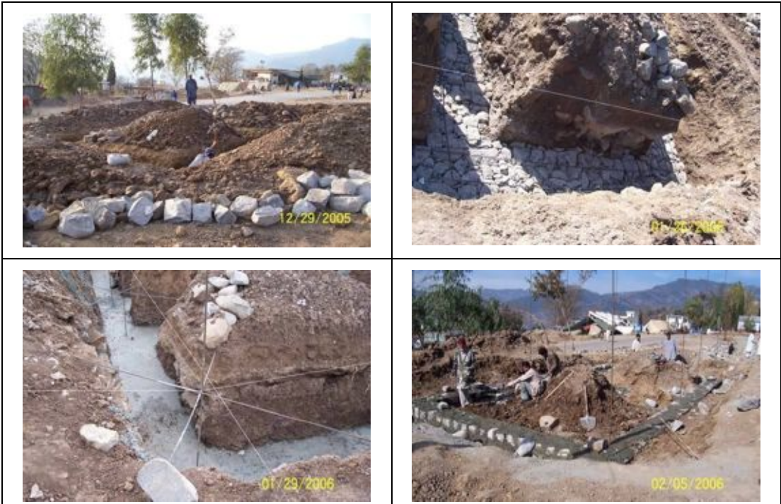
Figure 63 Preparation of foundations for a seismically resistant stone masonry house
