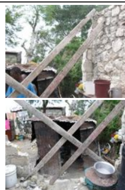
House 2 in the compound. Masonry walls failed. Two images showing the timber members resting against (and not propping) still standing stone masonry wall. (Corrugated iron structure in background still standing.)
