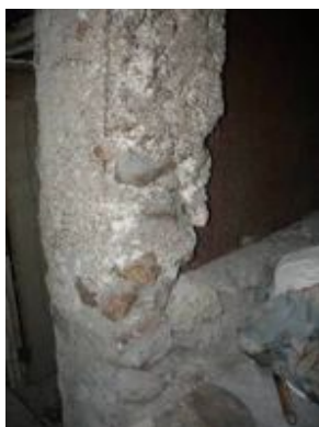
Figure 51 Example of a poorly graded concrete mix with large rocks evident in the mix.
