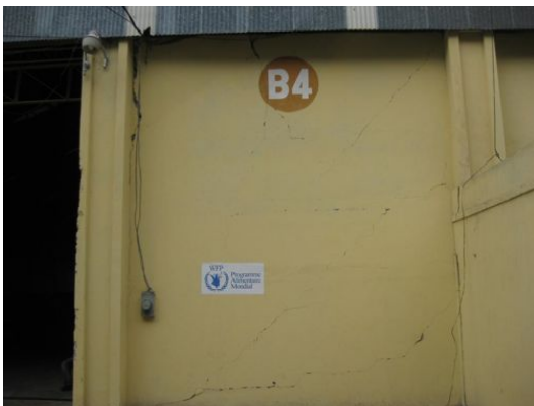
Figure 8 In plane cracking of masonry walls to the sides of the main warehouse loading entrance.
