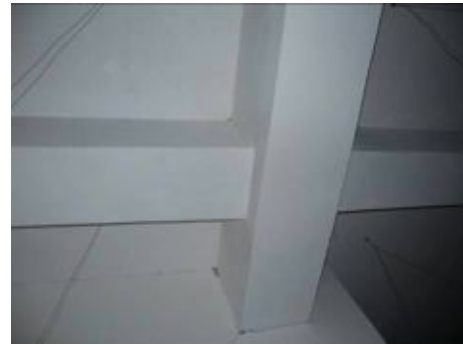
Figure 7 Part 4, single storey reinforced concrete frame with unreinforced masonry infill.
