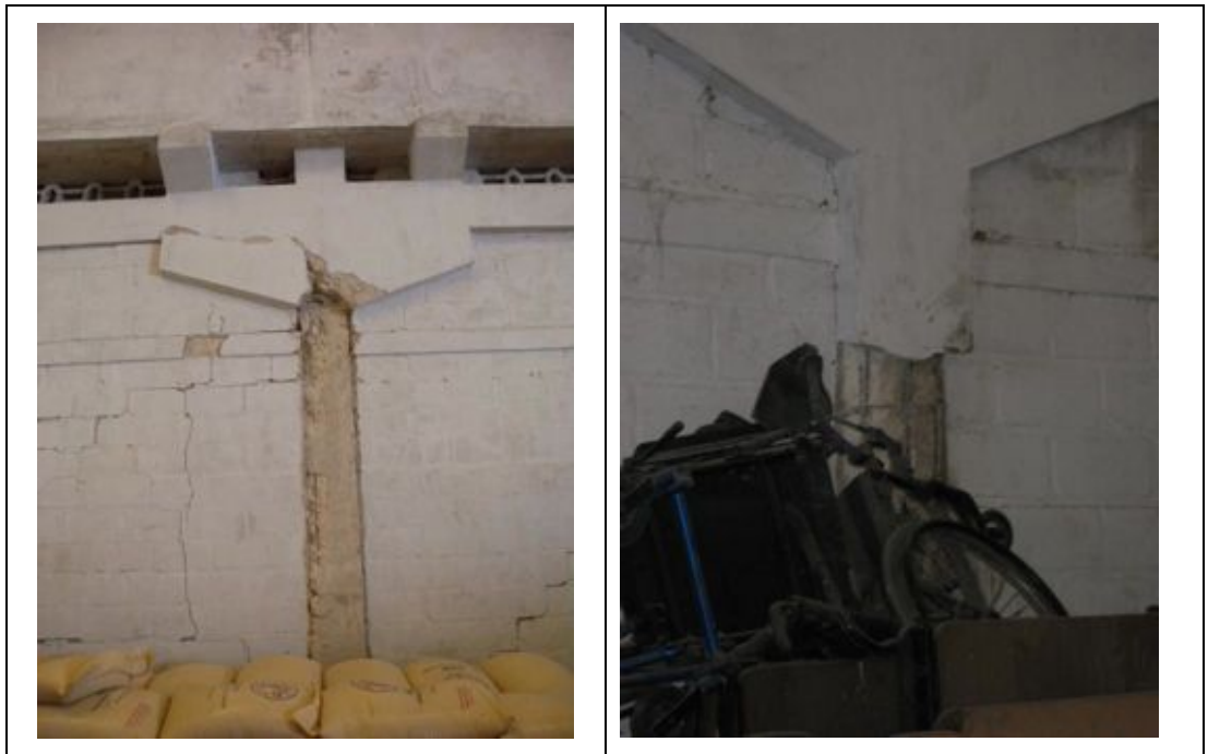
Figure 14 Damage to concrete columns appears to be limited to the cover. Damage to column head / around interface to gutter beam is apparent too.
