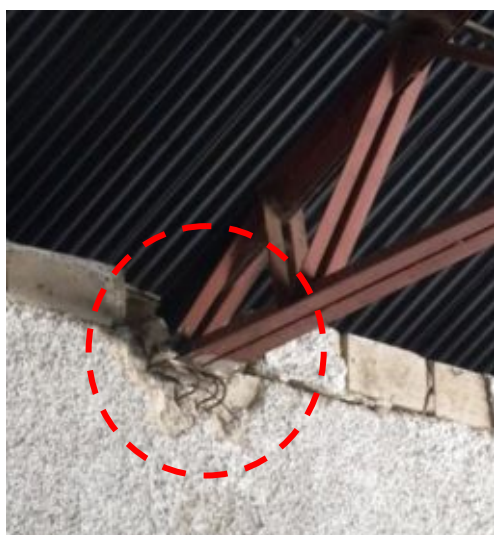
Figure 10 Steel to concrete connection
