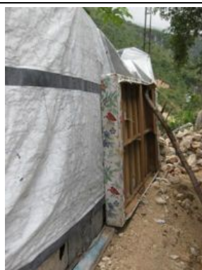
House 2 in the compound. Masonry walls which had been constructed collapsed. Temporary "walls" installed.
