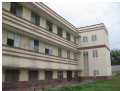
Rear view of Main Building #1 (3 storey). Stairwell (on right) added after construction of original building. Some minor cracking at junction between two constructions.
