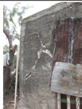
House 1 in the compound. View of South east of the house showing severe cracking in the masonry infill panel
