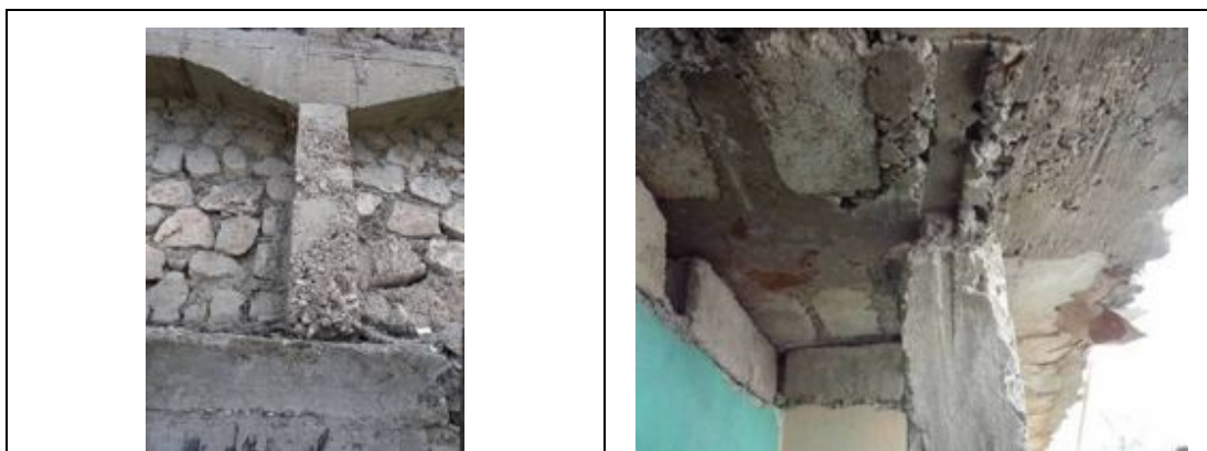
Figure 57 Example of poorly graded and poorly compacted concrete
