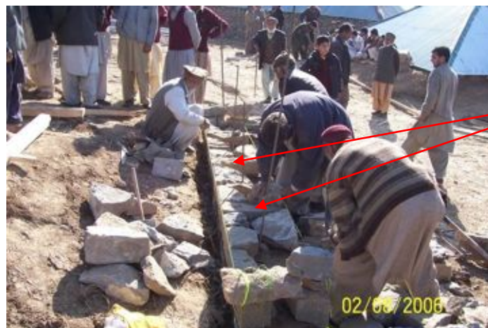
Figure 66 Through Stones and Vertical Reinforcement.
