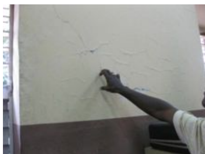
Cracking in plaster of thick masonry wall. Seen typically at the ground floor levels for all Main Buildings.
