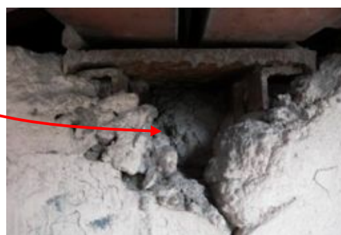
Figure 9 Gutter beam details and typical roof truss to concrete connection (taken from either warehouse B2 or B3 due to easier access at those locations).
