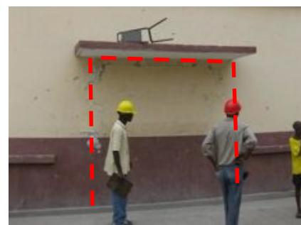
Cracking at junction between infill masonry pannel (apparently installed after original construction) and original structure. (possible original opening highlighted by red dotted line.)
