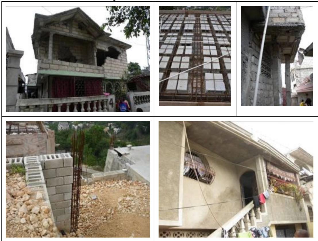
Figure 5 C4-HBFS-UHM, Concrete frame with hollow block flat slabs with un-reinforced hollow block masonry infill
