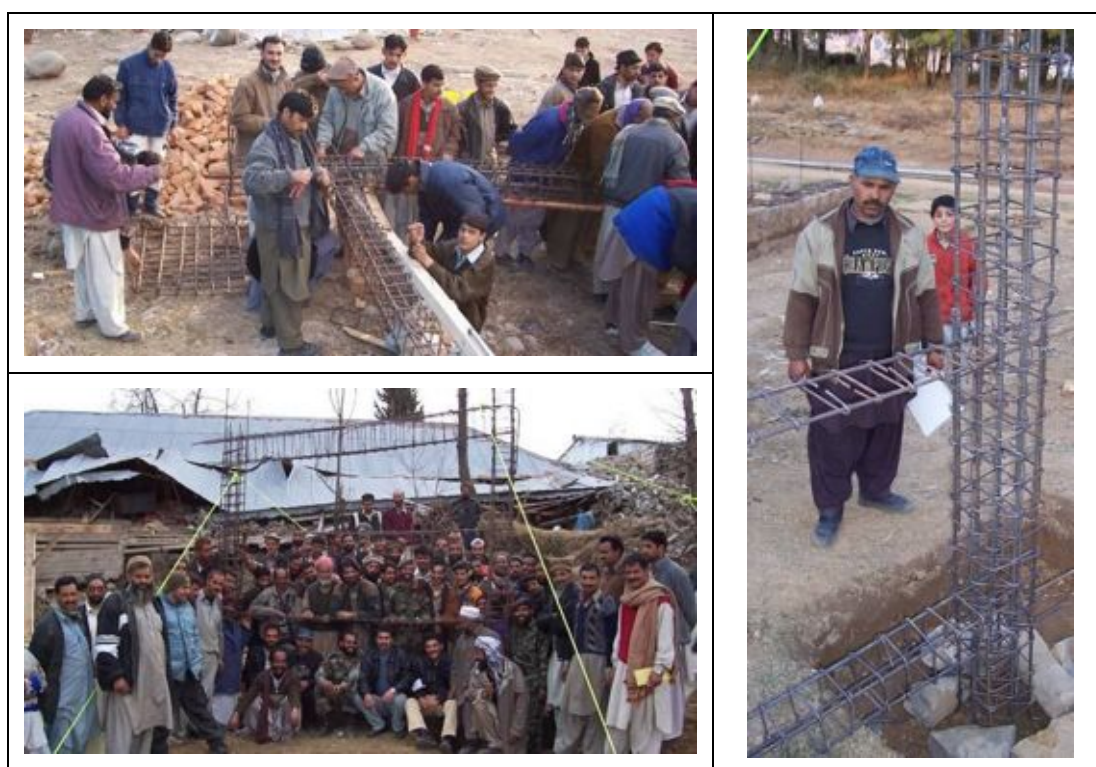
Figure 24 Practicing seismic detailing of reinforcement
