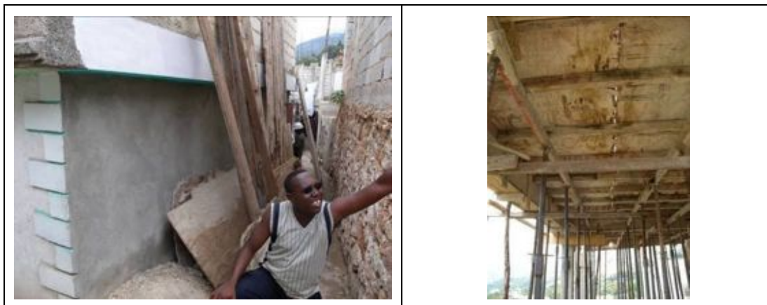
Figure 56 modular formwork system, that is constantly recycled
