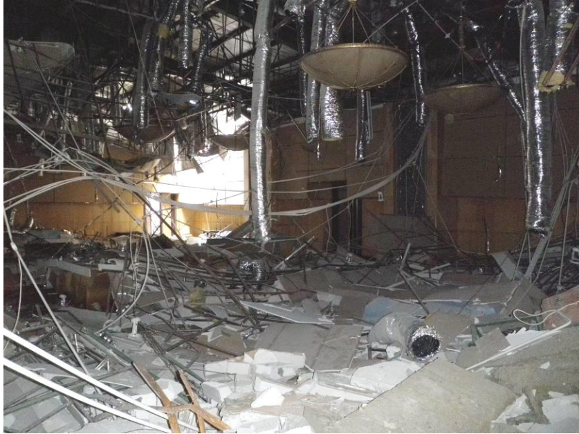
Figure 2: Second-Floor Ballroom in the Hotel with Collapsed Ceiling
