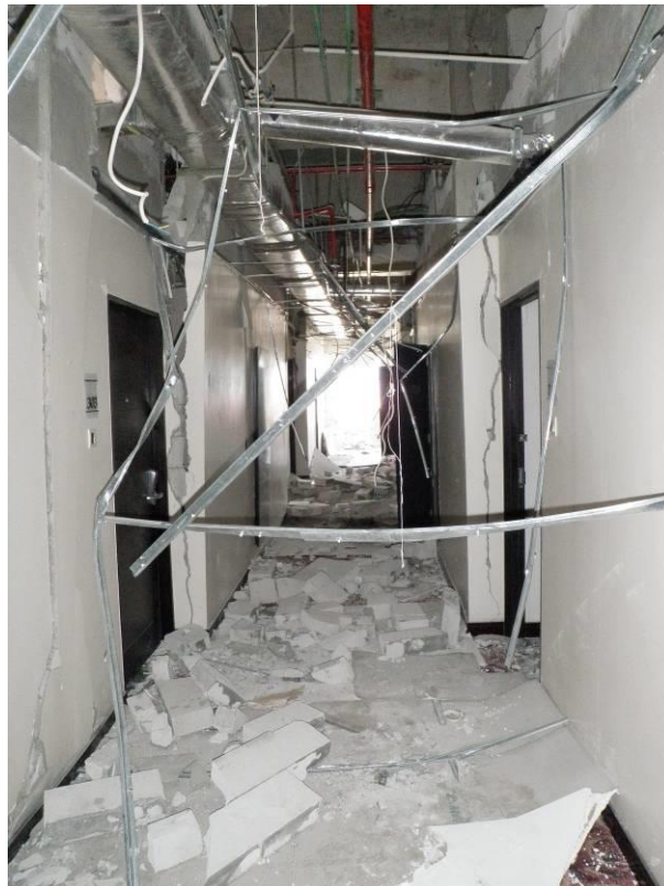
Figure 3: Fourth-Floor Hotel Corridor Showing Major Non-Structural Component Damage
